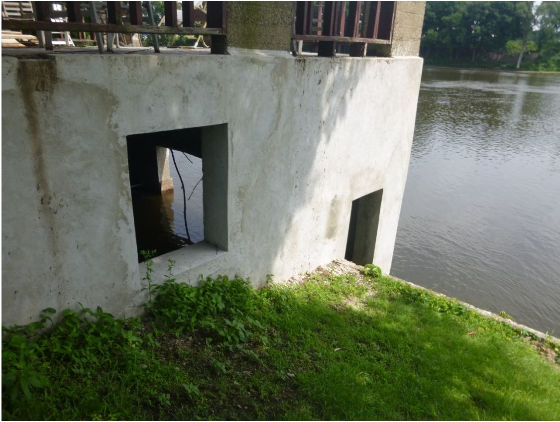
Figure 5 -- Boat house lower level, looking north.
