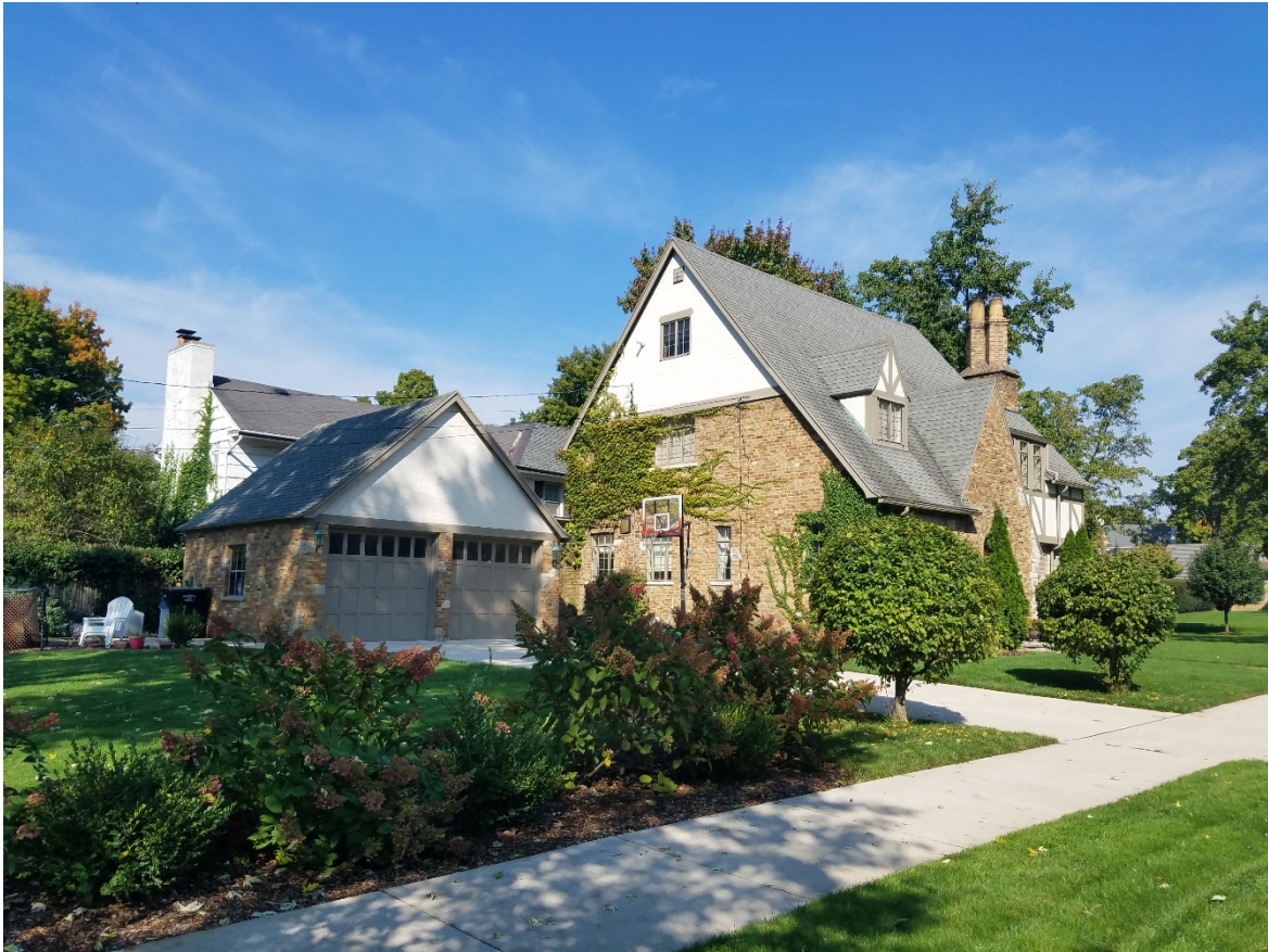
Figure 2 - 301 Sunnyside, showing the garage and the area for the new construction.
