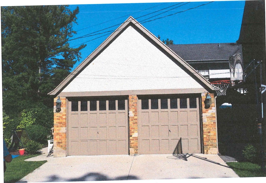
Existing Garage, East Elevation
