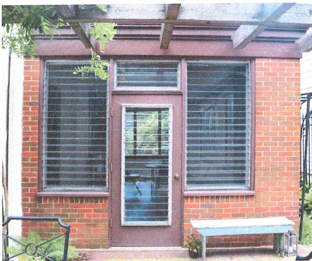
Existing North Elevation at Three-Season Porch
