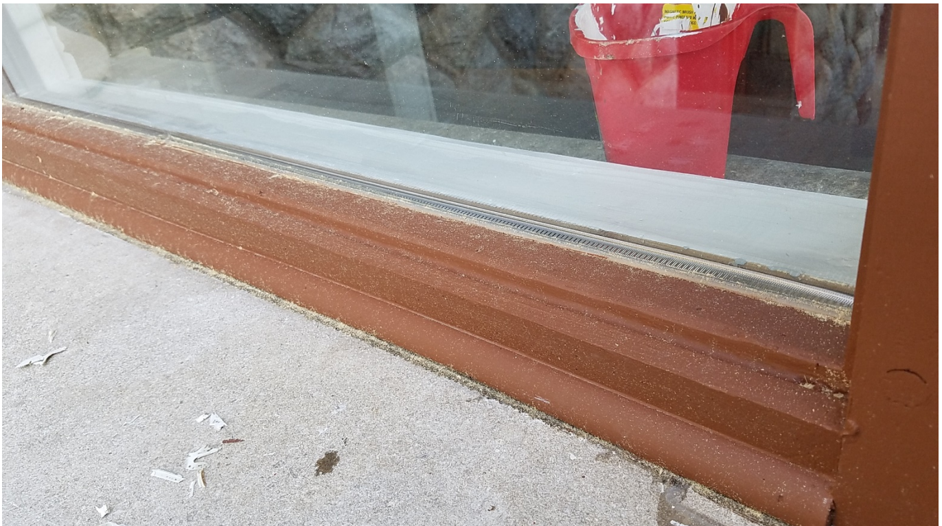
Figure 3 - Detail of replacement windows on enclosed porch.
