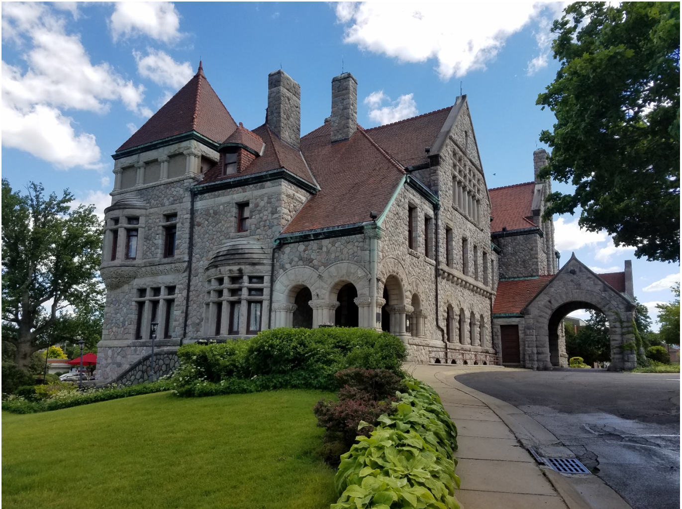
Figure 1 - 620 W Washington, from the driveway.
