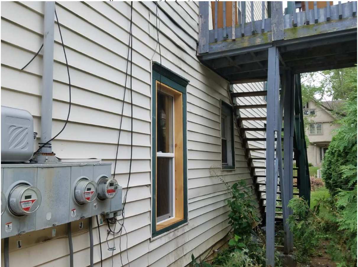
Figure 5 -- Subject property, looking southeast.
