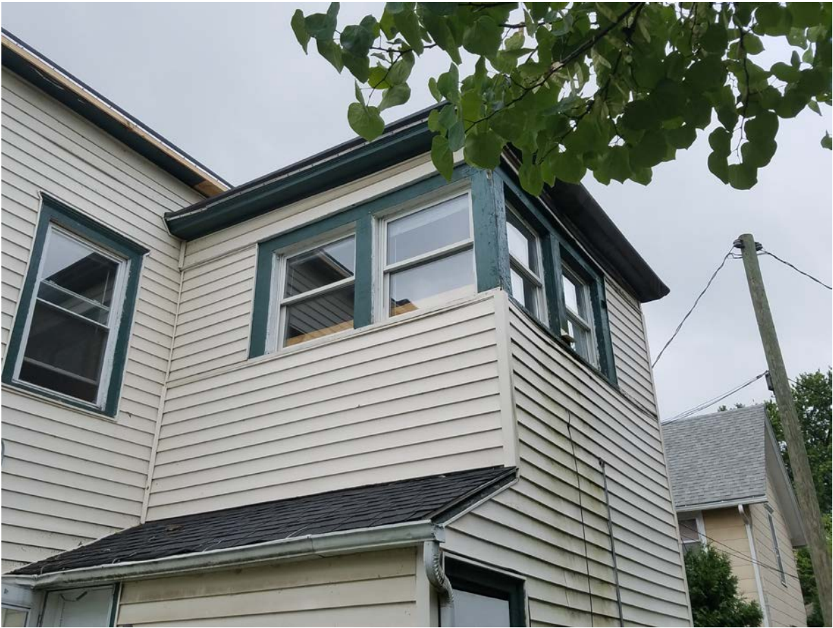
Figure 4 -- Rear of property, looking south east.
