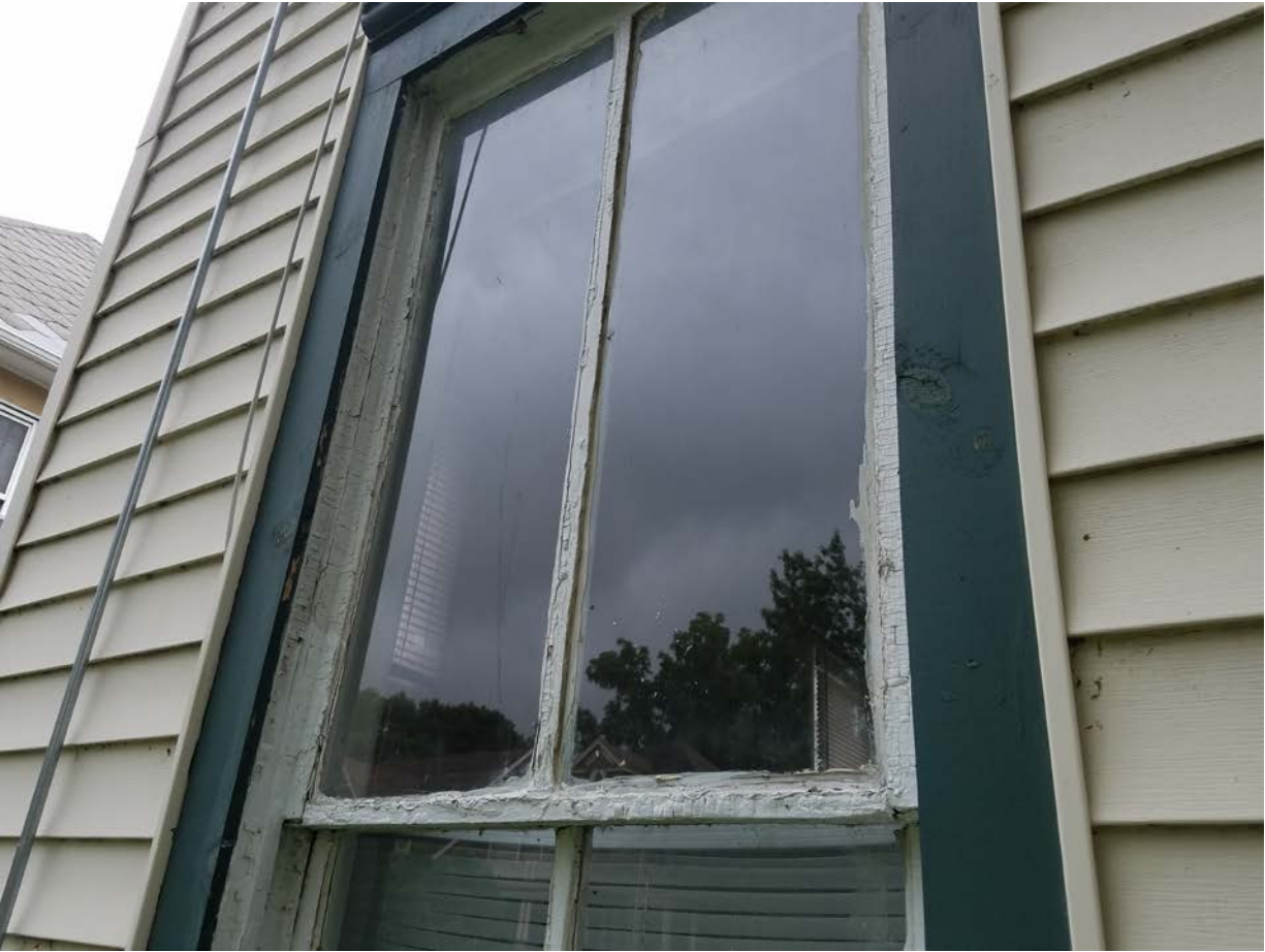
Figure 8 - Original window, south side of the subject property.
