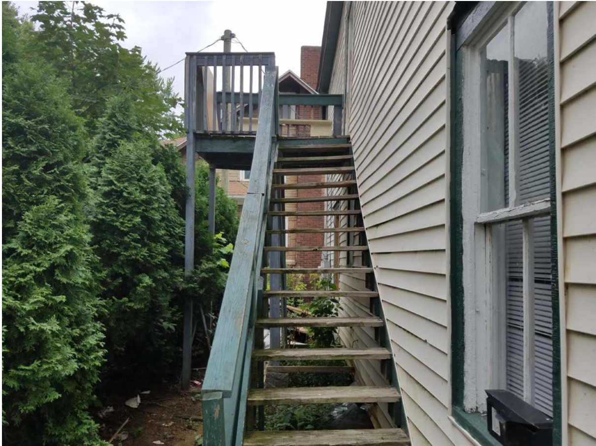
Figure 6 - Subject property, looking north. Original window at edge of frame.
