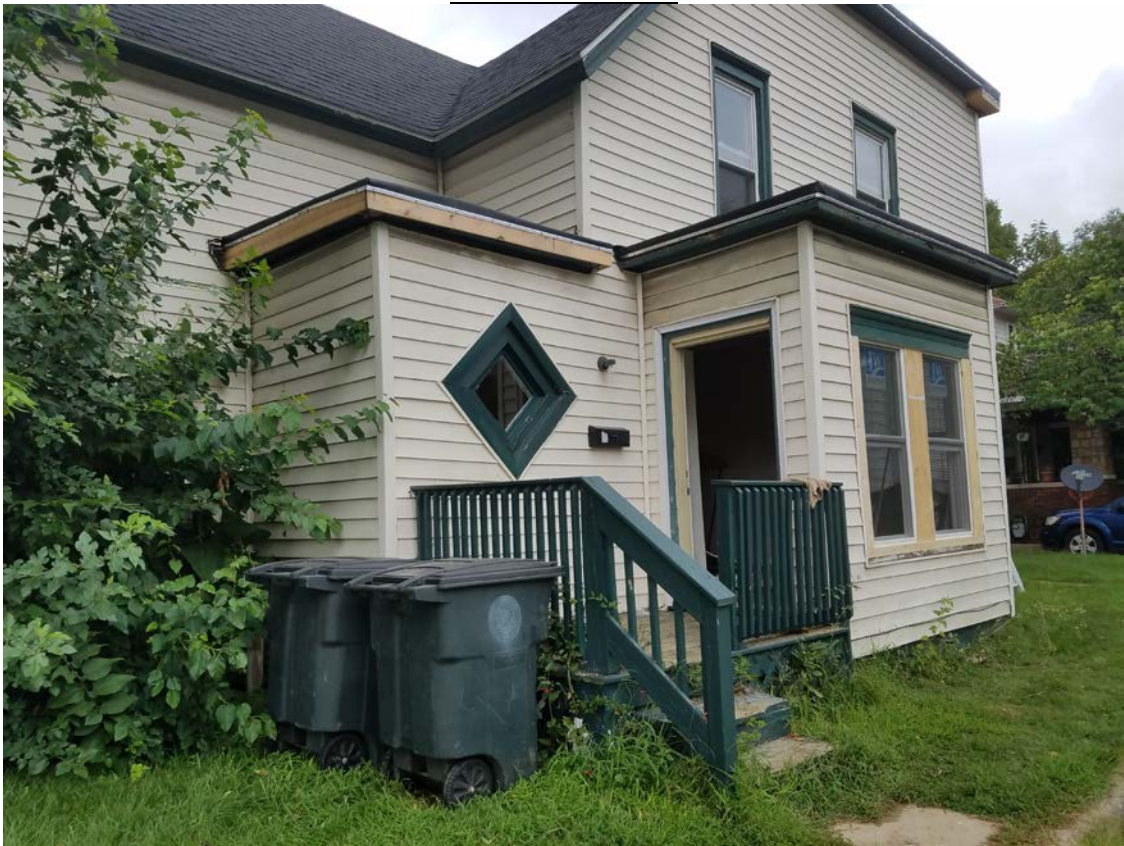
Figure 2 – 601 Lafayette Boulevard from the sidewalk, looking north west. Window replacement on entry addition is visible at right.
