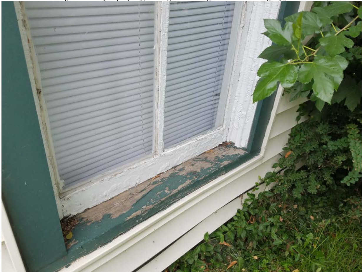
Figure 7 - Original window/sill on the south face of the subject property.
