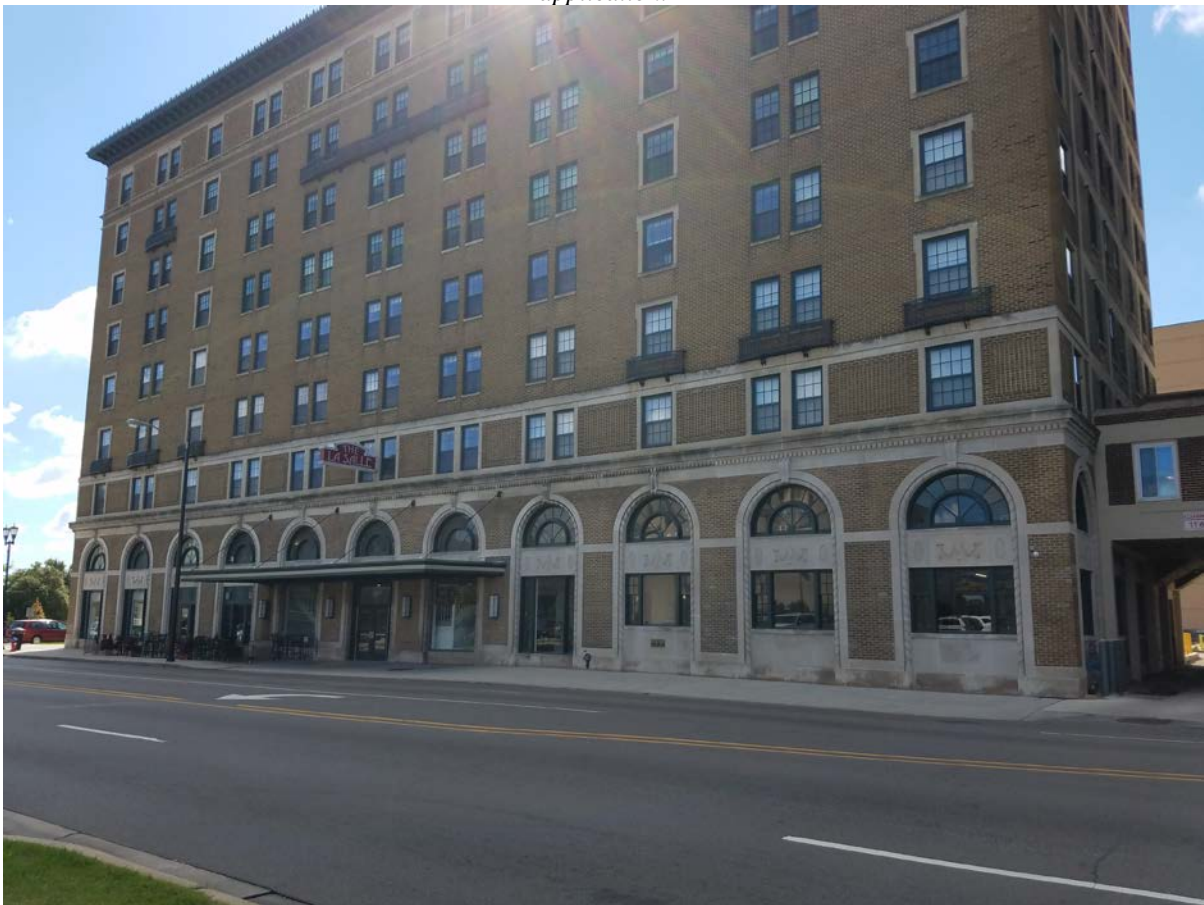
Figure 4 - The LaSalle Building, looking southeast.
