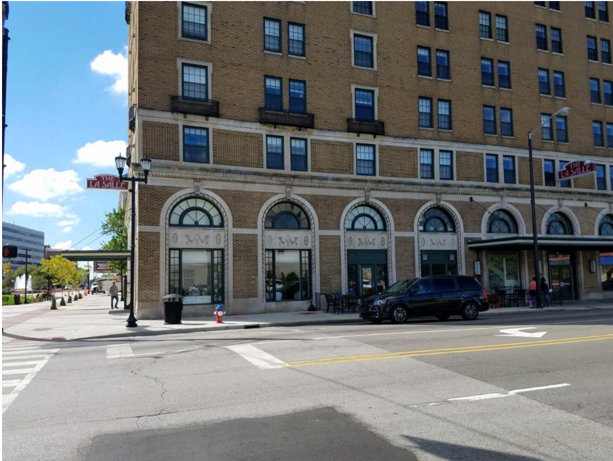
Figure 3 - The LaSalle Building, looking south. The two ground-floor windows closest to the corner are also part of this application.
