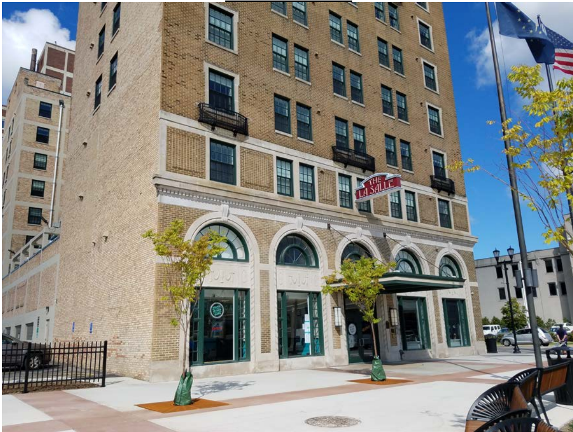
Figure 1 – 237 N Michigan from the street, looking northwest. Two of the subject windows are at the right.
