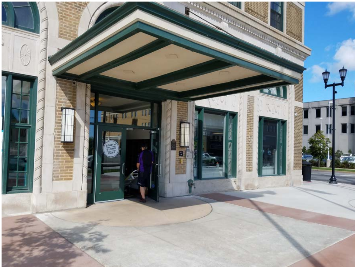
Figure 2 - The east entrance to the Lasalle Building. Two of the subject windows, at right. Note "South Blend Cafe" signage on door.
