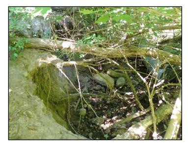
Photo 4-4 View of Erosion near 24" Diameter CMP Pipe
