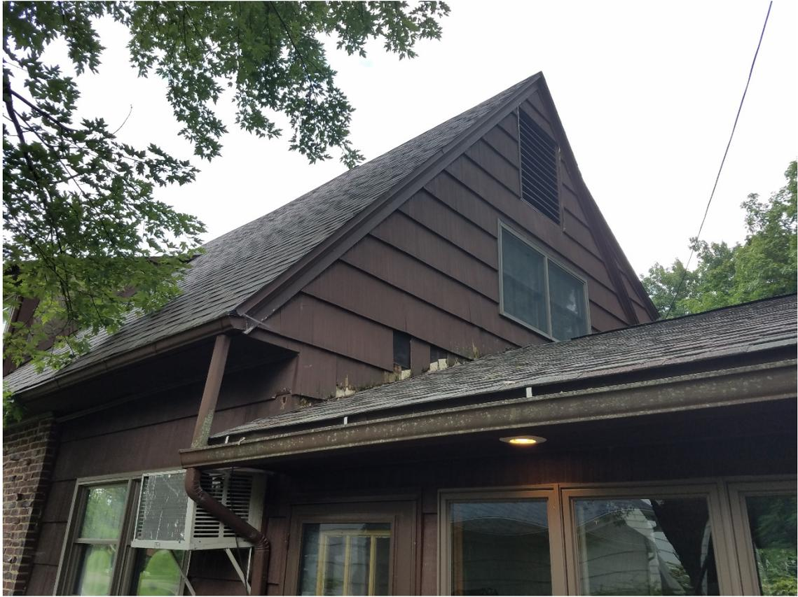
*Figure 6 - The later addition, looking to the west. The shed dormer is visible at the left edge of the image. Note Cedar siding deterioration.*
