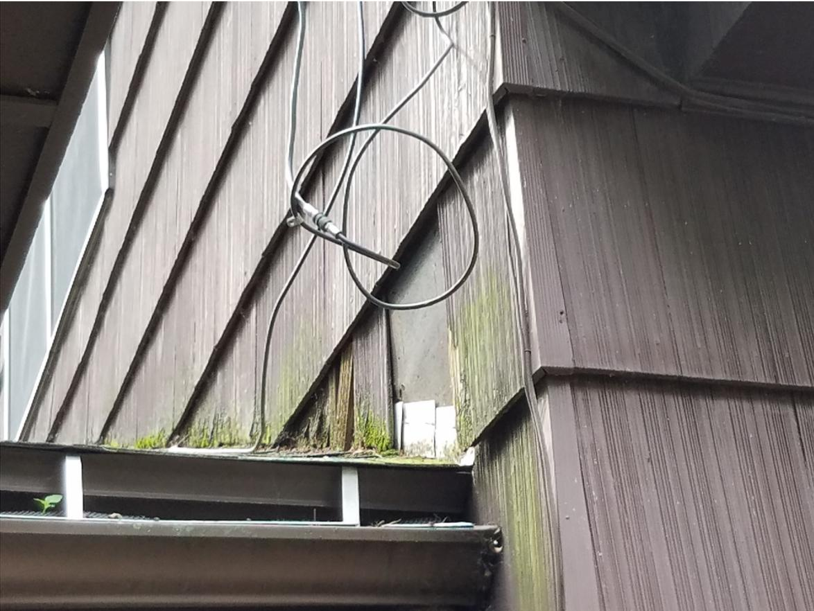
*Figure 11 - Shingle deterioration at rear of home on addition.*
