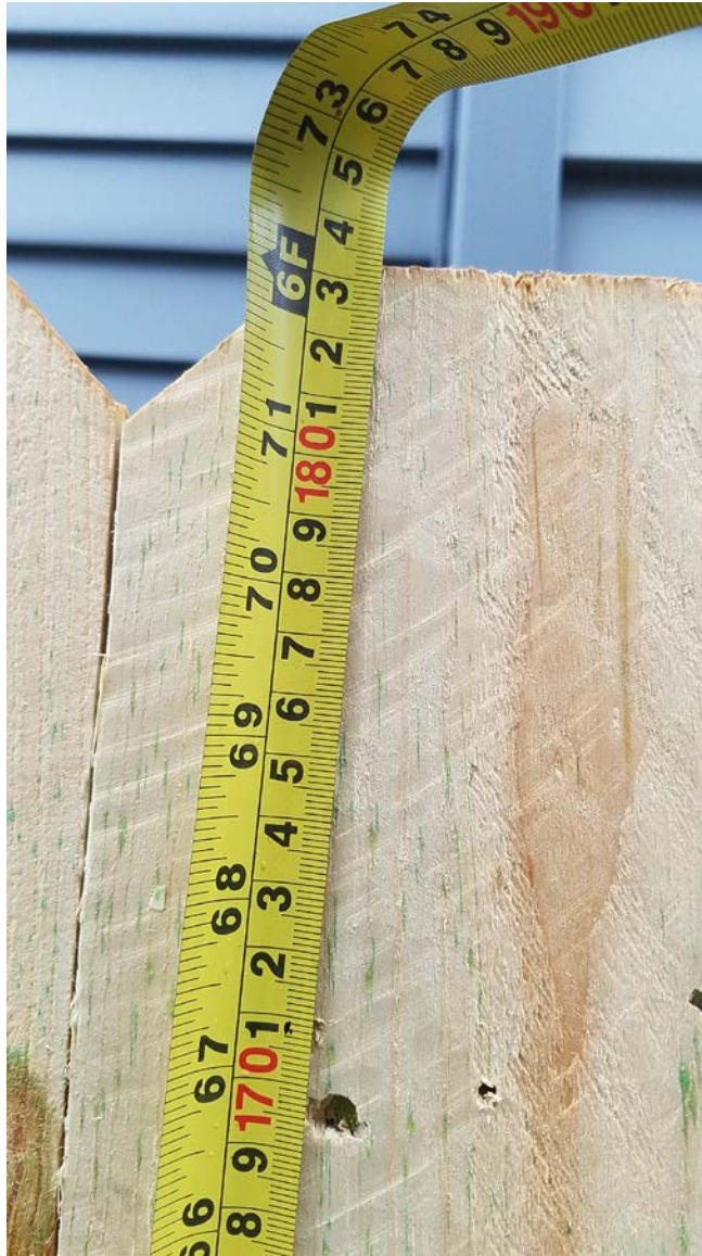
Figure 6 - Showing the height (6') of the fence.
