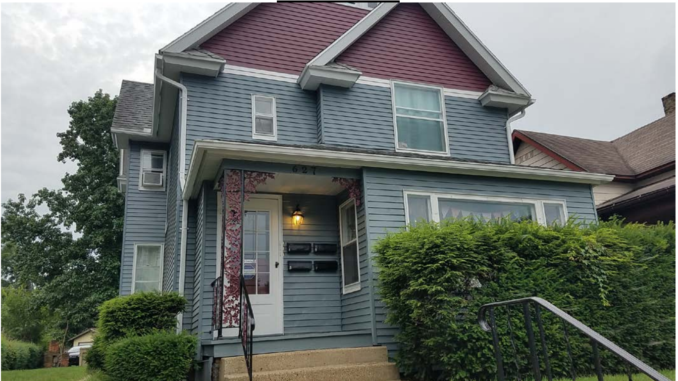
Figure 1 – 627 Portage from the street, looking west. The fence is to the right, on the other side of the hedge.
