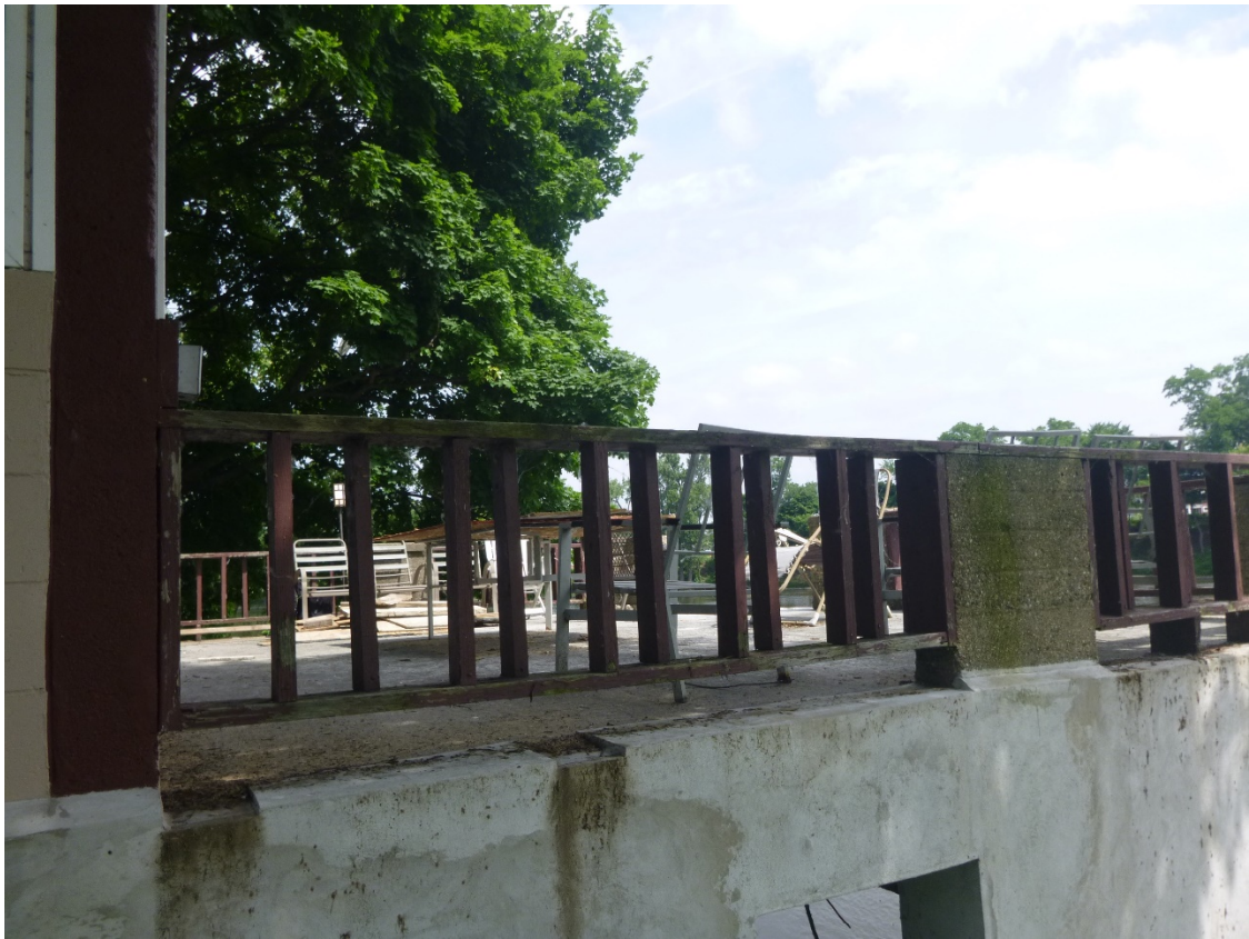
Figure 4 -- Boat house railing, looking north.
