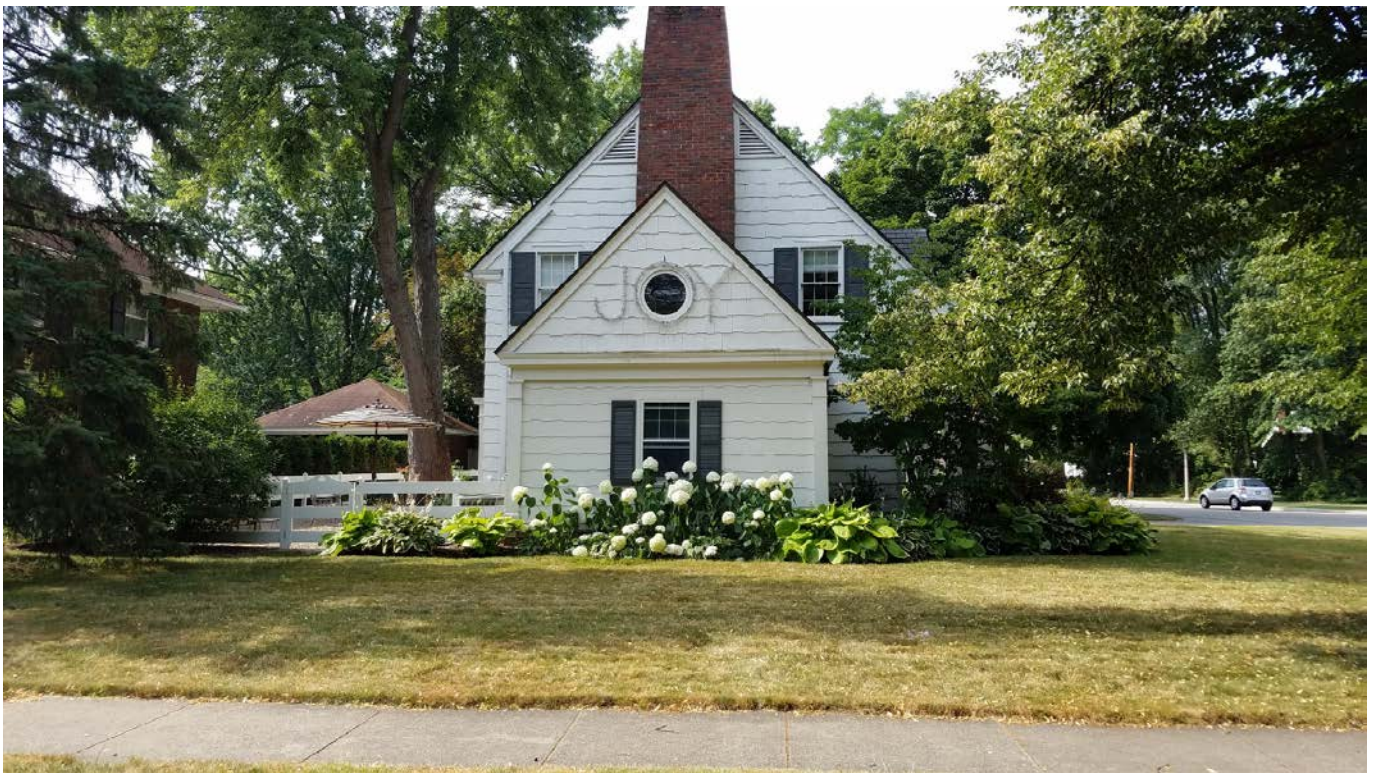
Figure 2 - 304 Twyckenham, north elevation.
