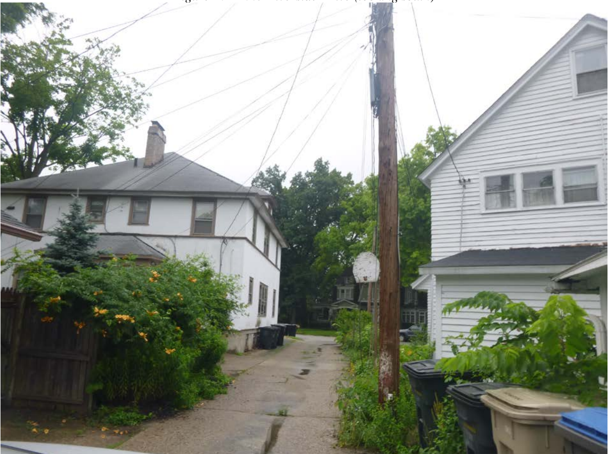
Figure 11 - Utility alley, looking north. Proposed TESCO box installation would be in this vicinity.
