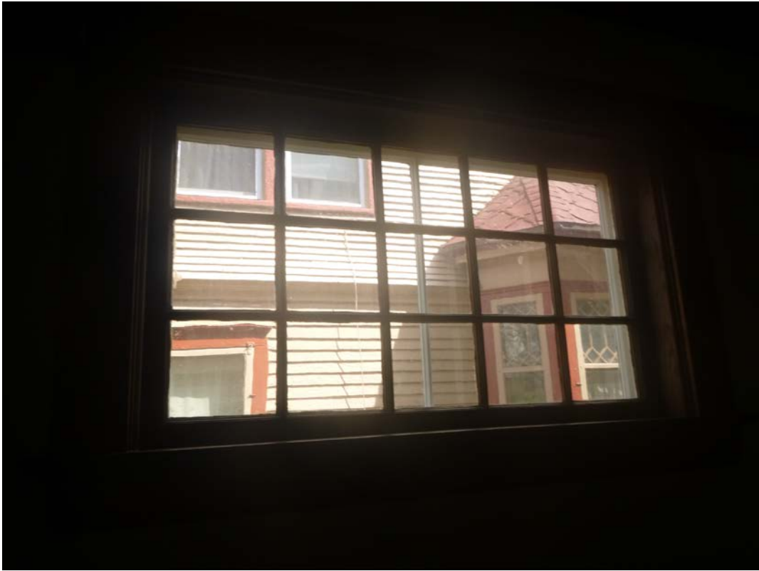
Figure 11 - 608 Park – north facing casement window.
