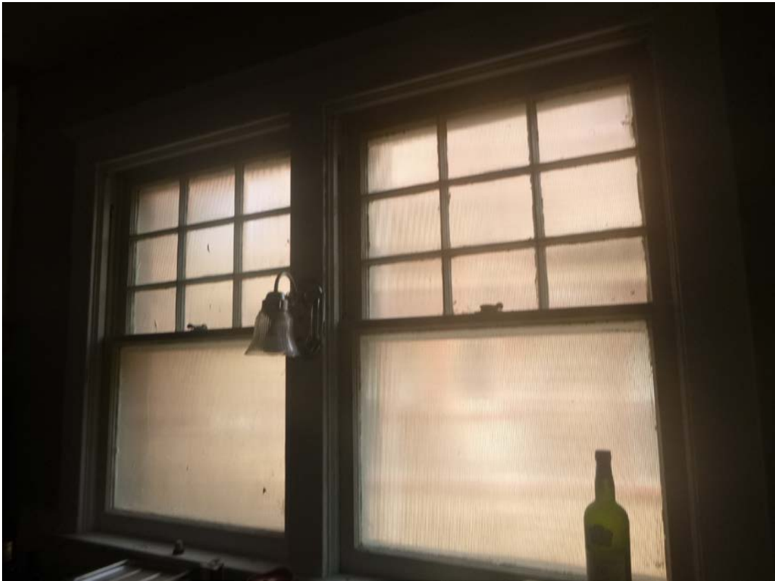
Figure 10 - 608 Park - existing / original 9/1 windows.
