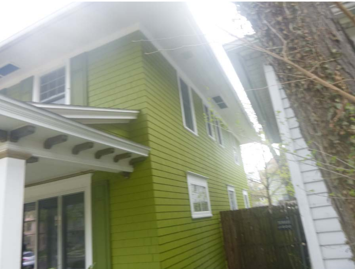
Figure 4 - 608 Park, south face.
