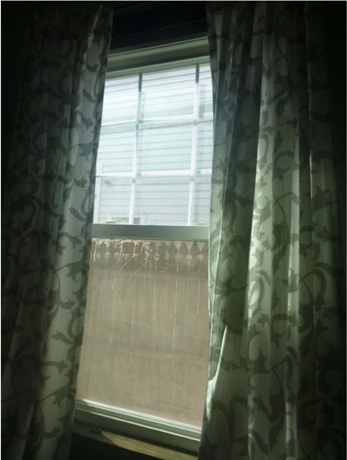
Figure 5 - 608 Park -- existing vinyl replacement window.
