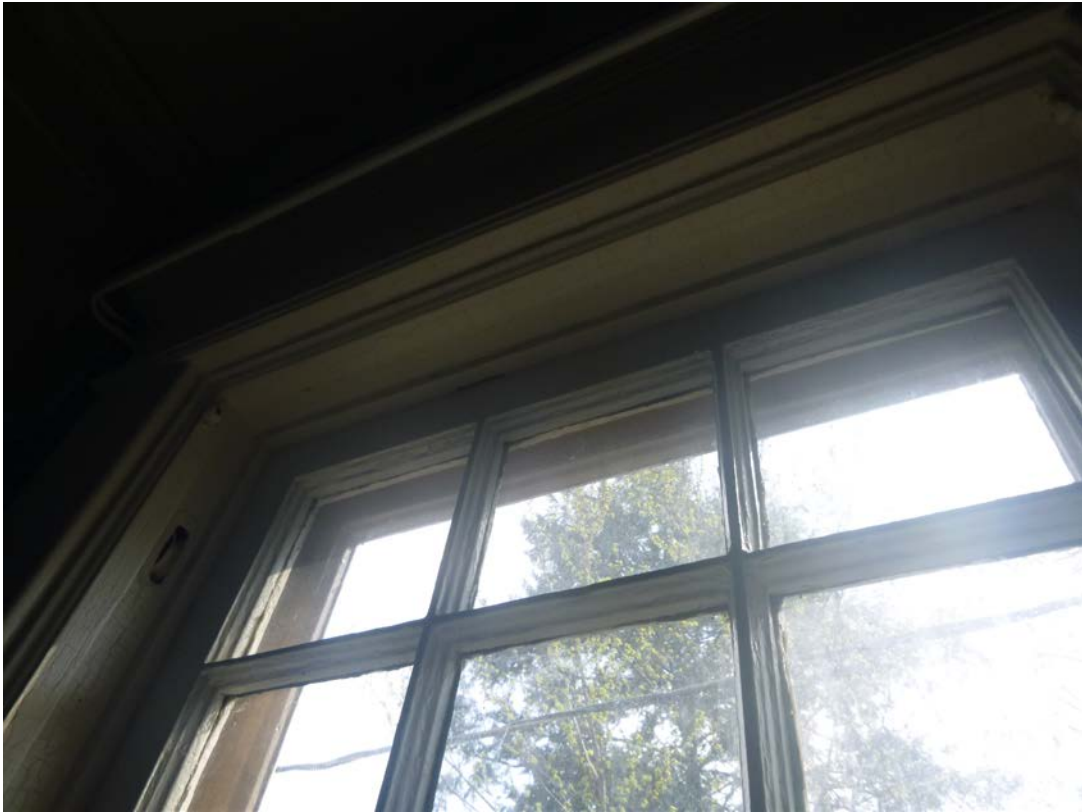
Figure 9 - 608 Park - close-up of existing / original 9/1 window.
