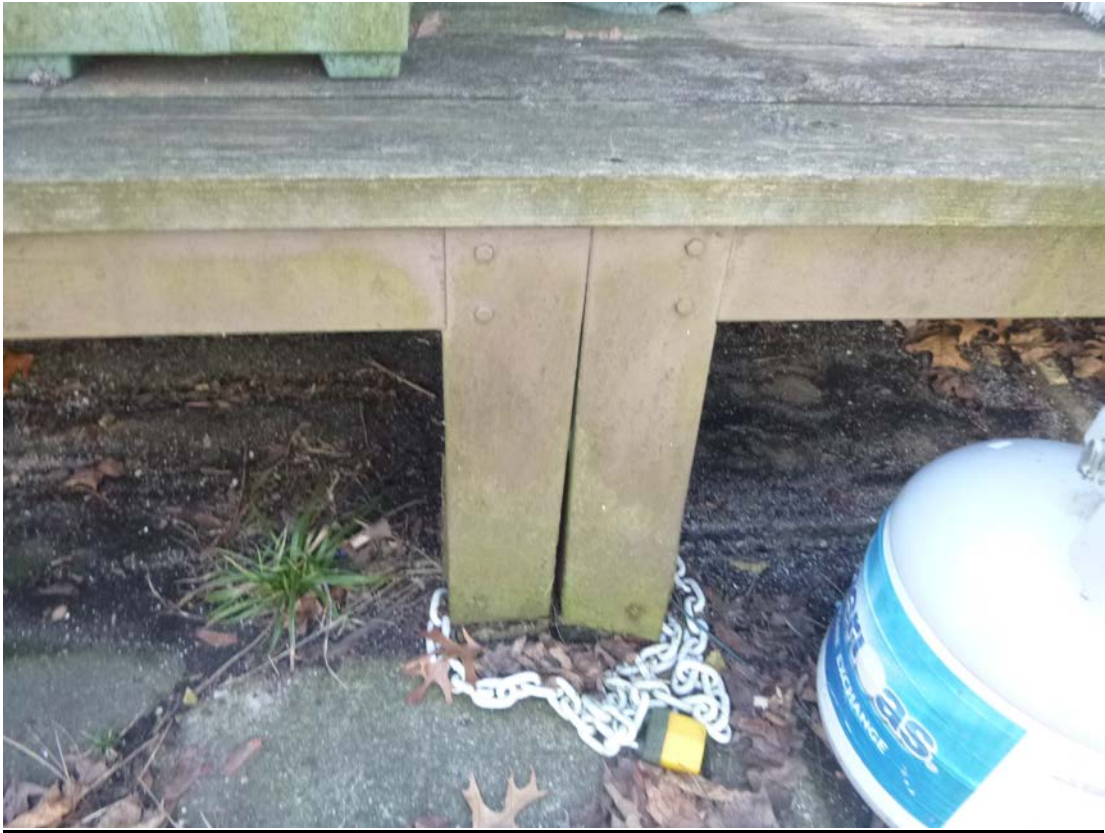
Figure 7 - 802 Forest, existing porch posts.
