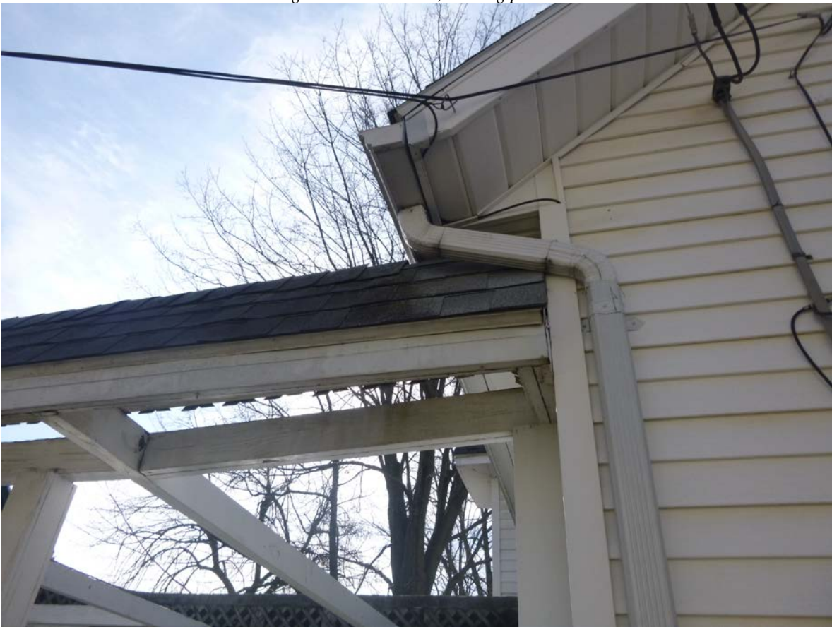
Figure 4 - 802 Forest, existing porch and pergola.
