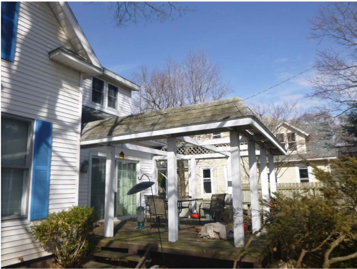
Figure 2 - 802 Forest, existing porch.
