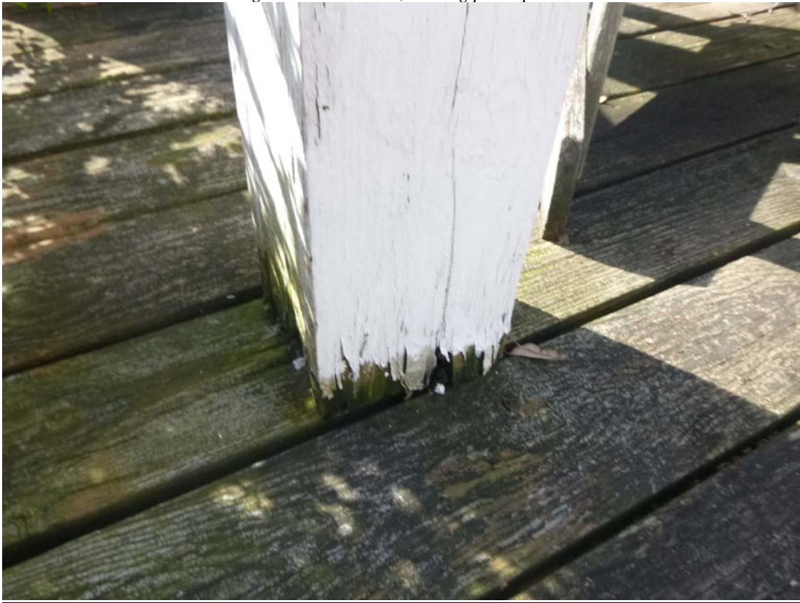
Figure 8 - 802 Forest, porch posts.
