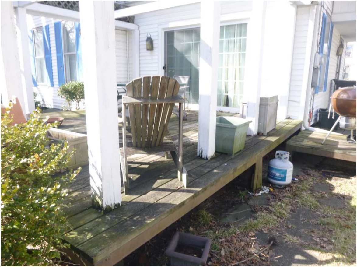
Figure 3 - 802 Forest, existing porch.
