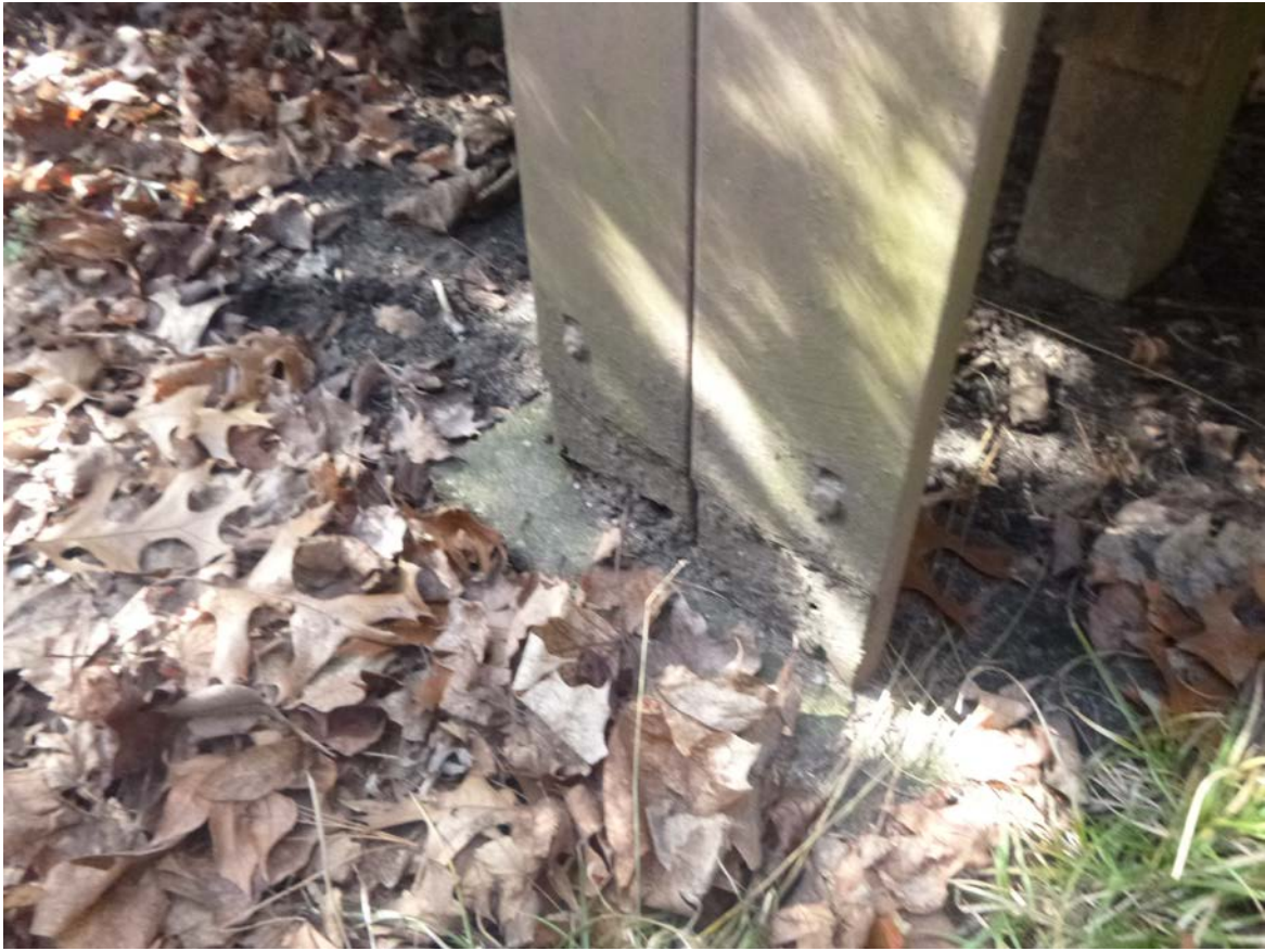
Figure 5 - 802 Forest, porch foundation post.
