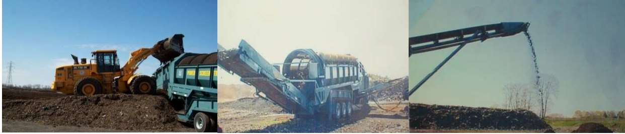
Screen machine being loaded
