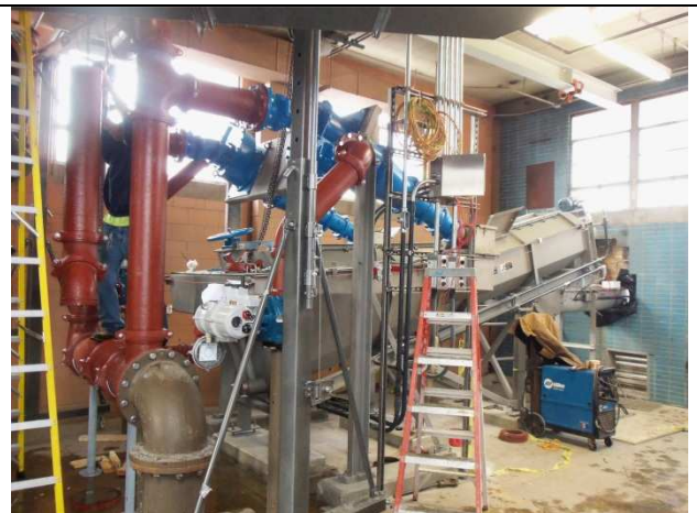
New WEMCO Hydrogritter Separator Unit, JDV Conveyor Unit, and Rotork Actuated Valves
