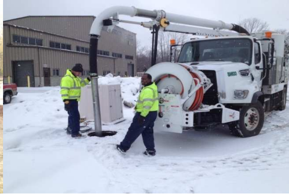
WWTP DRAIN & LIFT STATION CLEANING
