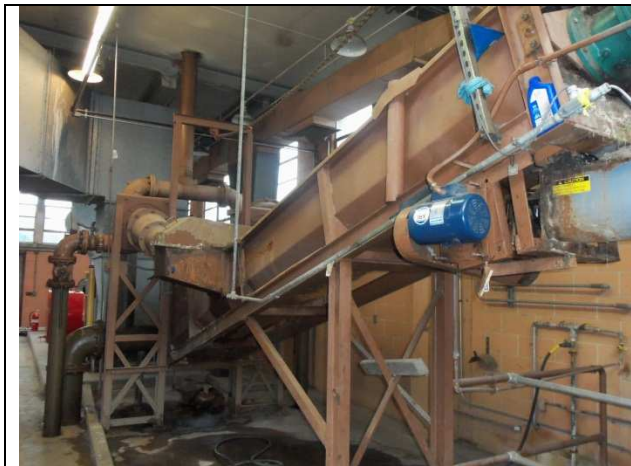
Old WEMCO Hydrogritter Separator Unit, conveyor, and manually actuated valves
