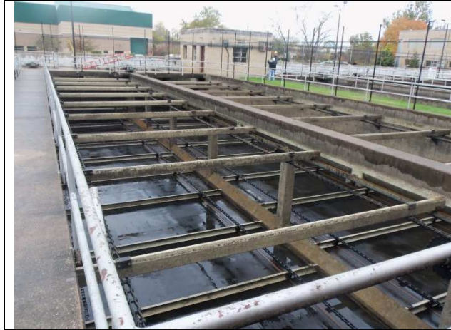
Demolition of Air Pipe from Primary Tunnel
