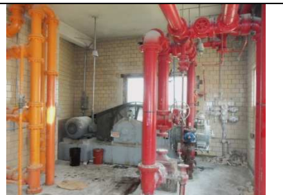
Digester 2 Control Building before demolition
