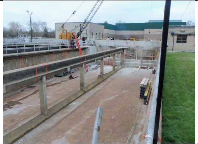
Installation of New Electrical Conduit in Tunnel
