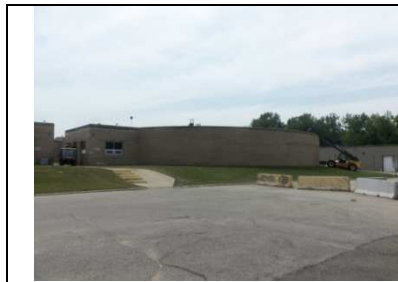
Digester 2 façade prior to demolition
