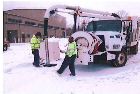
WWTP DRAIN & LIFT STATION CLEANING
