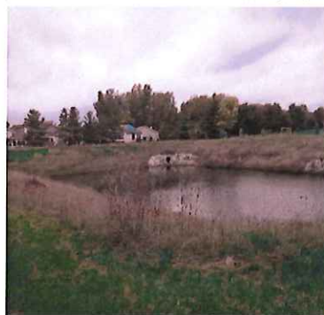
FAIRFAX BASIN (PRIOR TO CONSTRUCTION)
