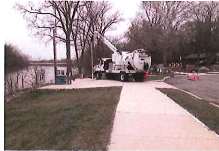
27 TH STREET LIFT STATION WET WELL CLEANING
