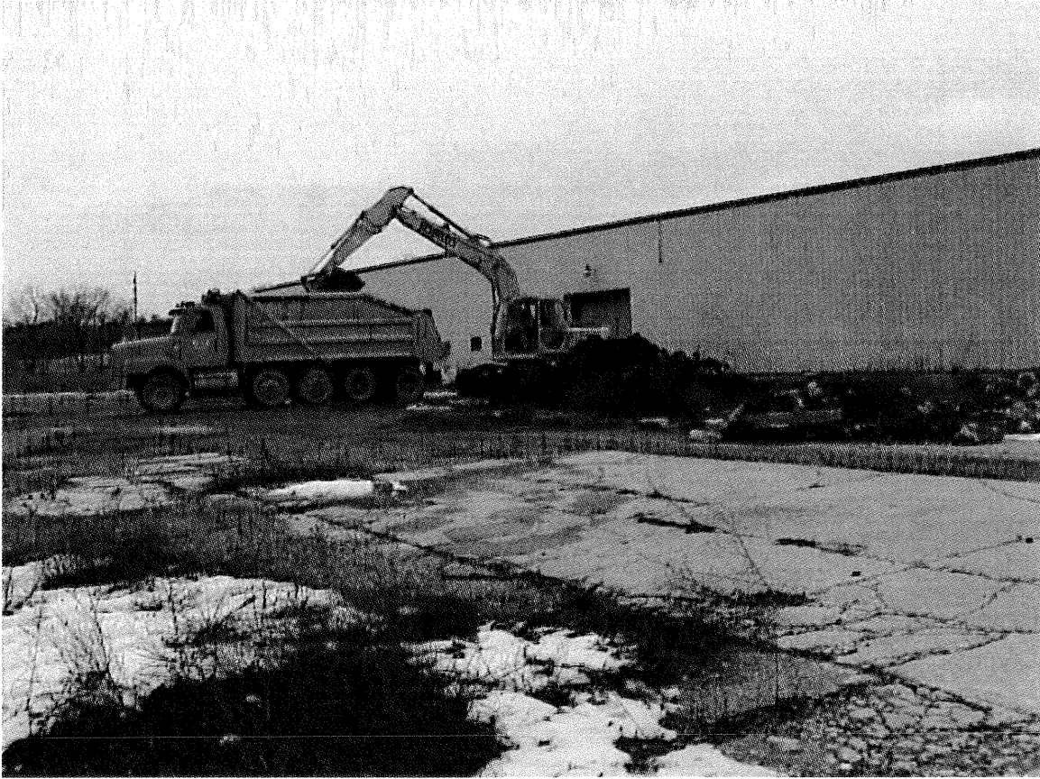
Loading the impacted soil for transport to Prairie View RDF.
