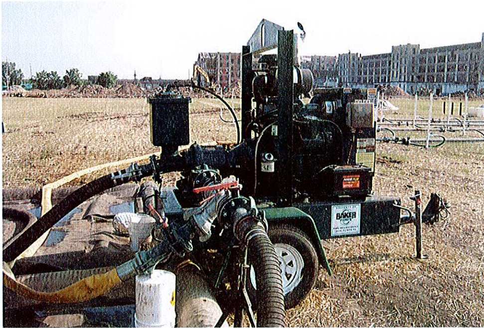
No. 3 – Diesel pump (900 gpm) used for mixing and injecting the permanganate solution.
