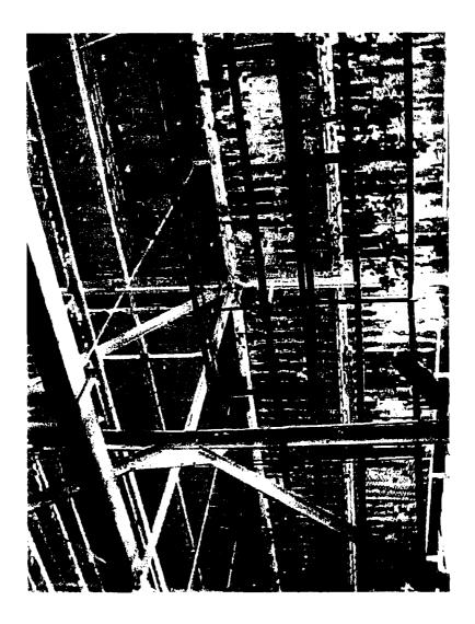
Photo #8: Typical condition of approximately 60% of the ceiling paint located inside Building 103. Ceiling paint is considered to be lead-based.
