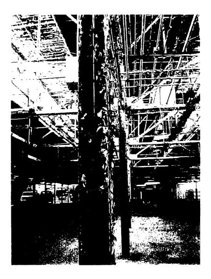
Photo #7: Typical condition of paint on approximately 50% of the columns inside Building 103. Paint is considered to be lead-based.
