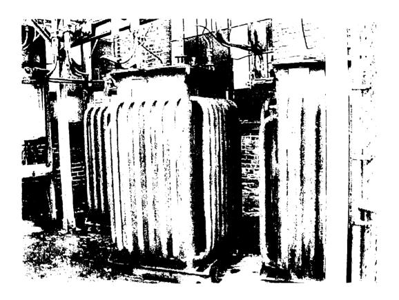
Photo #3: Close-up of three of the transformers within the fenced area outside the southwest side of Building 103 (near Building 104). Condition of transformers and concrete pad is typical of the area.
