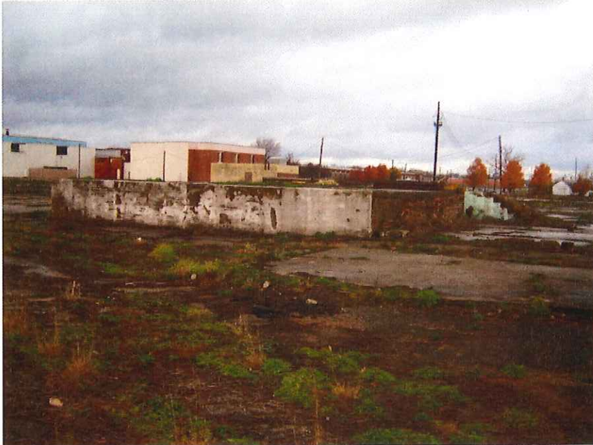
Remnants of possible elevated dock platform associated with demolished building.
