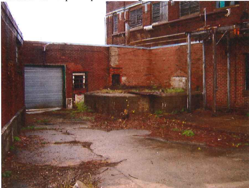
Enclosed area of power plant building where transformers were located.
