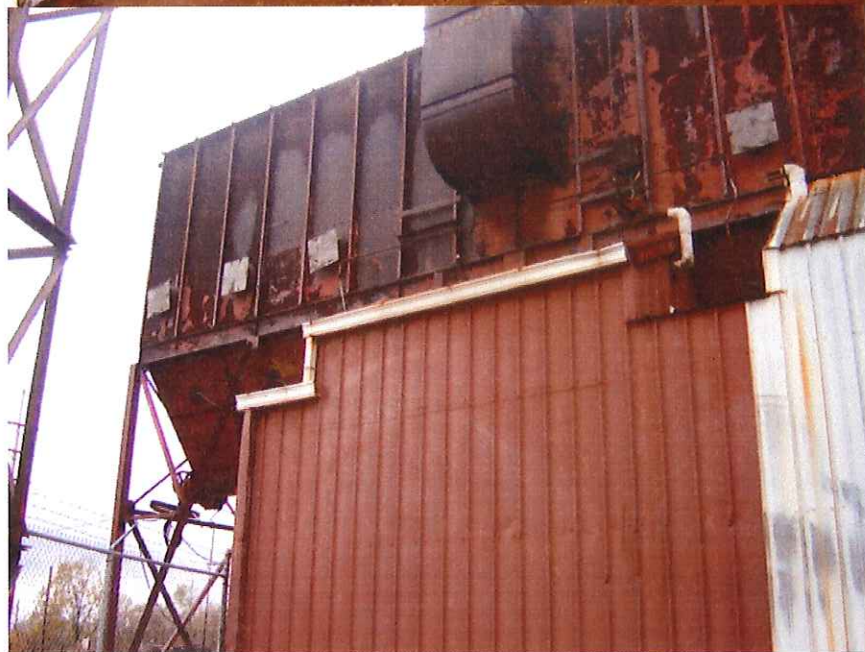
Baghouse area? located to the east of power plant building
