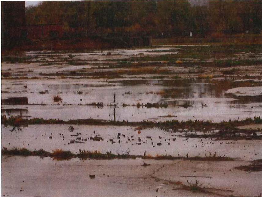
Former building floor slab that covers most of the Property.
