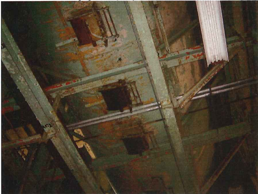
Overhead coal chutes.
