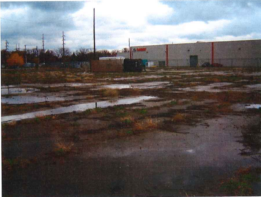
Property looking northeast. Enclosed area houses a groundwater recovery and treatment system.
