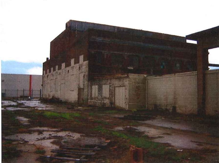
Northern wall of power plant building.
