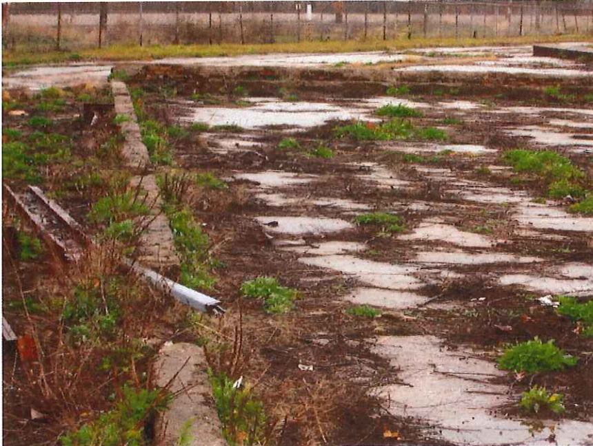
Remnants of building footings located near southern Property boundary.
