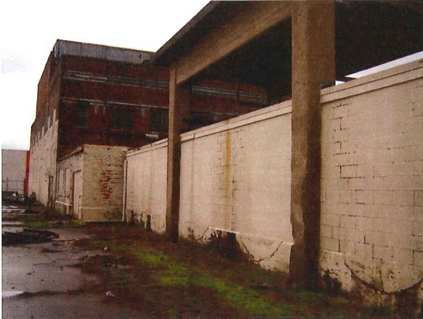
Northern wall of power plant building looking east.
