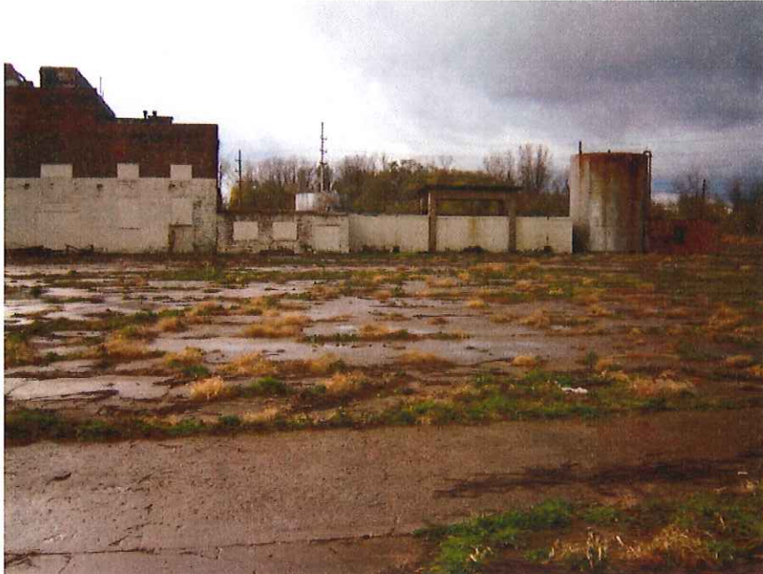
Photo of power plant building looking southward.
