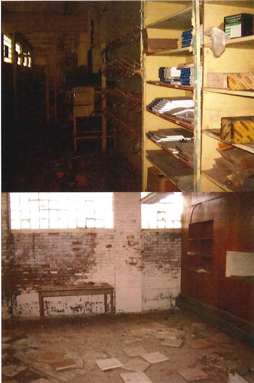
Office and records room located inside power plant building.
