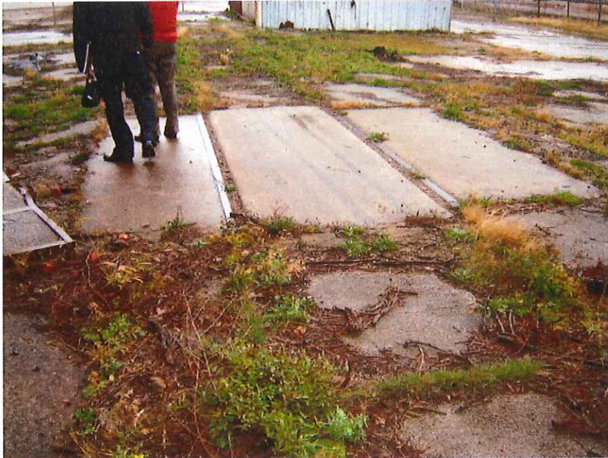
Rail spur located near power plant building.
