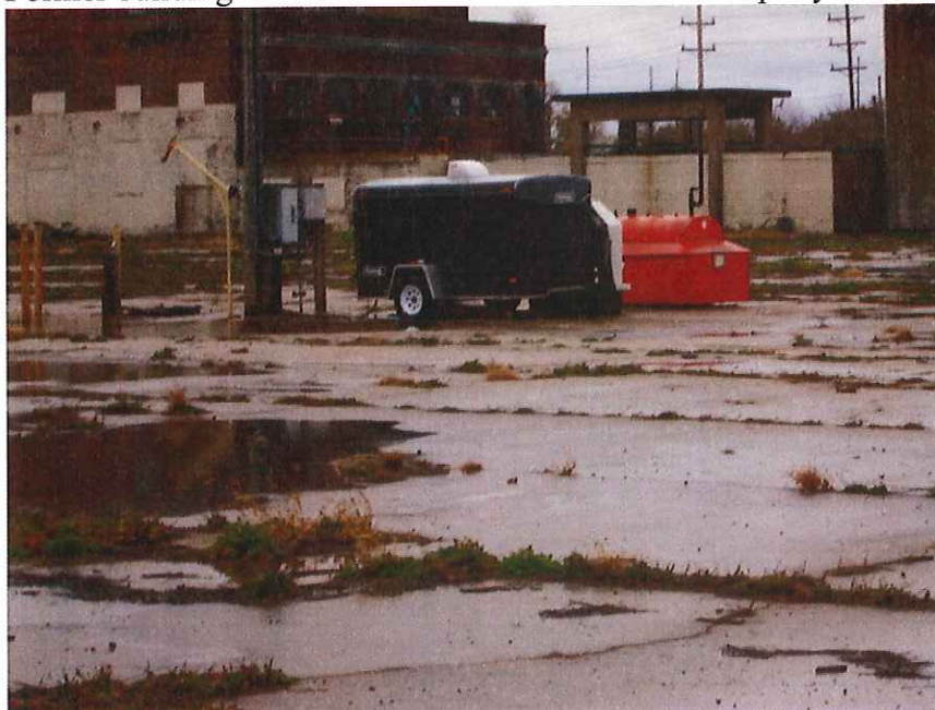
Naptha Free Product Recovery System centrally located on Property?
