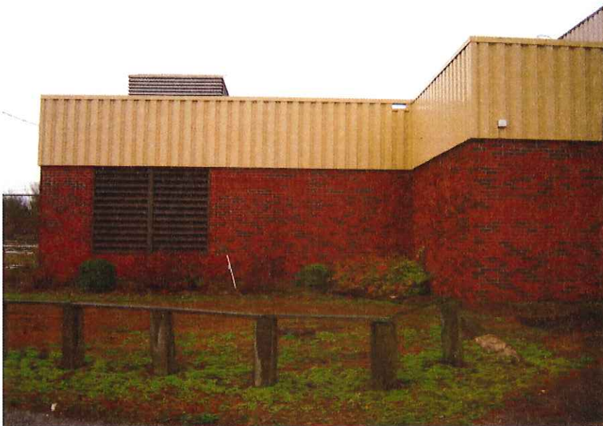
Photo of Bldg 501 located at the northwest corner of Property.
