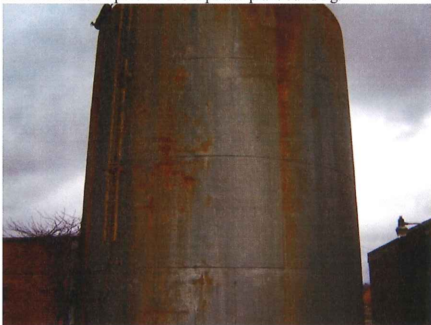
Empty water tank.
