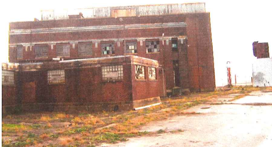
Photo of western portion of the power plant building.
