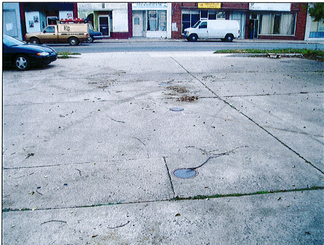
Subject site - UST system fillports (three)
