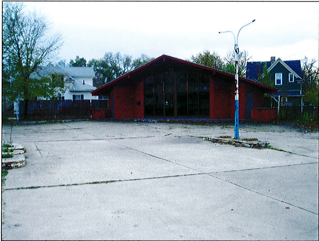
Subject property - existing building and dispenser islands
