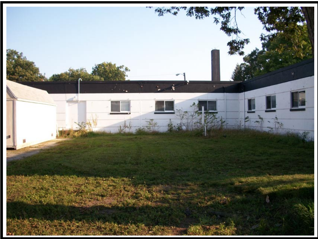
Photo No. 1: View looking north at subject site and location of tank pit area. Note Vent Pipe and fill port in grassed area.
