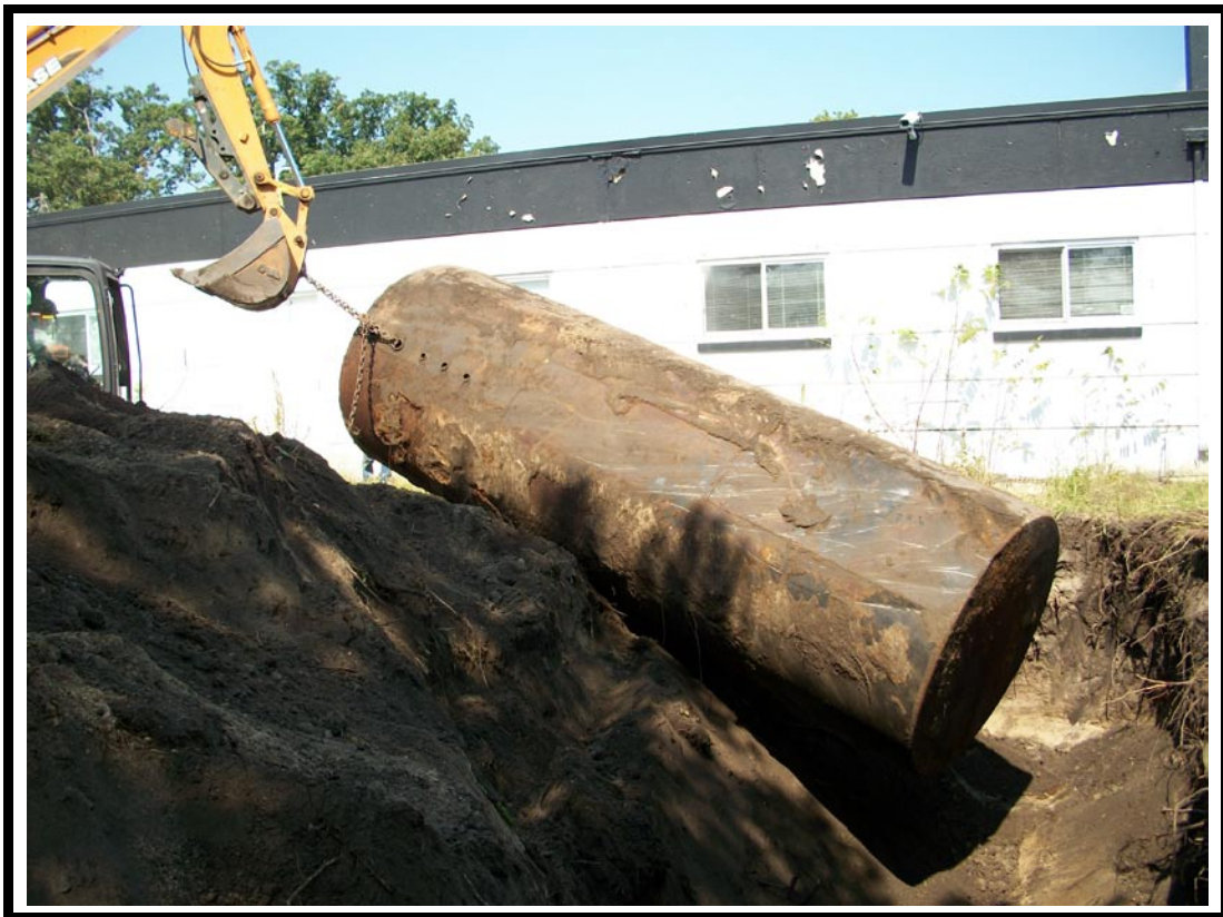
Photo No. 5: View of UST being removed from excavation pit.
