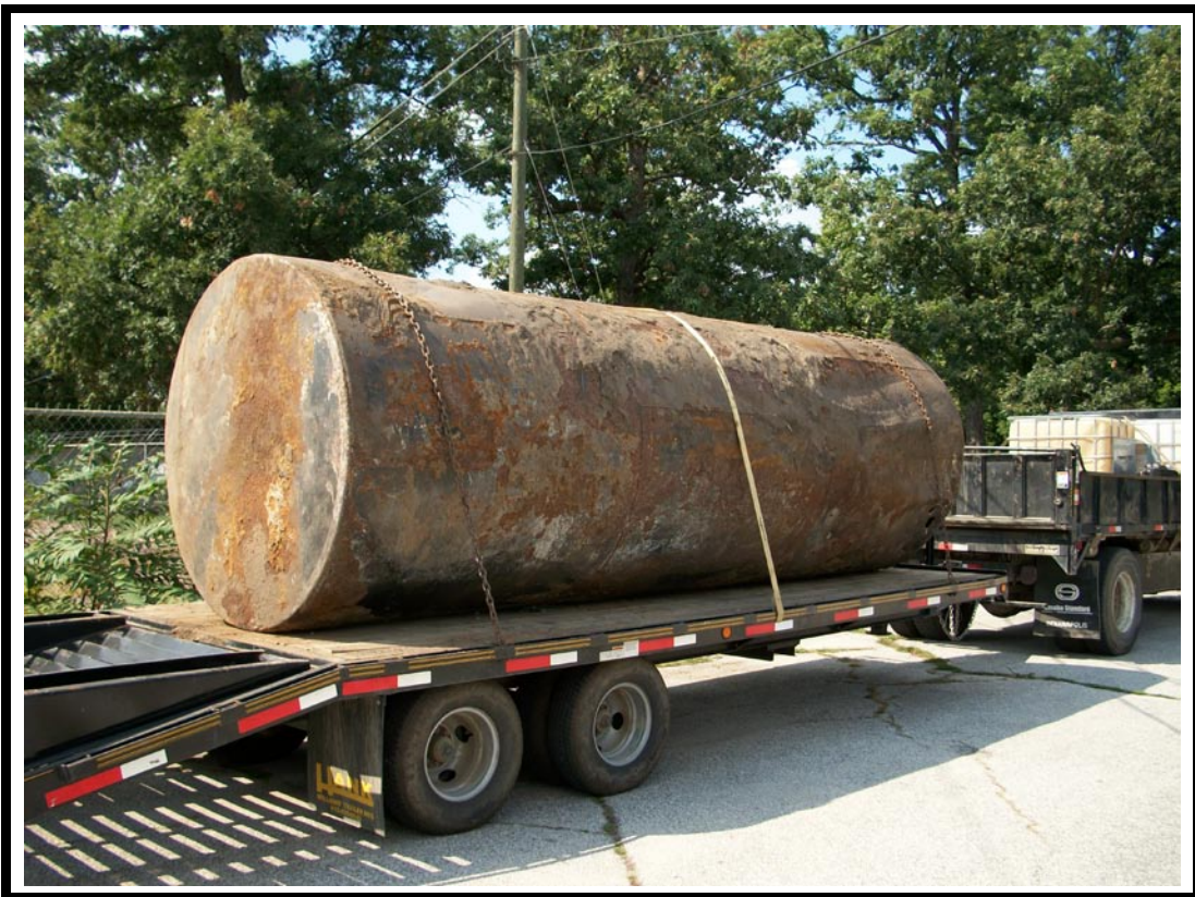
Photo No. 7: View of staged UST prepared for offsite removal and disposal
