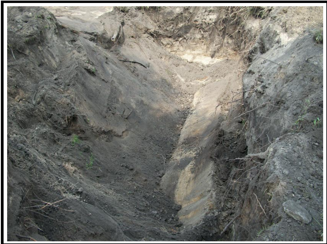
Photo No. 6: View of tank pit after removal of UST.
