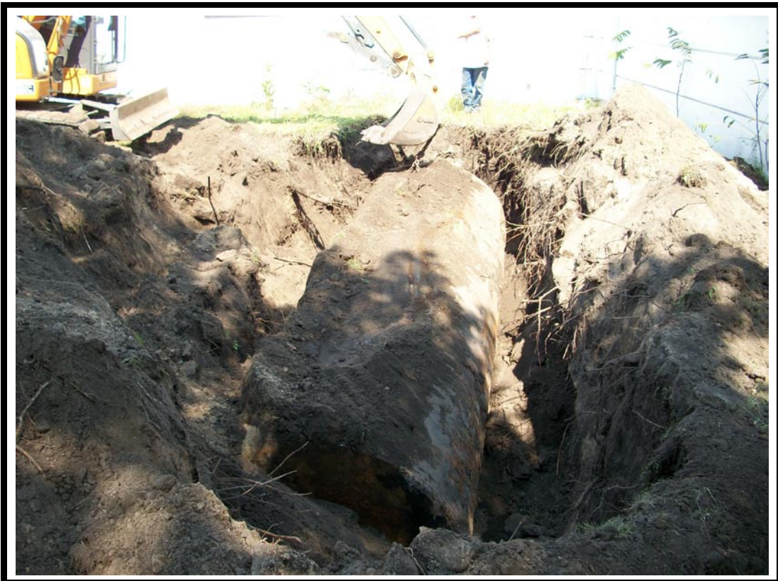
Photo No. 4: View looking north of exposed UST.
