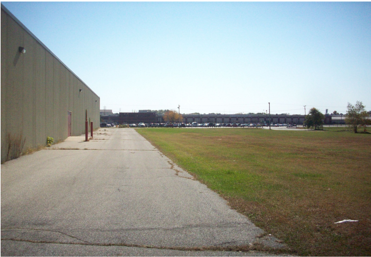
View along west side of subject site building
