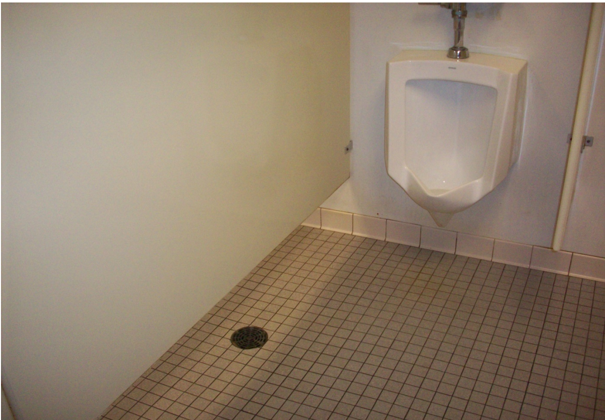
Tile floor and drain in public restroom (typical)
