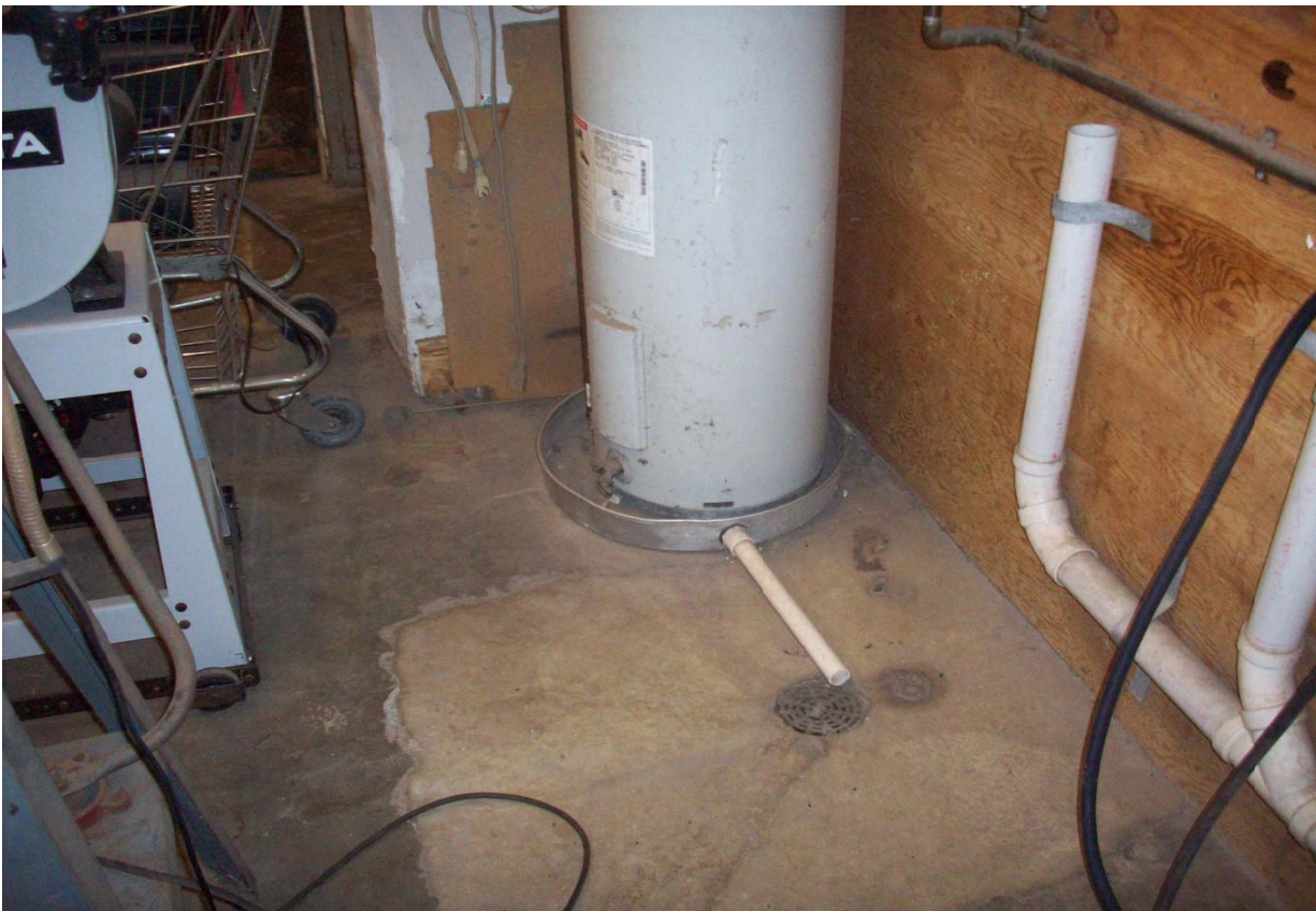
Floor drain from hot water heater in appliance test area
