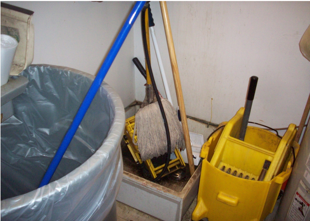
Slop sink and drain in janitorial closet
