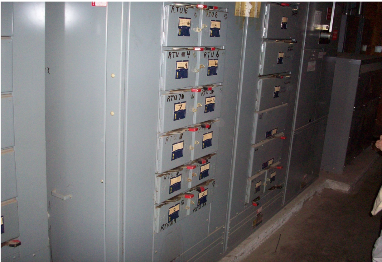
Electrical switch room
