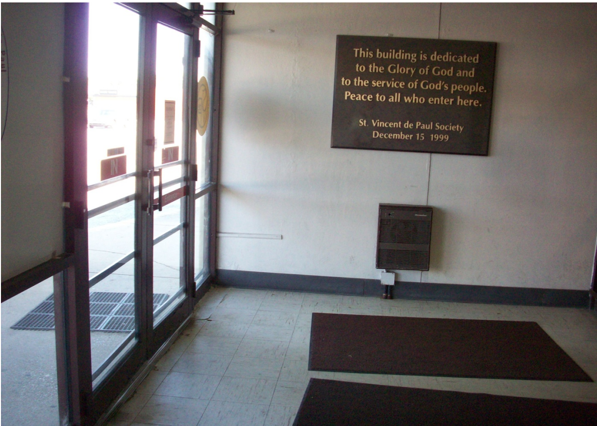
Electrical heater at entry to retail center
