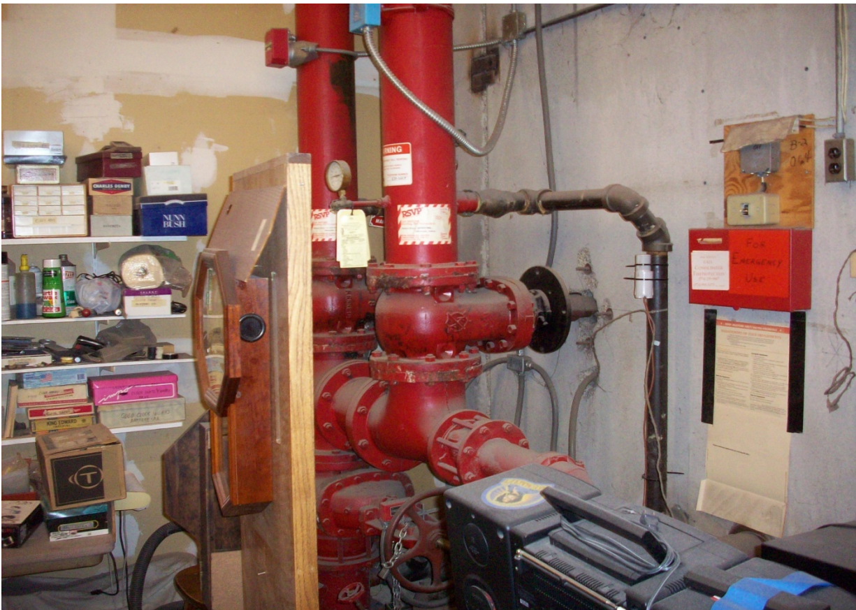
Fire protection system – connection to municipal water supply
