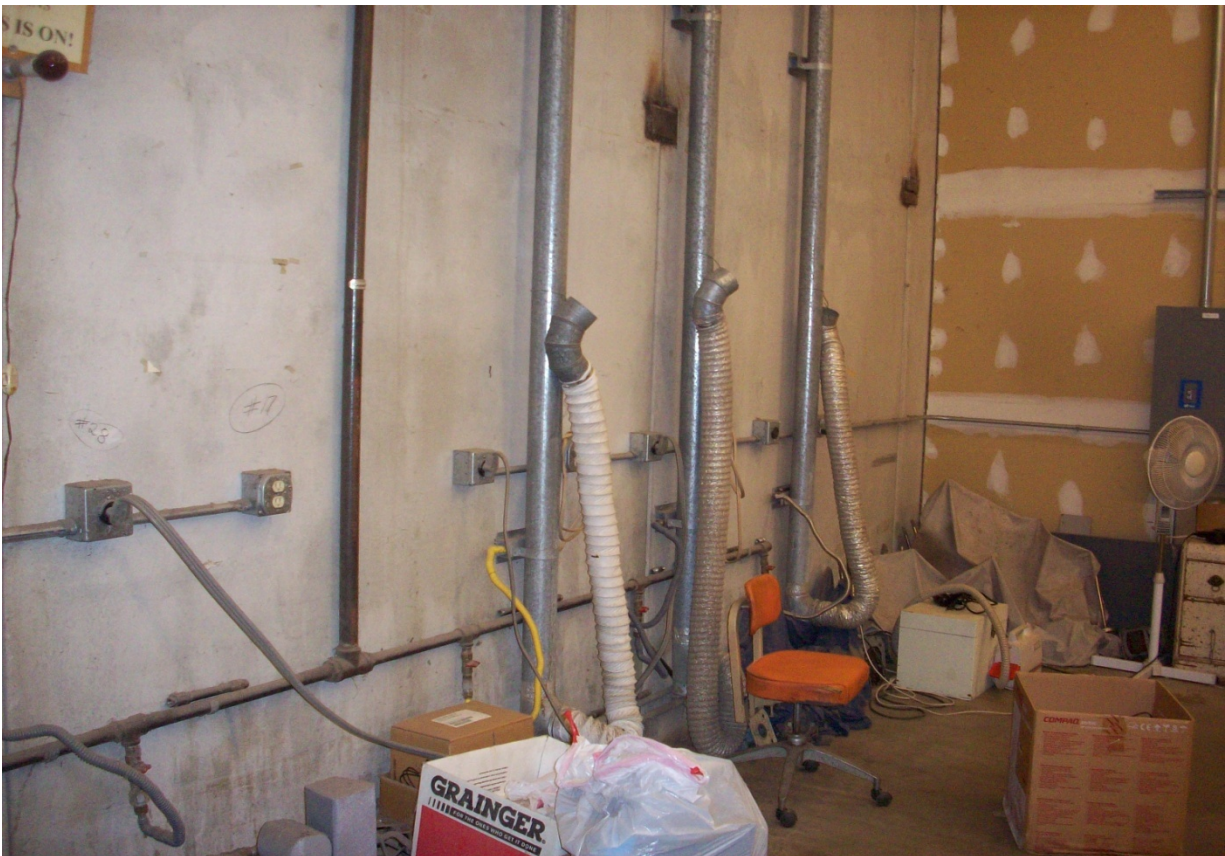
Exhaust vents in appliance test area
