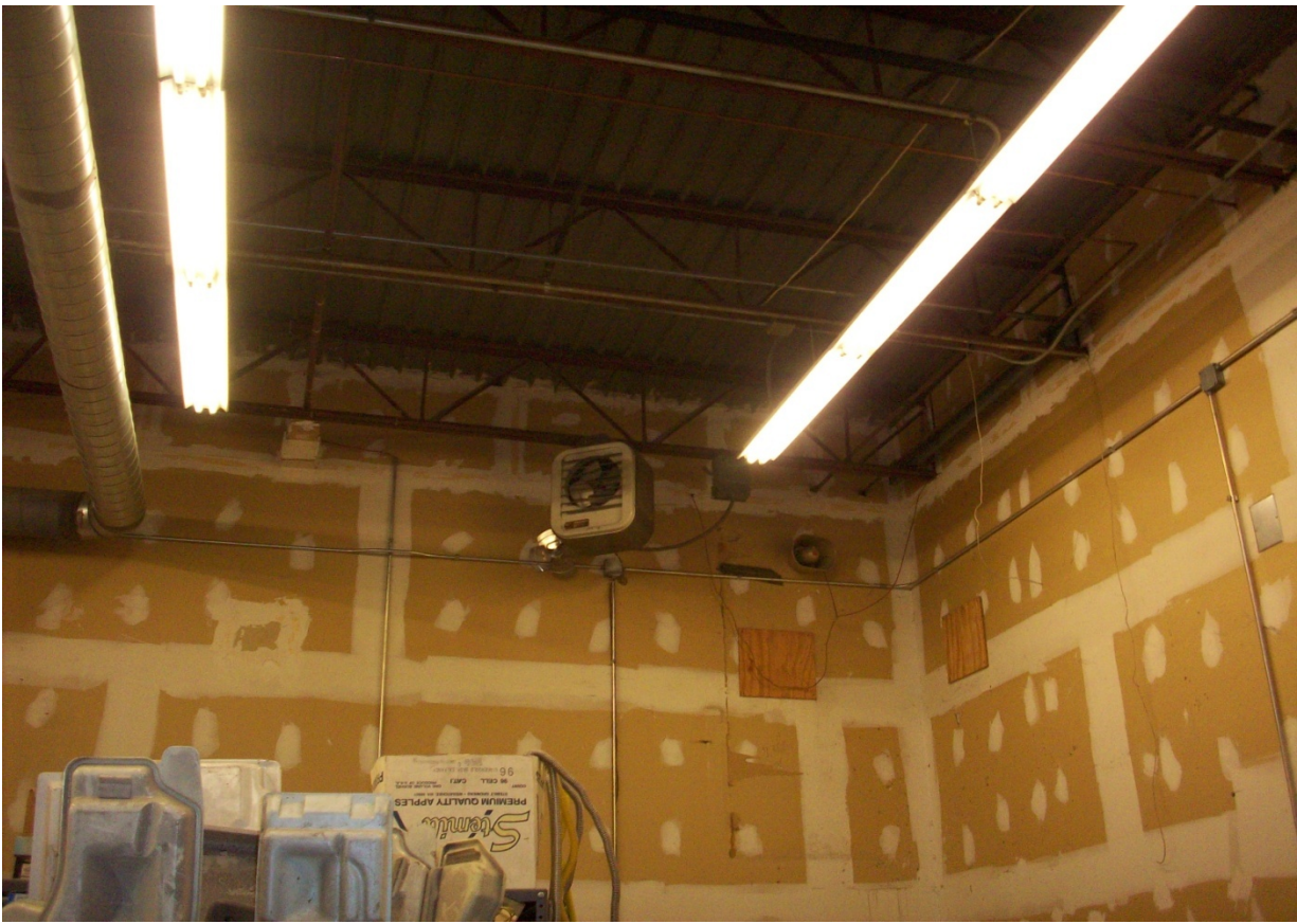
Hanging electrical heater unit (typical throughout facility)
