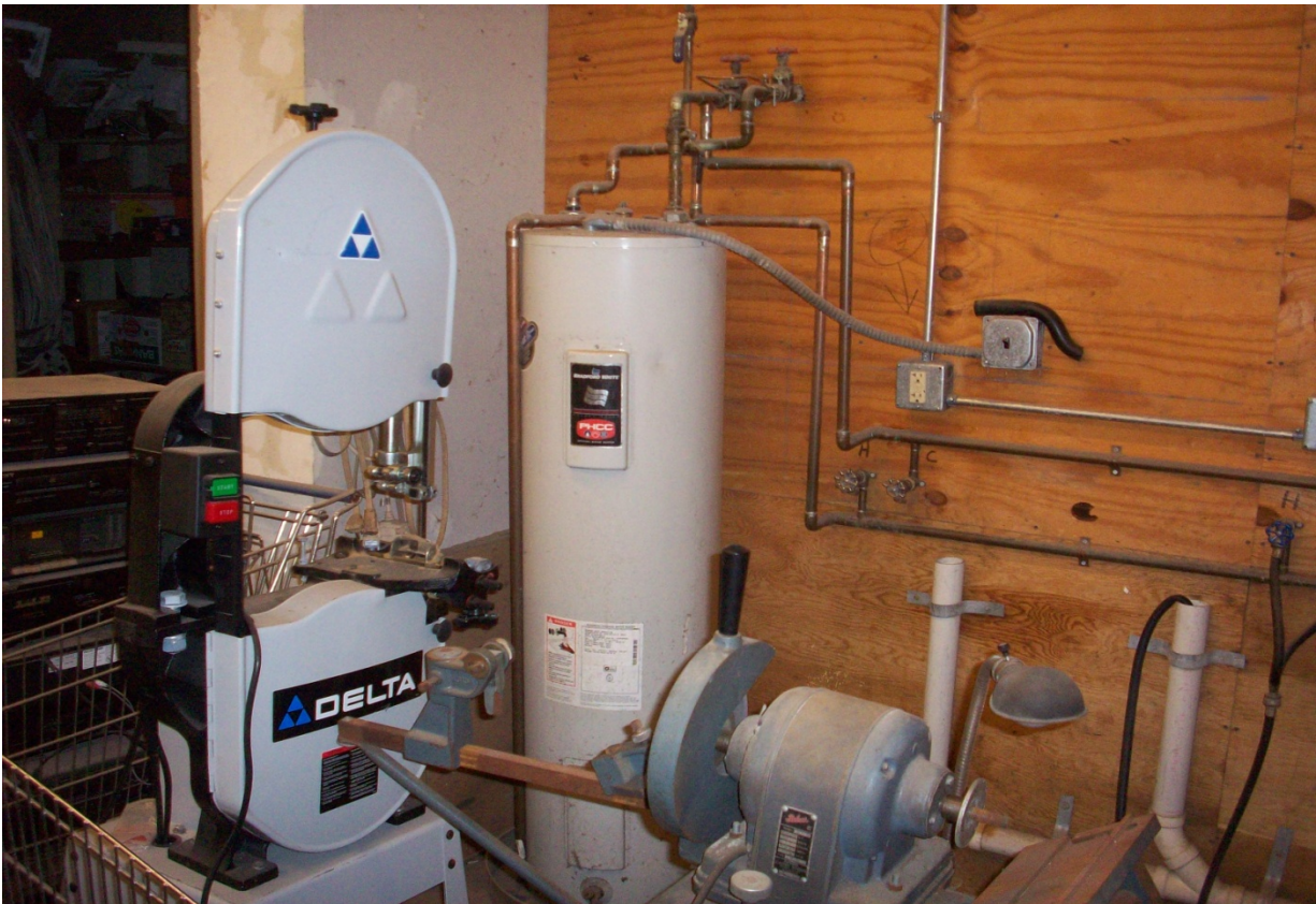
Electric hot water heater in appliance test area
