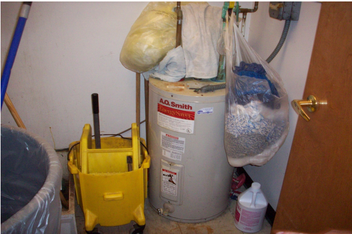
Electrical hot water heater in janitorial closet
