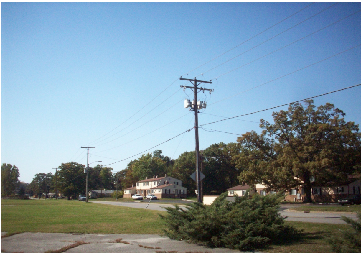
Pole-mounted transformers along Ardmore Trail at northern property boundary
