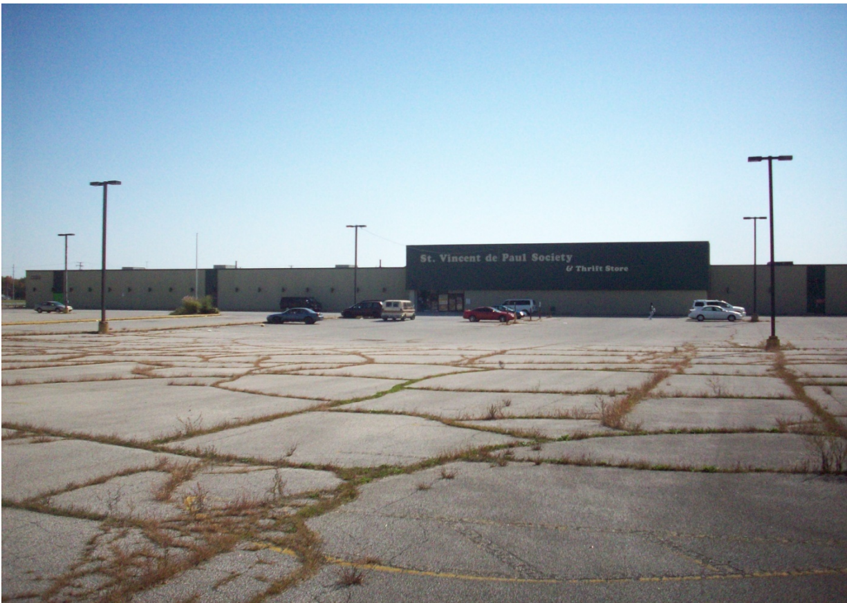
Frontal view of subject site
