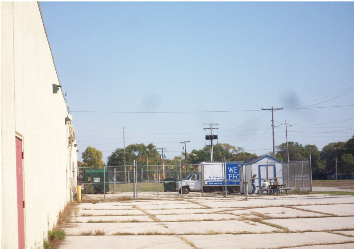
South side of subject site building, fenced area
