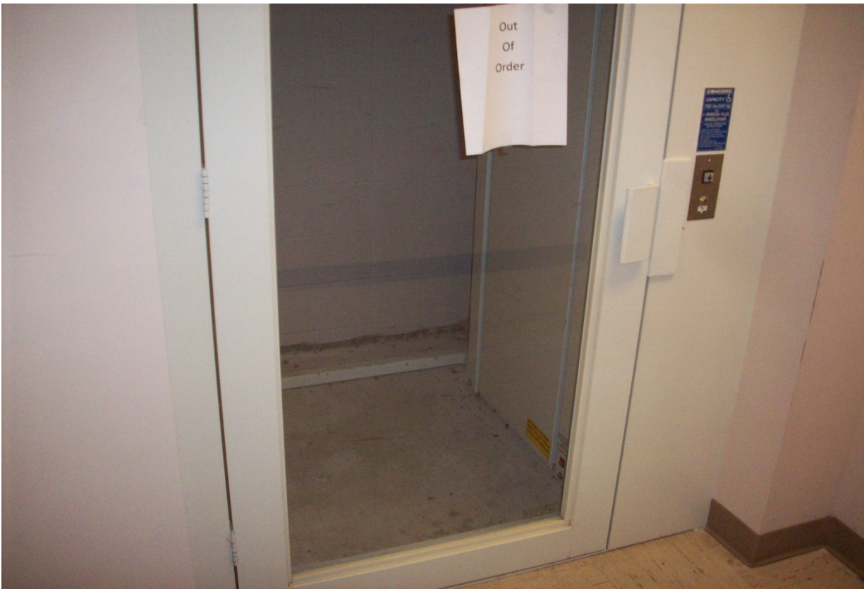
Wheelchair lift between ground and mezzanine levels
