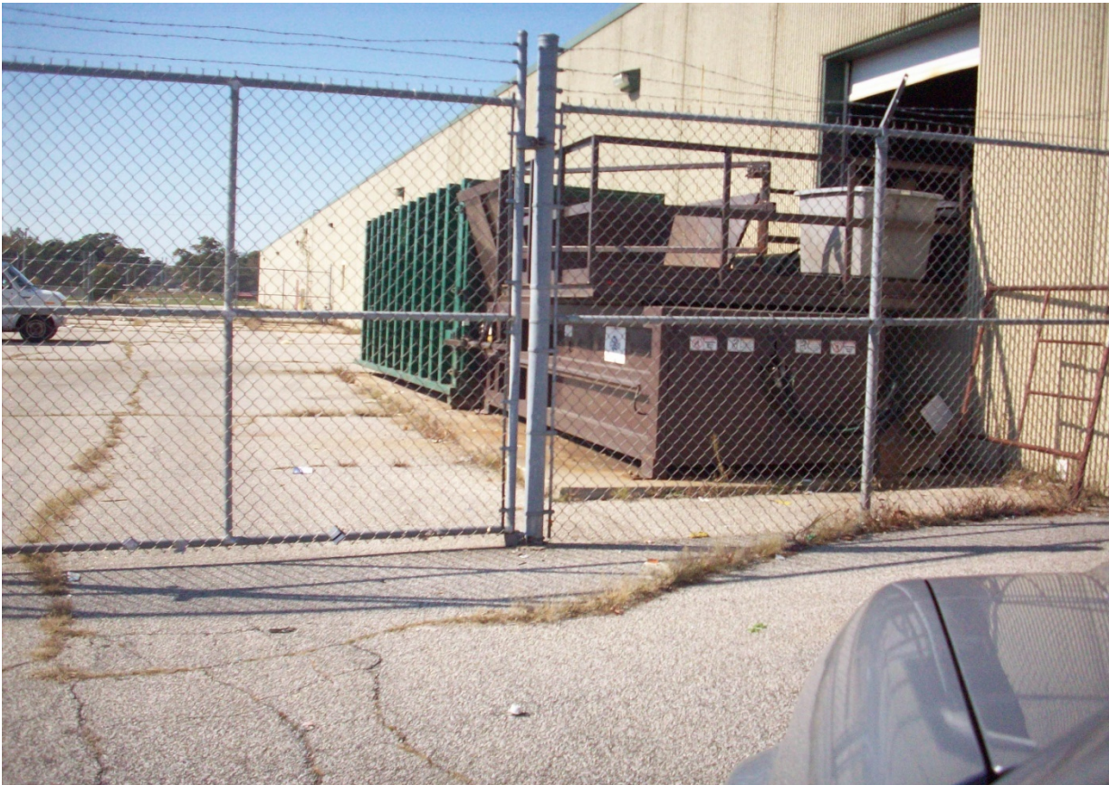
Hydraulic compactor at southeast corner of building, near donation drop-off
