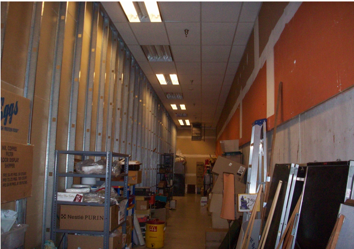
Hanging natural gas furnace unit in front storage area - Non-operational (1 of 2)
