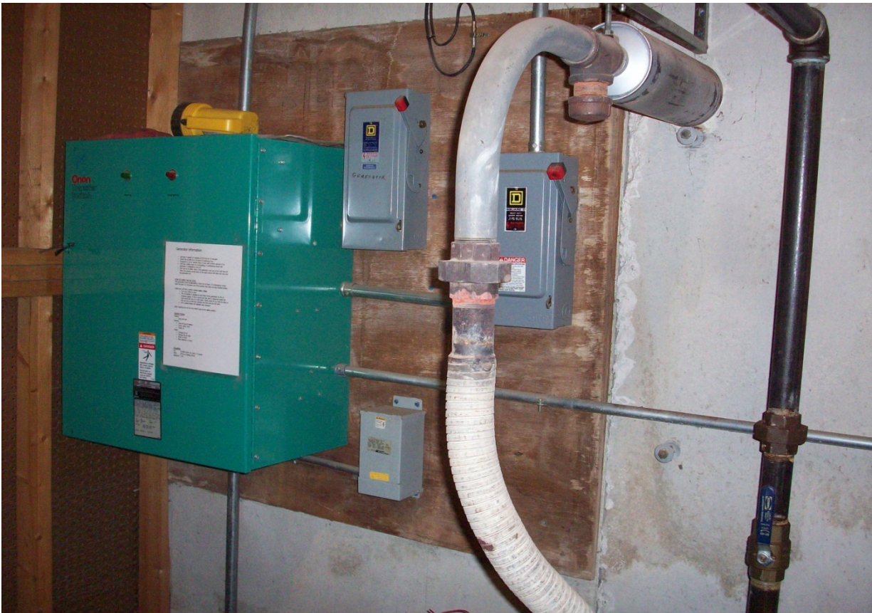
Controller and exhaust to outside for emergency generator
