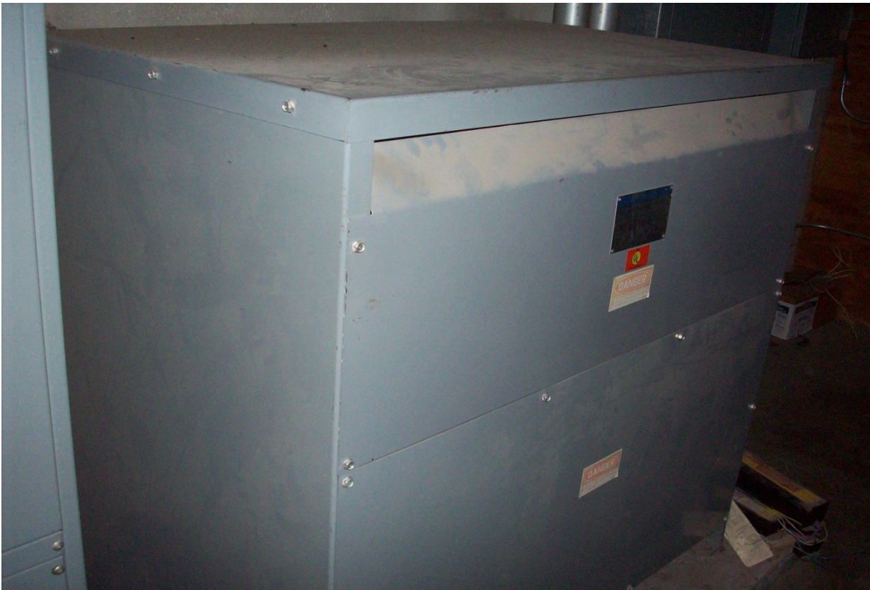
Dry-type transformer in electrical switch room
