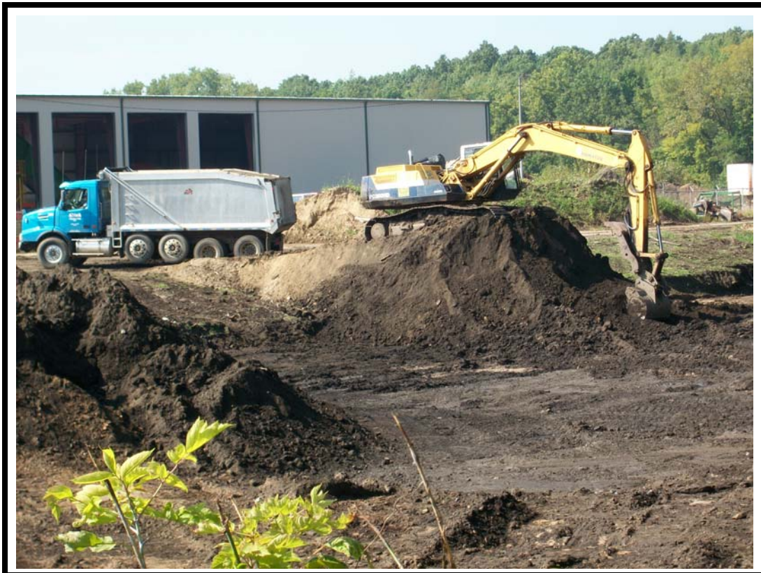
Photo No. 8: View of removal of staged soils for offsite disposal.
