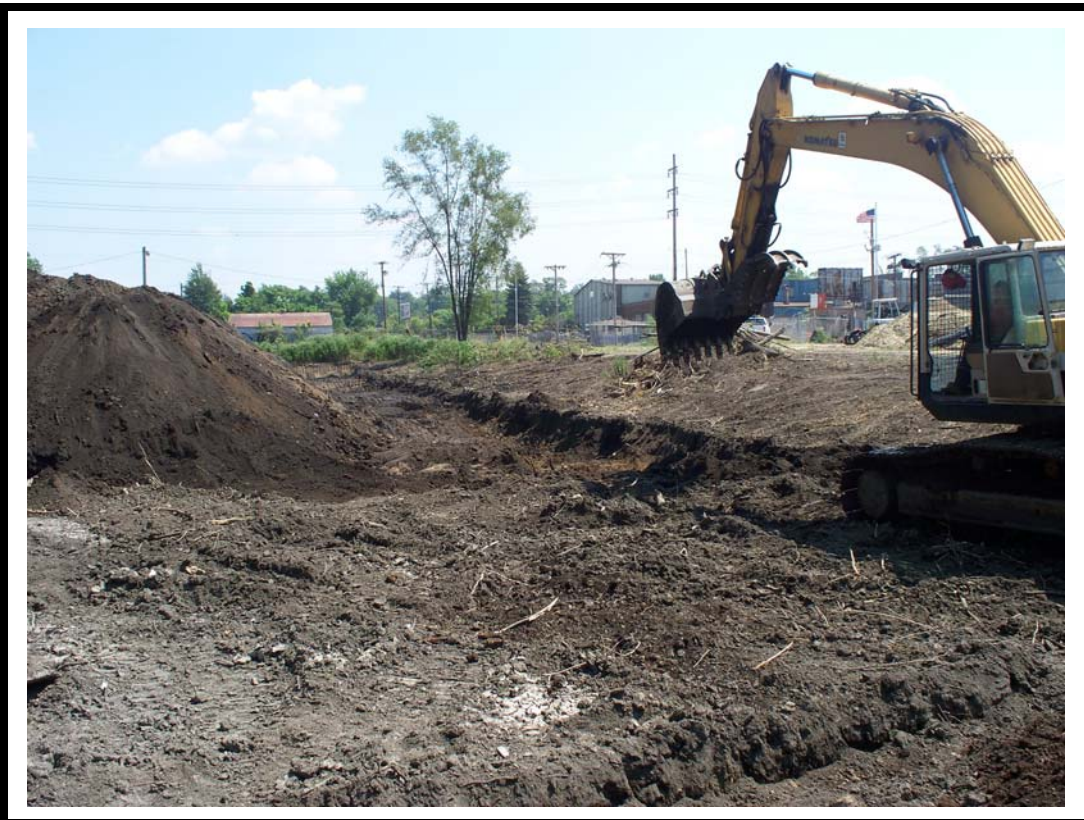
Photo No. 4: View looking northeast of northern extent of excavation.
