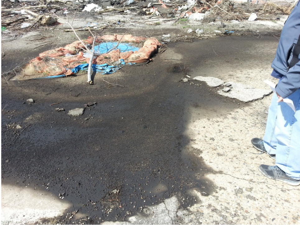
#31: Oil stain at the northwest of the Property, close to the gas house. The tarp-and-sandbag area corresponds to the approximate location of another groundwater monitoring well installed by a previous investigator.
