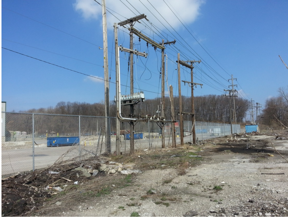
#27: Derelict utility poles at the western edge of the Property. The oily stain can be seen at the right of the photo.
