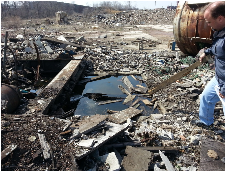
#26: Water-filled pit behind the furnace. The plank being held was used to test the depth of the pool. It was at least four feet deep.
