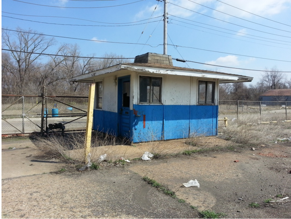
#33: Exterior of the gate house.
