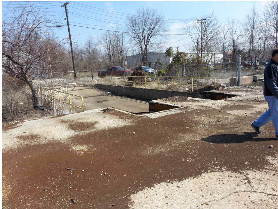
#38: Loading dock located at the northeastern corner of the Property.
