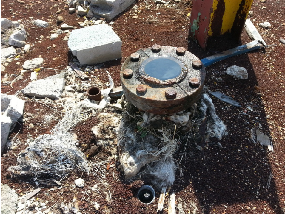
#37: Close-up of the pipe depicted in photo #36.
