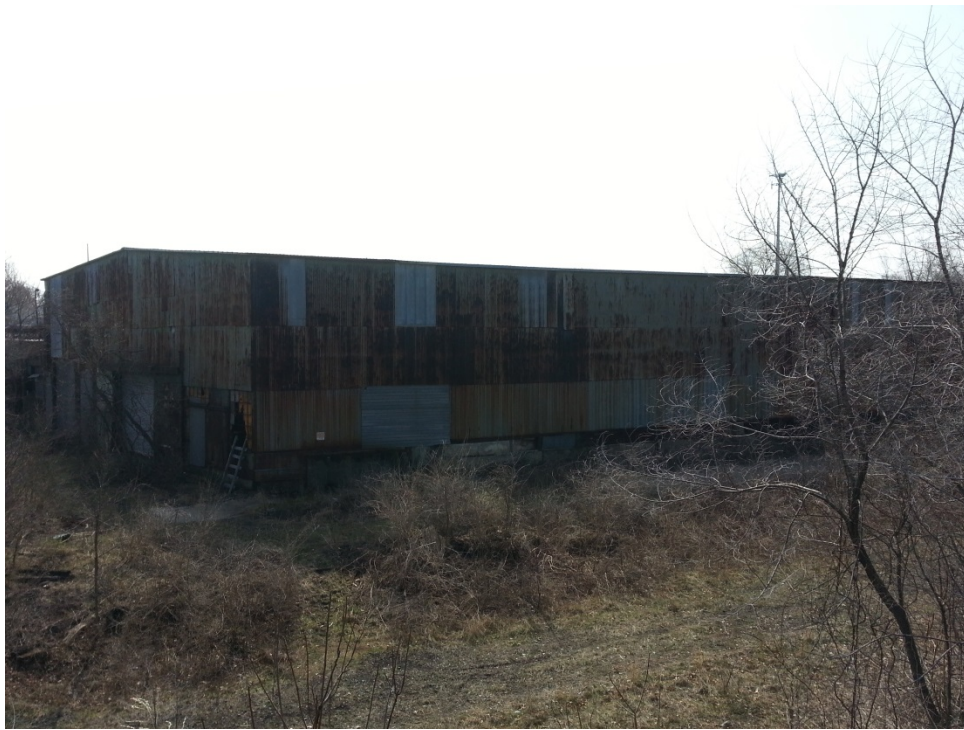
#11: Photo taken from the highest point of the Property, facing southeast. The large building was formerly used for manufacturing steel.
