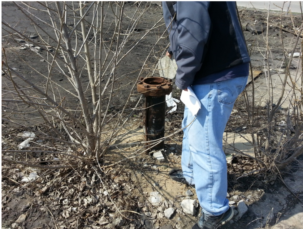
#18: One of the suspected wells at the western edge of the former foundry building. This pipe was covered with a slab of concrete (being held up).
