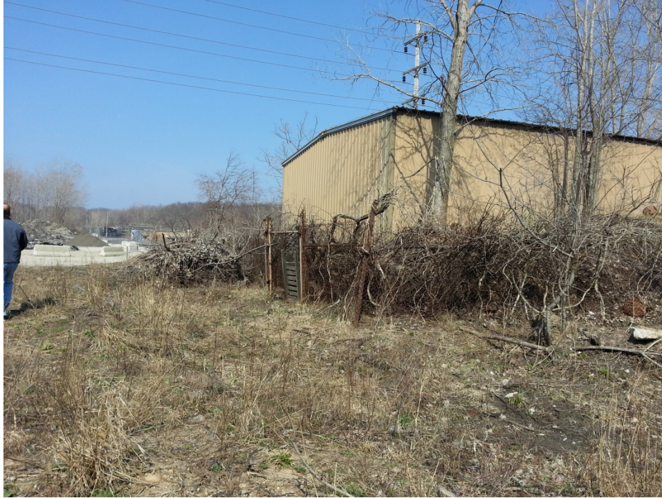
#7: The backside of warehouse, at the southernmost edge of the Property.
