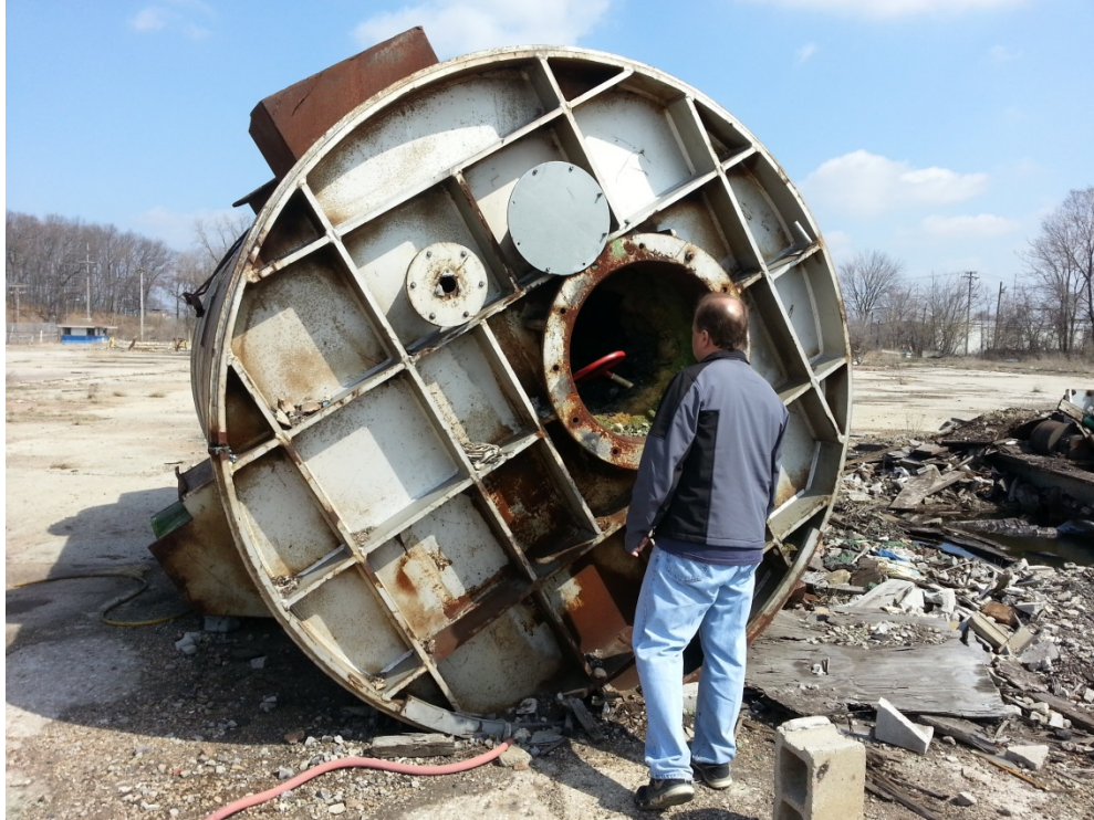
#21: This photo provides a scale for the furnace's size.
