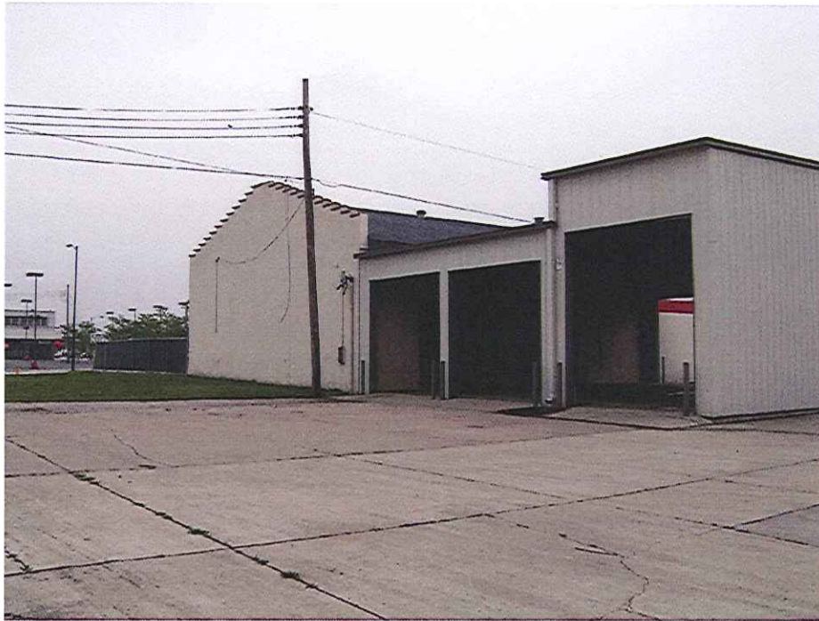
North side of building
