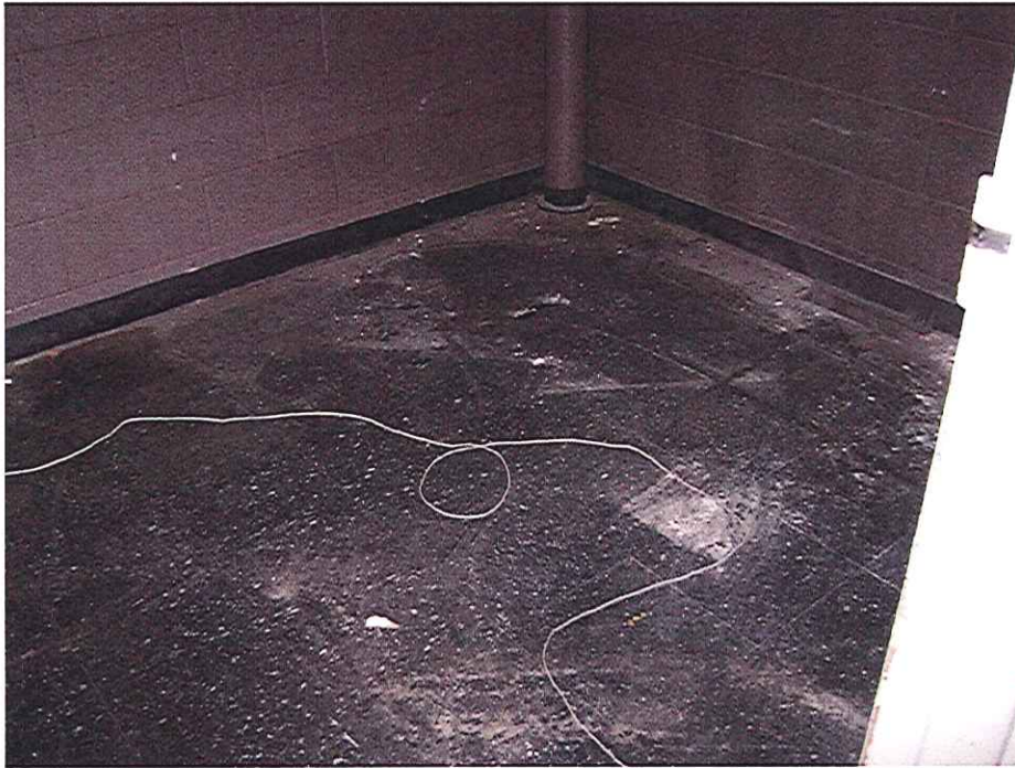
Black floor tile and mastic (ACM) in northeast room
