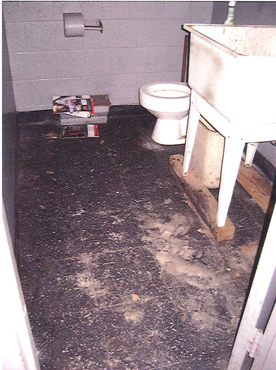
Black floor tile and mastic (ACM) in bathroom
