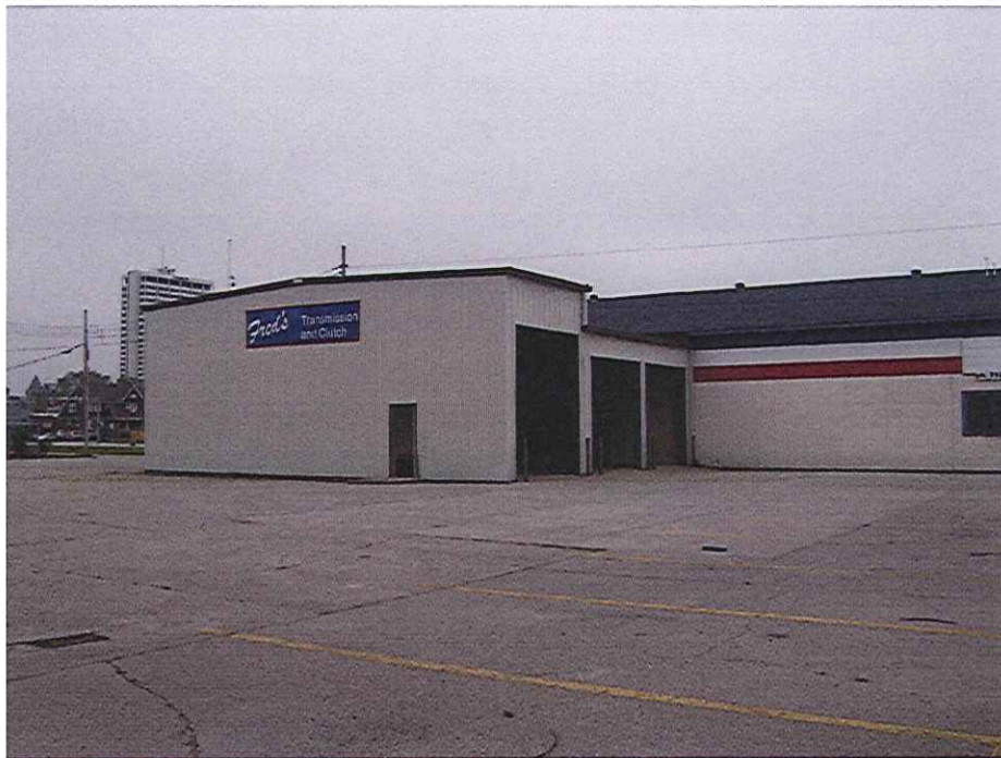
West side of building
