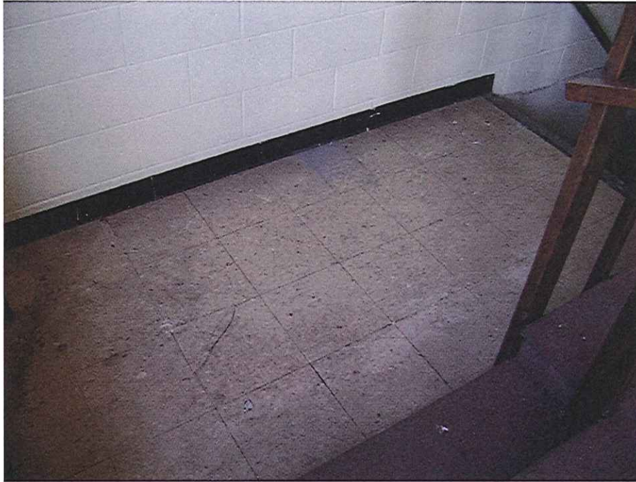
Brown floor tile and mastic (ACM) in south stairwell
