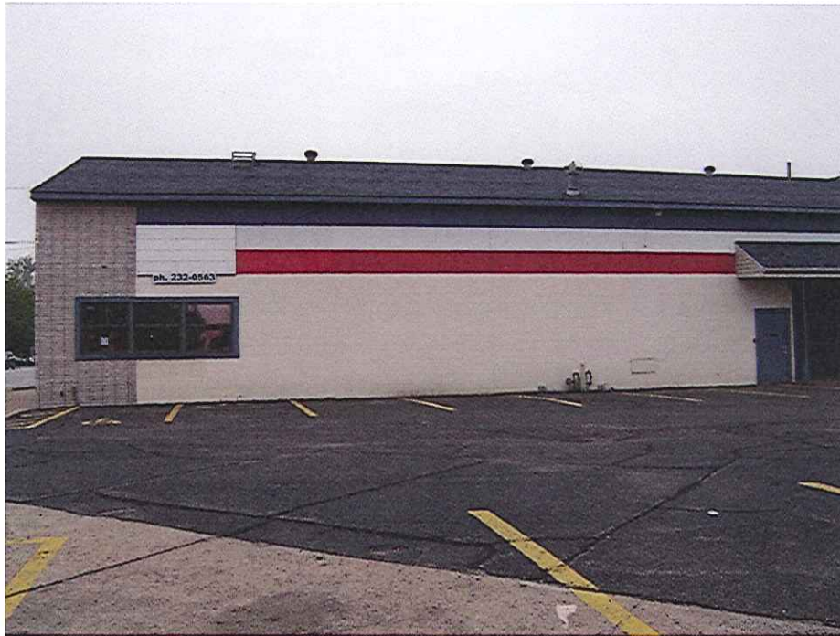
East side of building
