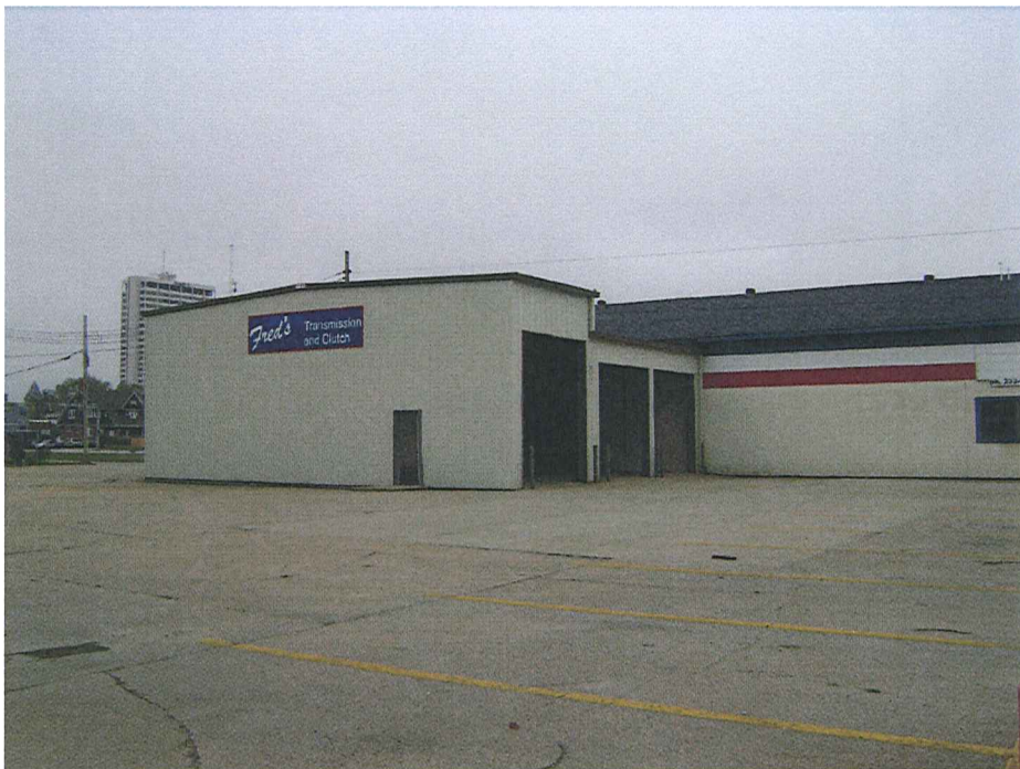
West side of building
