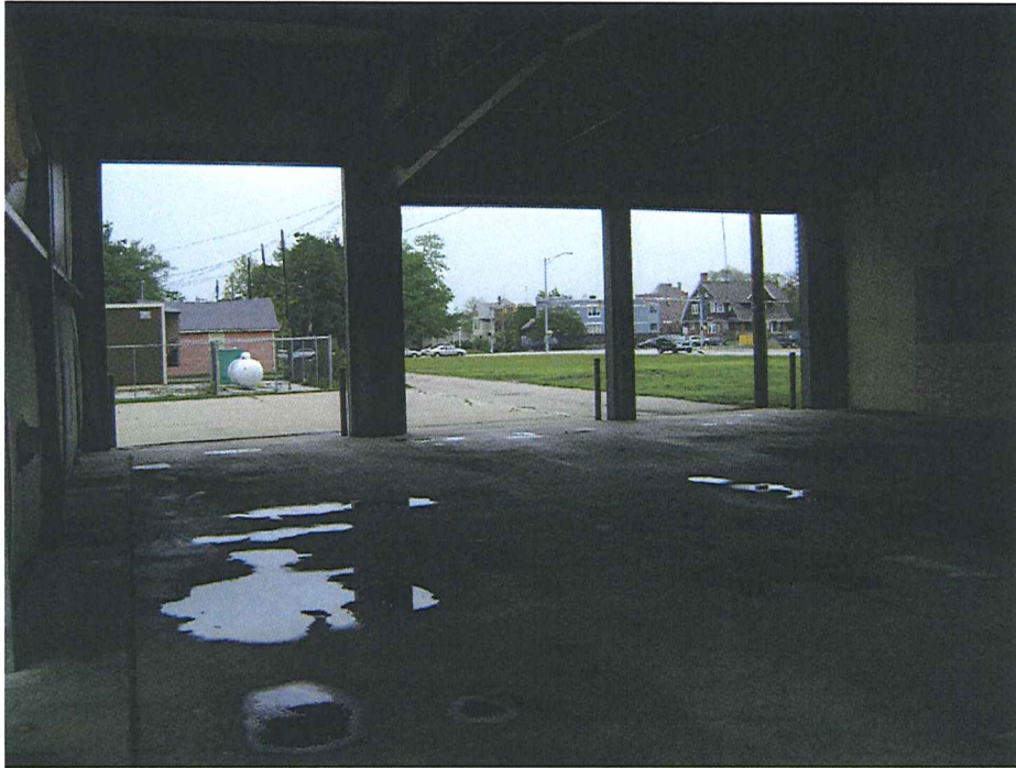
Interior of garage
