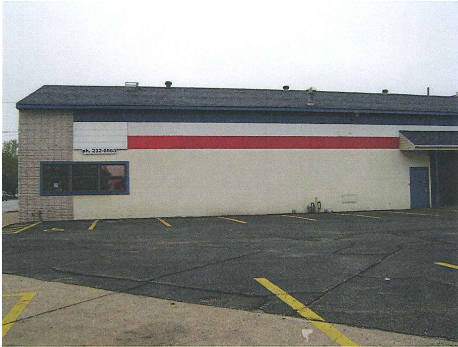
East side of building
