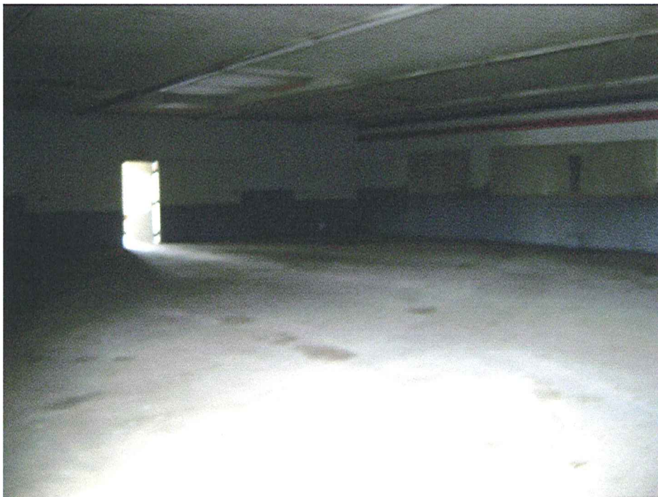
Main room of eastern half of building
