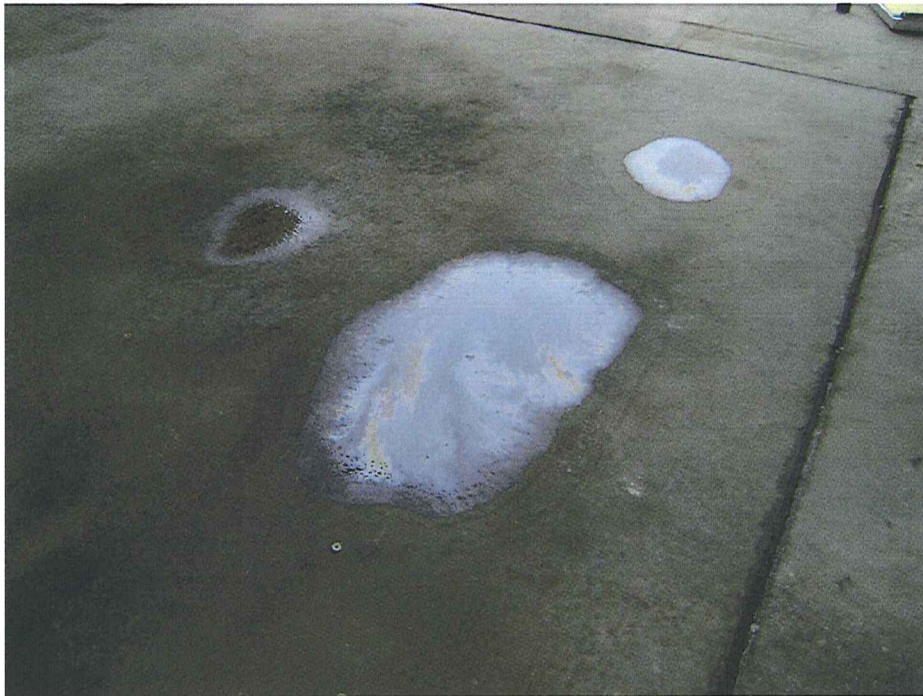
Puddle with oily sheen in garage
