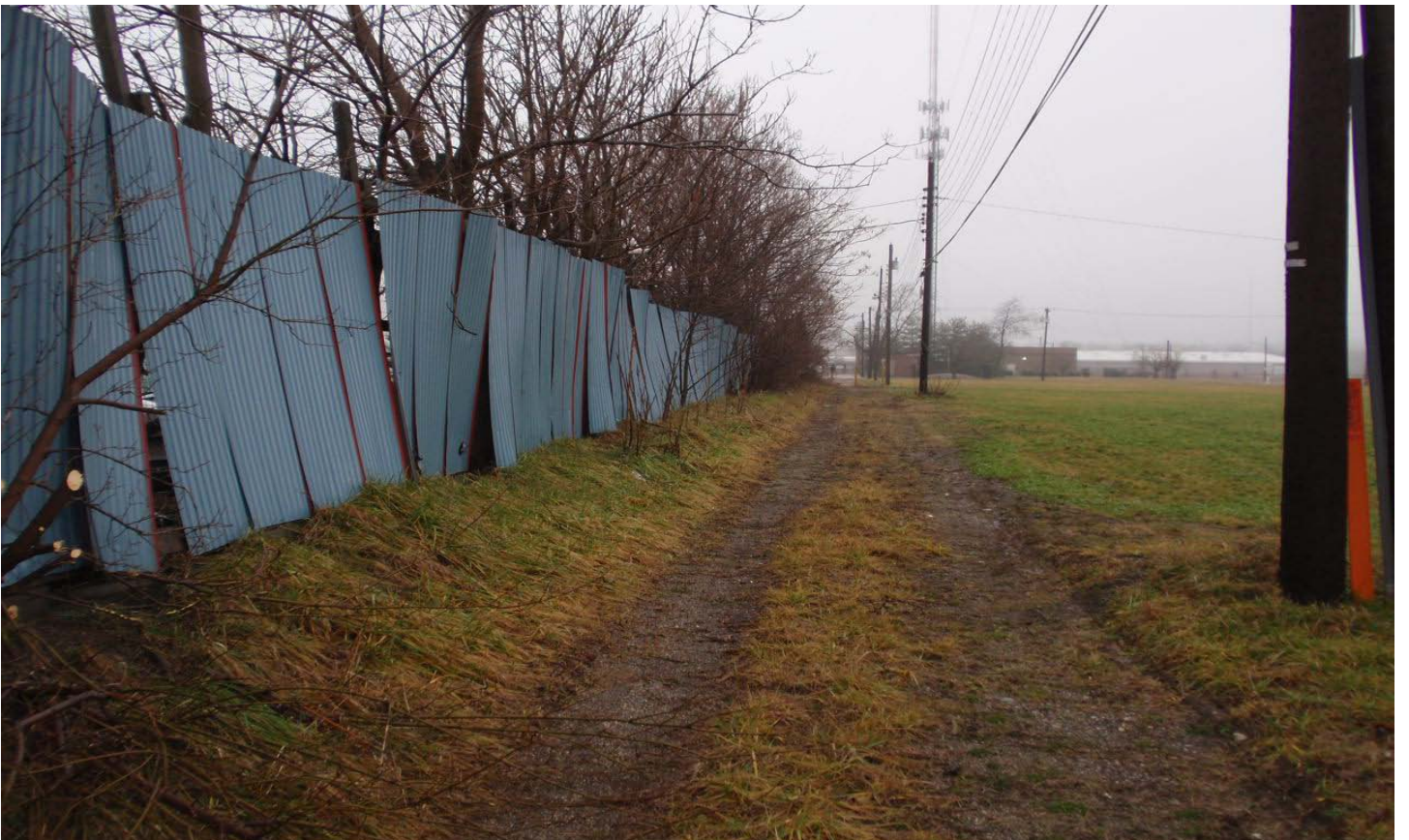
Western Fence Line of Property
