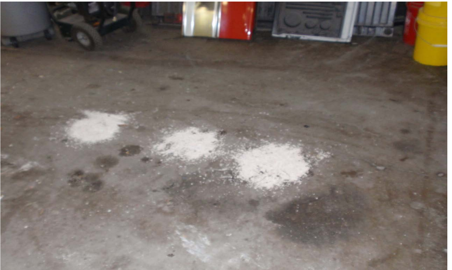
Oil Staining with Floor Dry
