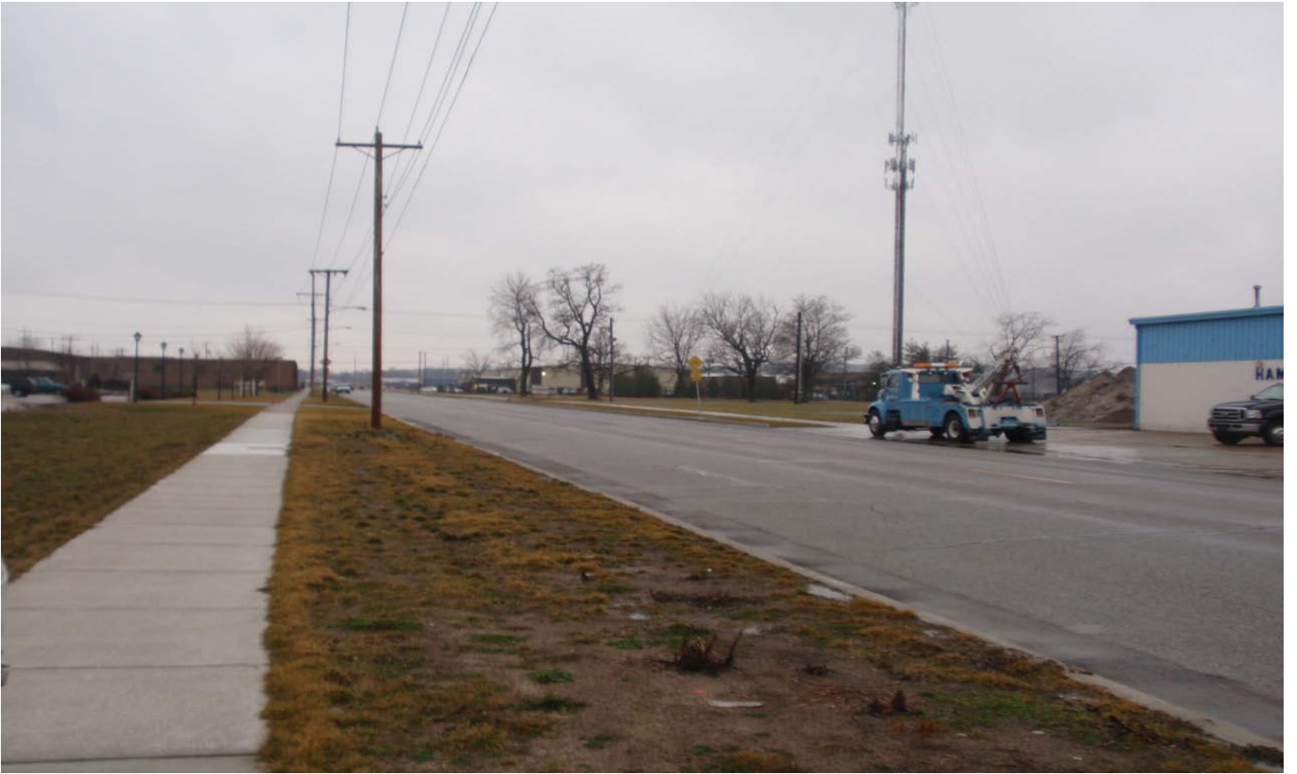
South Lafayette Boulevard with Electrical Lines on the East Side
