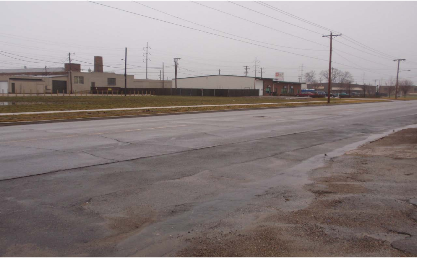
Southeast Adjacent Property
