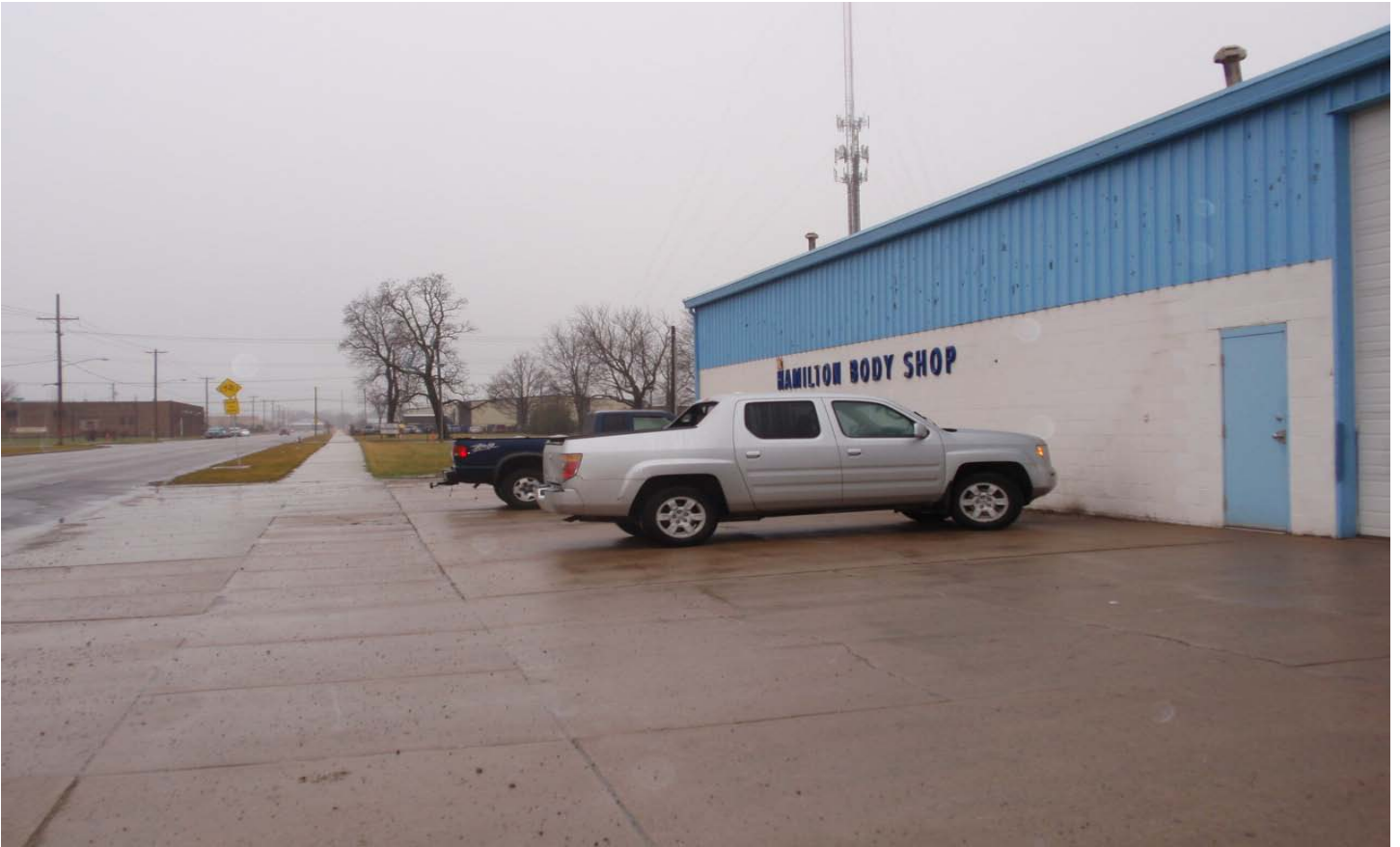
Eastern Side of Main Structure
