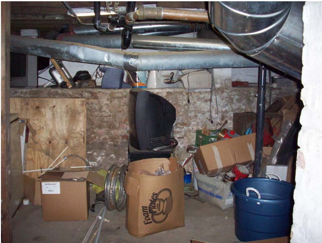
Basement (personal storage)
