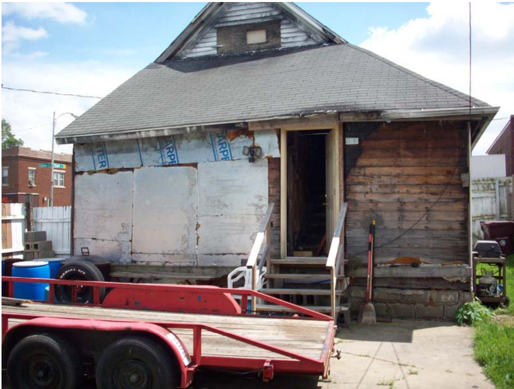
Subject site (rear entry to club house)
