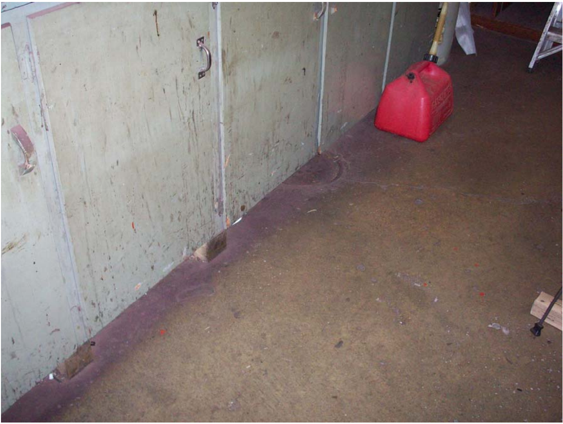
Floor drain beneath existing cabinets (closed)
