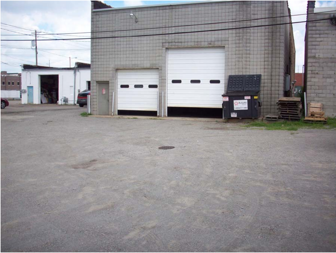
Storm grate (1 of 2) in rear gravel parking lot
