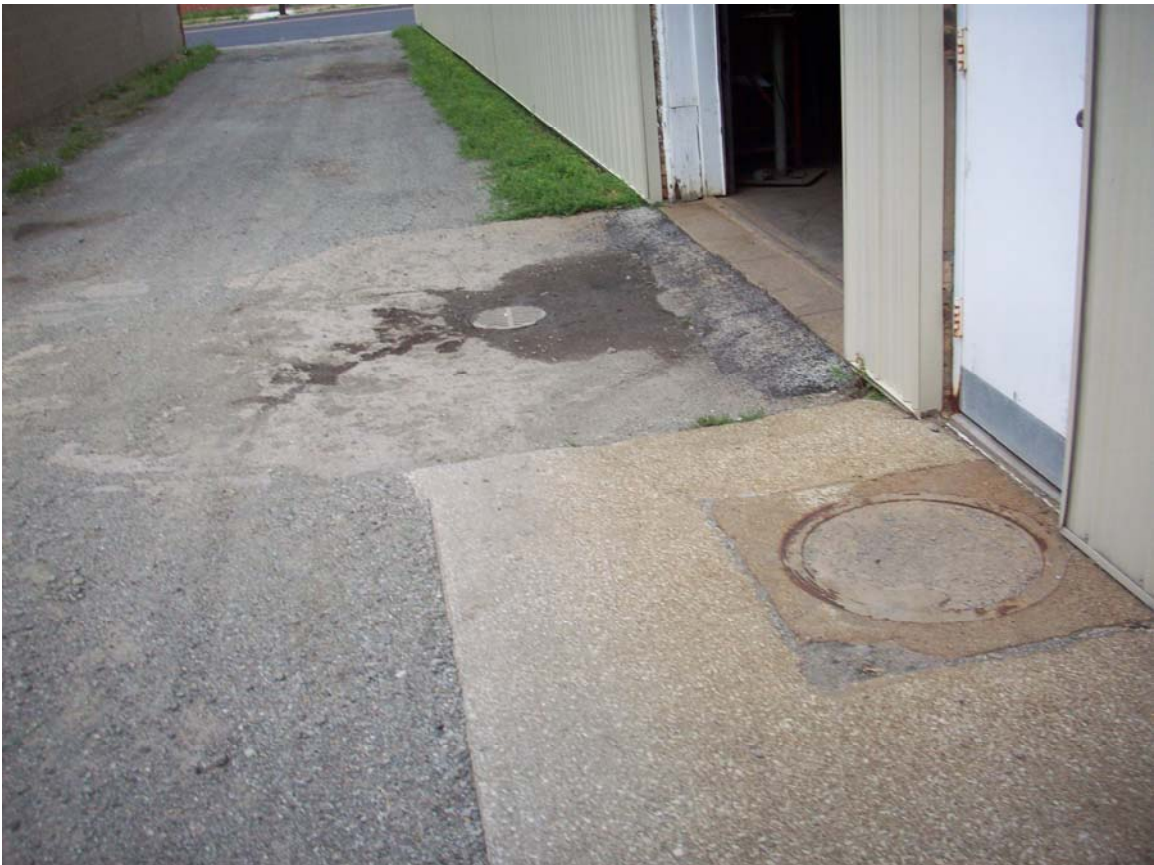
Storm drain at western overhead door, former coal chute
