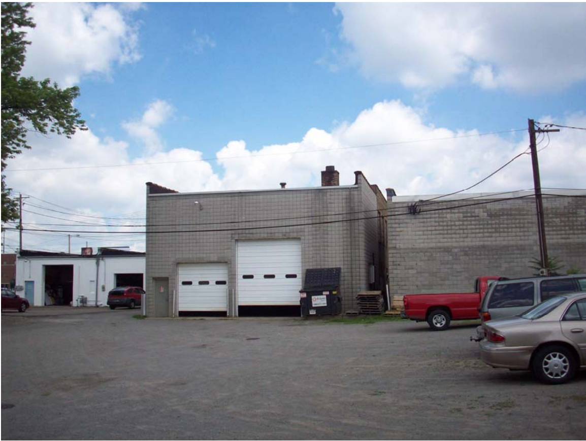
Rear view of Subject site – Looking North
