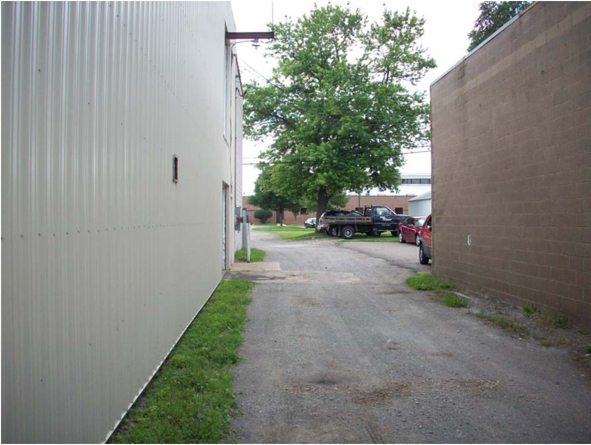
Western property boundary w/adjacent Mason Heating
