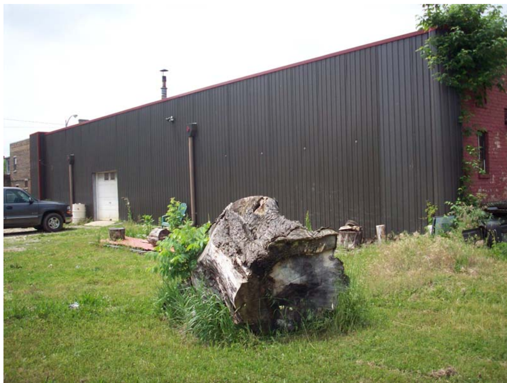
Looking southwest – Barany Sheet Metal 735-747 W. Indiana Ave
