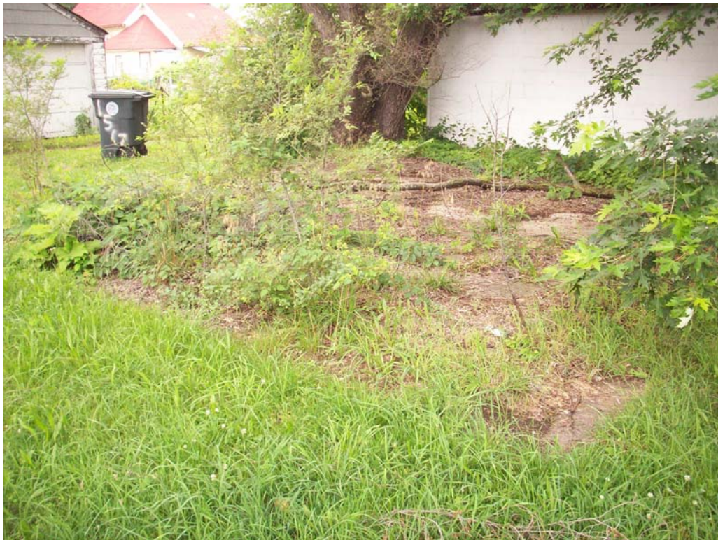
Concrete slab – former detached garage – 1521 Kendall Ave
