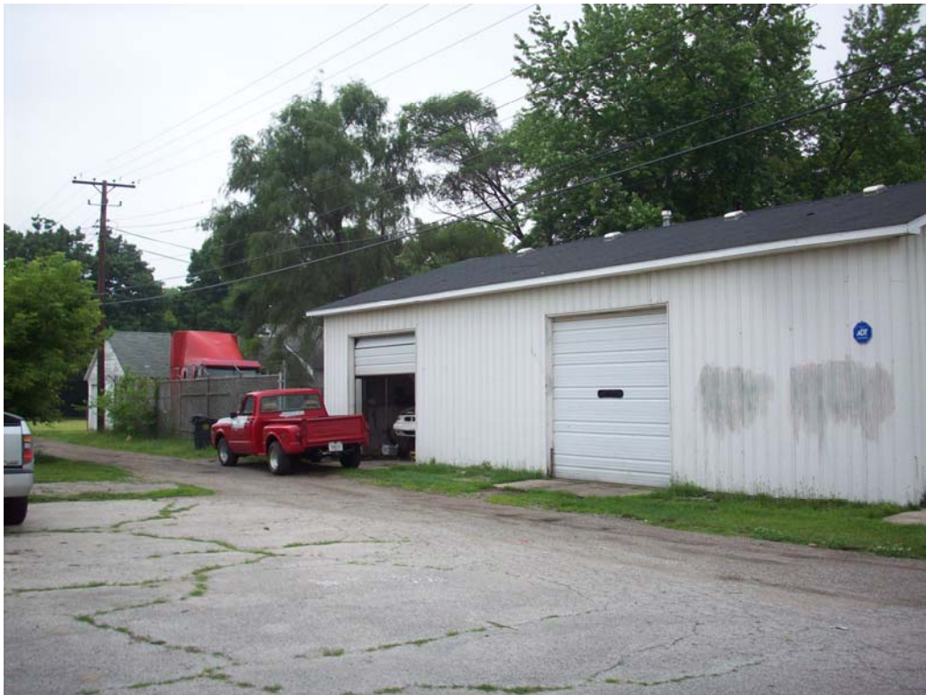
View of subject site garage bldg – 1527 Kendall Ave
