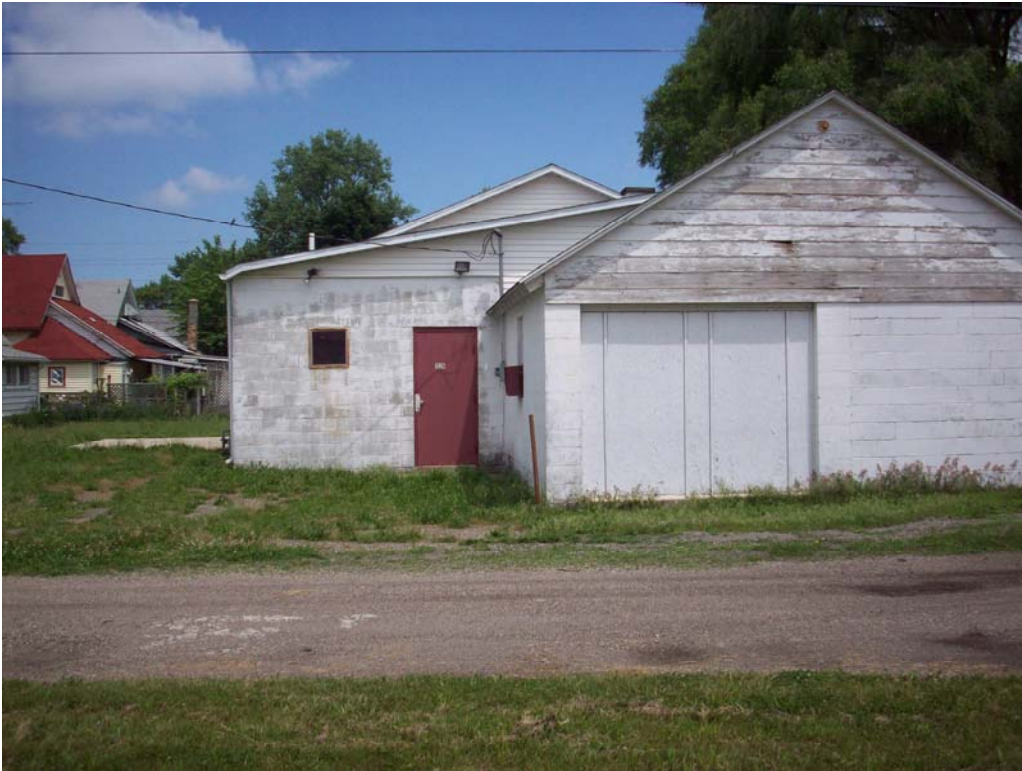
Residential to west of subject site – 1536 Chapin St
