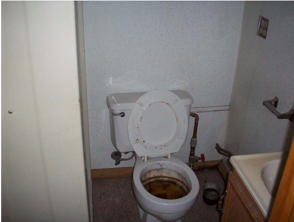
Rest room in office area (water service terminated)
