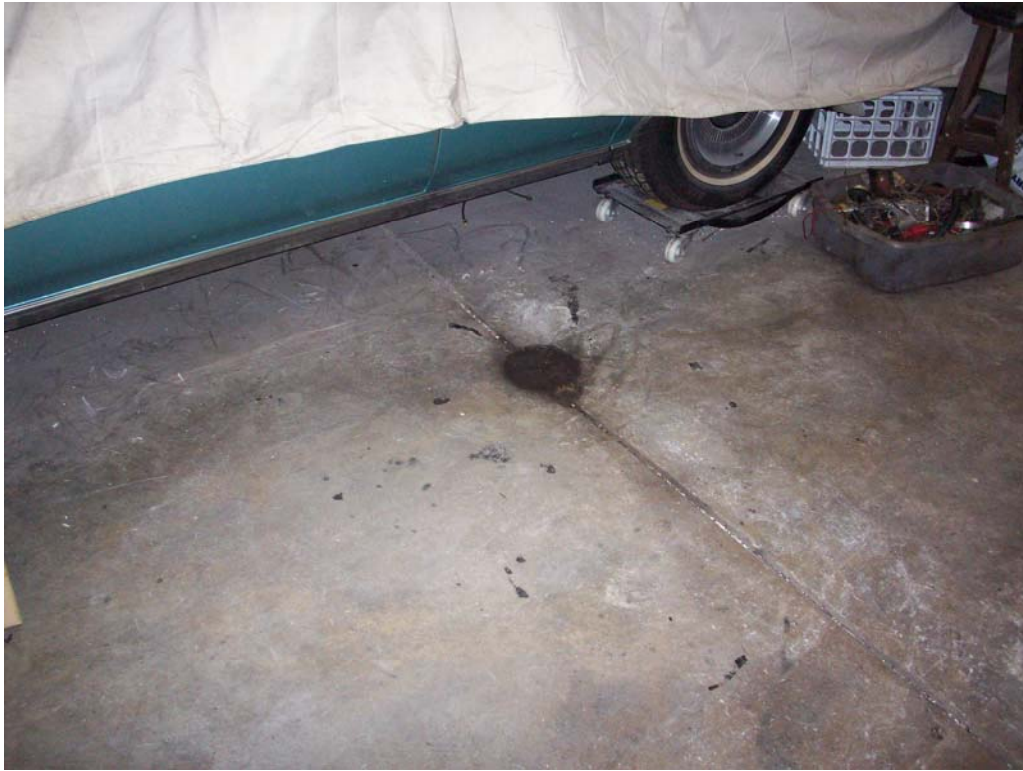
Floor drain at rear of garage area (east bay)
