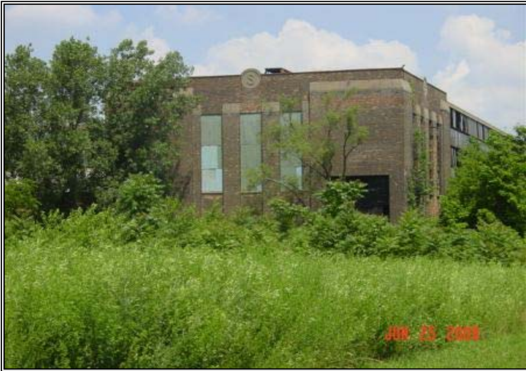
PHOTO 13: View looking north at the southeast corner of the Property.
