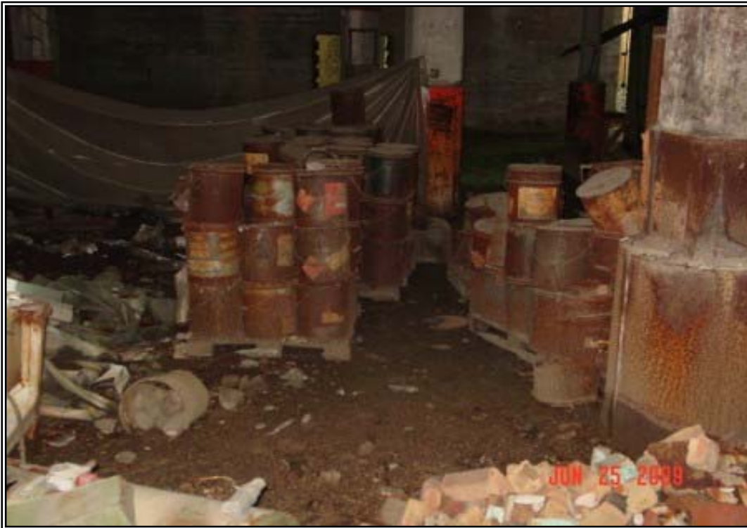
PHOTO 10: Five gallon pails palletized with flammable labels found under the foundry stacks.
