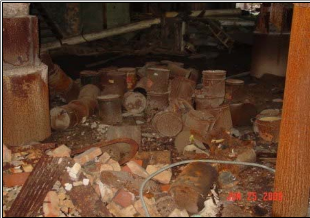
PHOTO 11: Five gallon pails piled under the foundry stacks.
