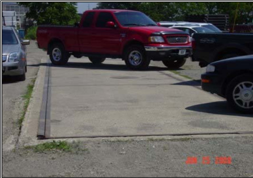
PHOTO 5: Unknown concrete form with steel framing in the ground.
