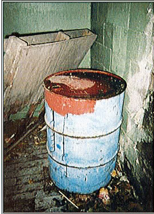
PHOTO 19: A 55-gallon drum labeled 'kerosene' observed in the closet area of the rail yard house. Note that the drum is uncapped.
