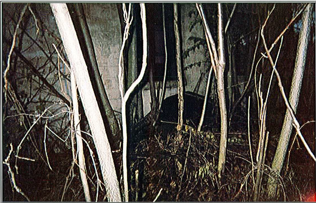
PHOTO 20: West side of the rail yard house, showing an approximately 150-gallon steel AST leaning against the side of the building.
