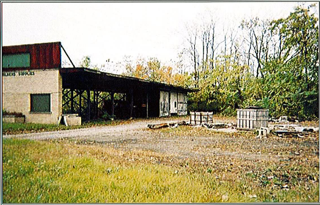
PHOTO 1: North facing side of the open-air lumber storage building on the Eckler-Lahey property.
