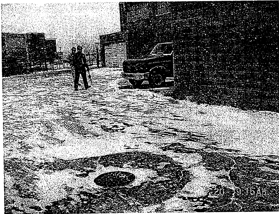
26. VIEW OF A DRY WELL LOCATED EAST OF THE HUCKINS TOOL & DIE BUILDING.
