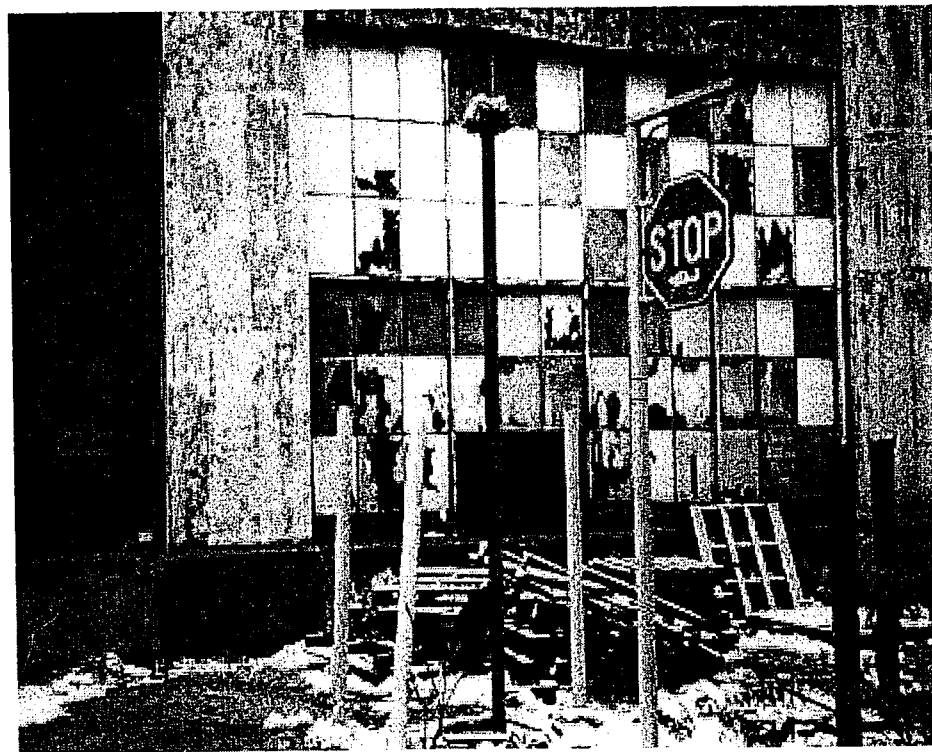
16. VIEW OF A VENT PIPE LOCATED SOUTH OF BUILDING 78.
