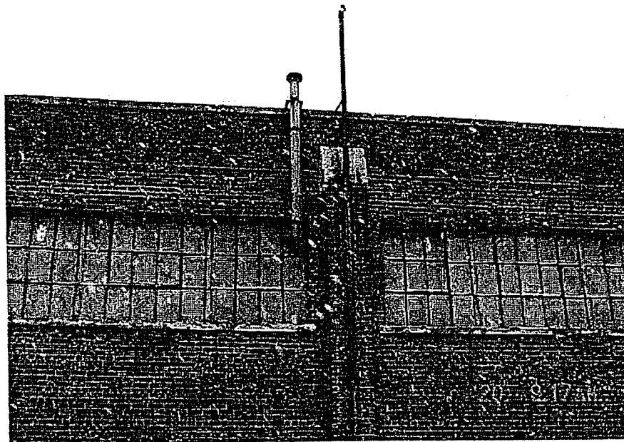
24. VIEW OF A VENT PIPE ASSOCIATED WITH A 5,000-GALLON UST LOCATED EAST OF THE HUCKINS TOOL & DIE BUILDING.
