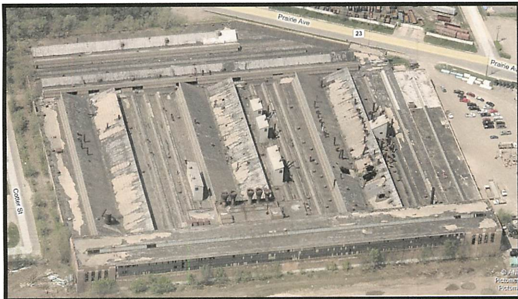
View of Building From East, Looking West
