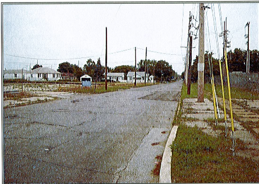
PHOTO 28: Godland Avenue followed by an empty lot and residences borders the Site to the west.
