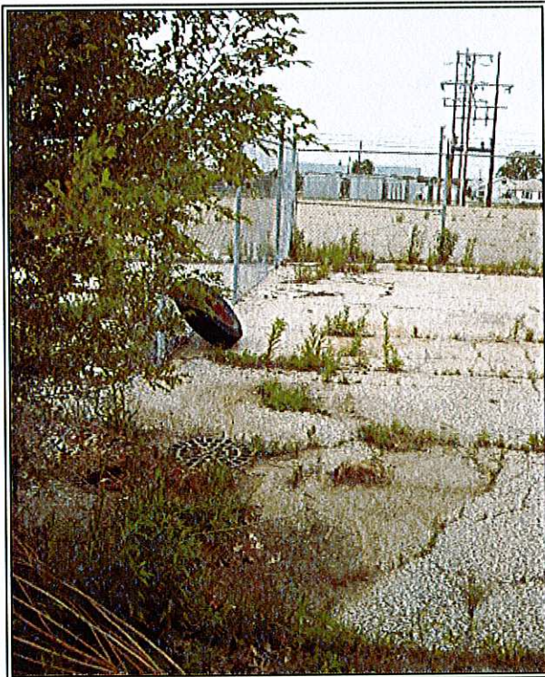
PHOTO 20: Drain on southern portion of main building lot.
