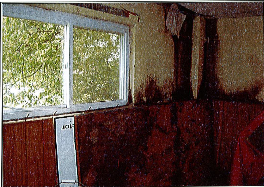
PHOTO 6: Additional view of walls in southern portion of the building.
