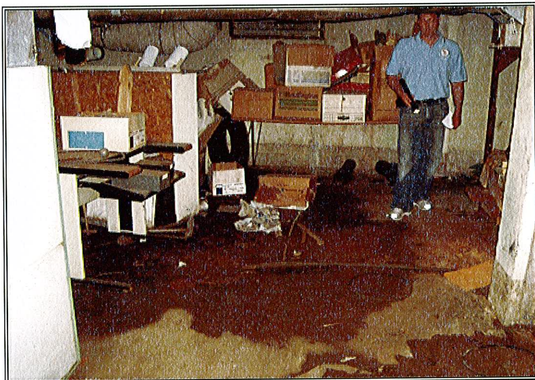
PHOTO 12: Floor in basement damp from flooding through drains.
