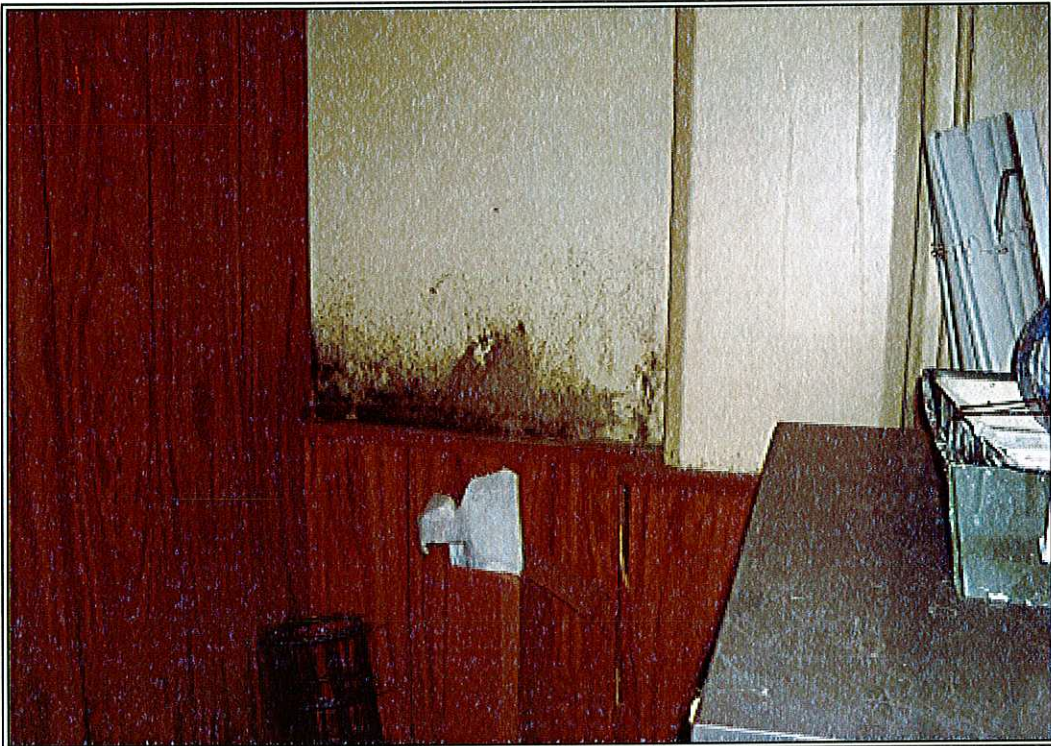
PHOTO 5: View of walls in southern portion of the main building.
