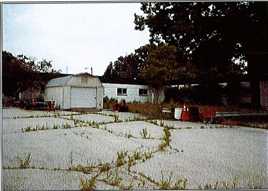
PHOTO 19: Storage shed located on the southern portion of the main building lot.
