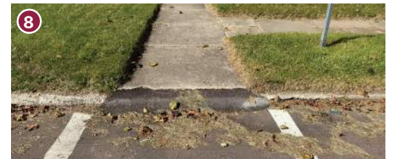
8 Missing or out of compliant ADA ramps
