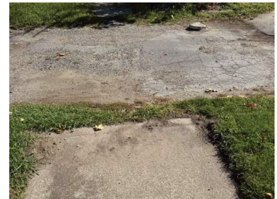
Deteriorated Driveway at Sidewalk Crossing
