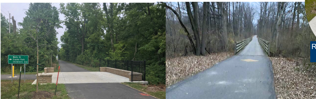
Pufferbelly Trail | Fort Wayne, IN | Inspection & design of 1.6 miles of 12' wide shared-use asphalt trail along former rail corridor. Extensive inspector/supervisor coordination to include amenities such as benches and a spur to connect to Franke Park along with refurbishing pedestrian bridge.
