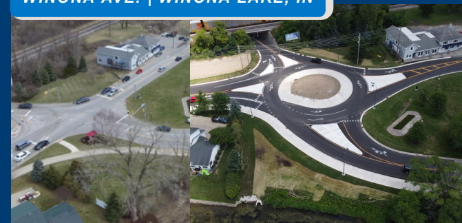
Before and After: Multi-leg roundabout and trail design, improving safety, traffic flow, and pedestrian connectivity. The project required complex drainage design, utility coordination, and constructability planning—skills directly applicable to the Ewing Avenue intersection and trail corridor.
