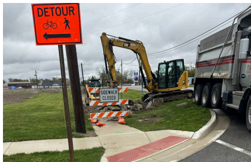
Woodburn Trail & Sidewalk | Woodburn, IN | Inspection & design of 10' wide HMA trail, sidewalks, curb ramps, crosswalks, and storm sewer improvements.
