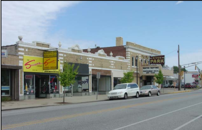
Photo 4: Colonial Gardens (2900) Block – An example of well-maintained, connected commercial units
