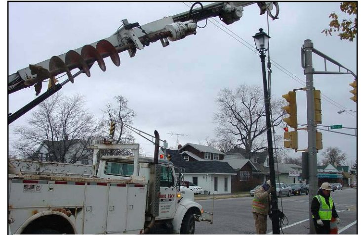
Photo 3: Installation of Decorative Lighting at 26th Street
