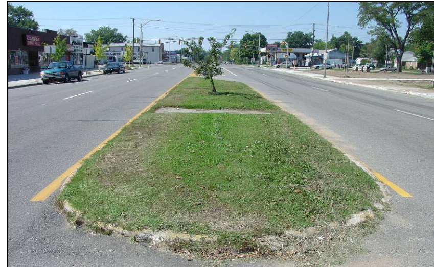
Photo 17: Existing median between Ironwood Dr. and Twyckenham Dr.
