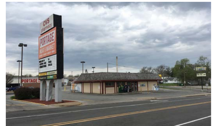
Existing condition of entry into retail plaza from Portage Ave.
