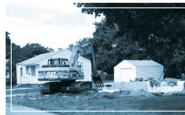
Demolition of dilapidated house in a South Bend neighborhood.
