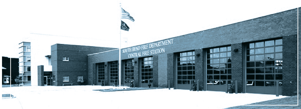
New Central Fire Station on Michigan Street just south of downtown.
