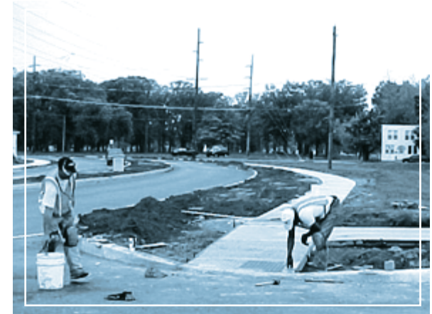
Construction crew installing new sidewalks.
