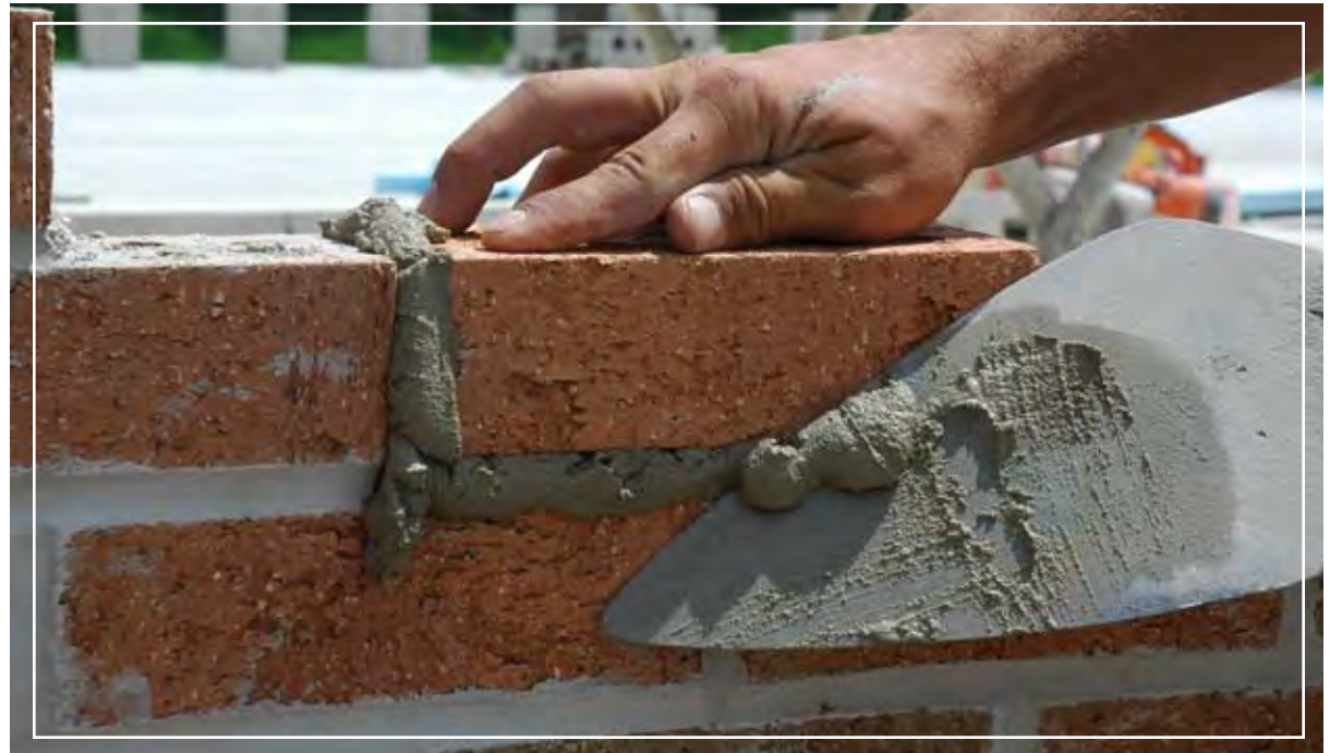
Project Implementation: A mason laying bricks on a construction site.
