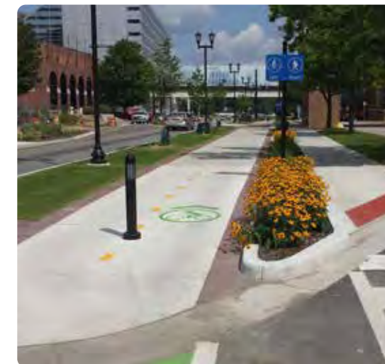
Protected Bike Lane Facility separated from motor vehicle traffic by a curb, planter, or other physical barriers for the exclusive use of people on bicycles
