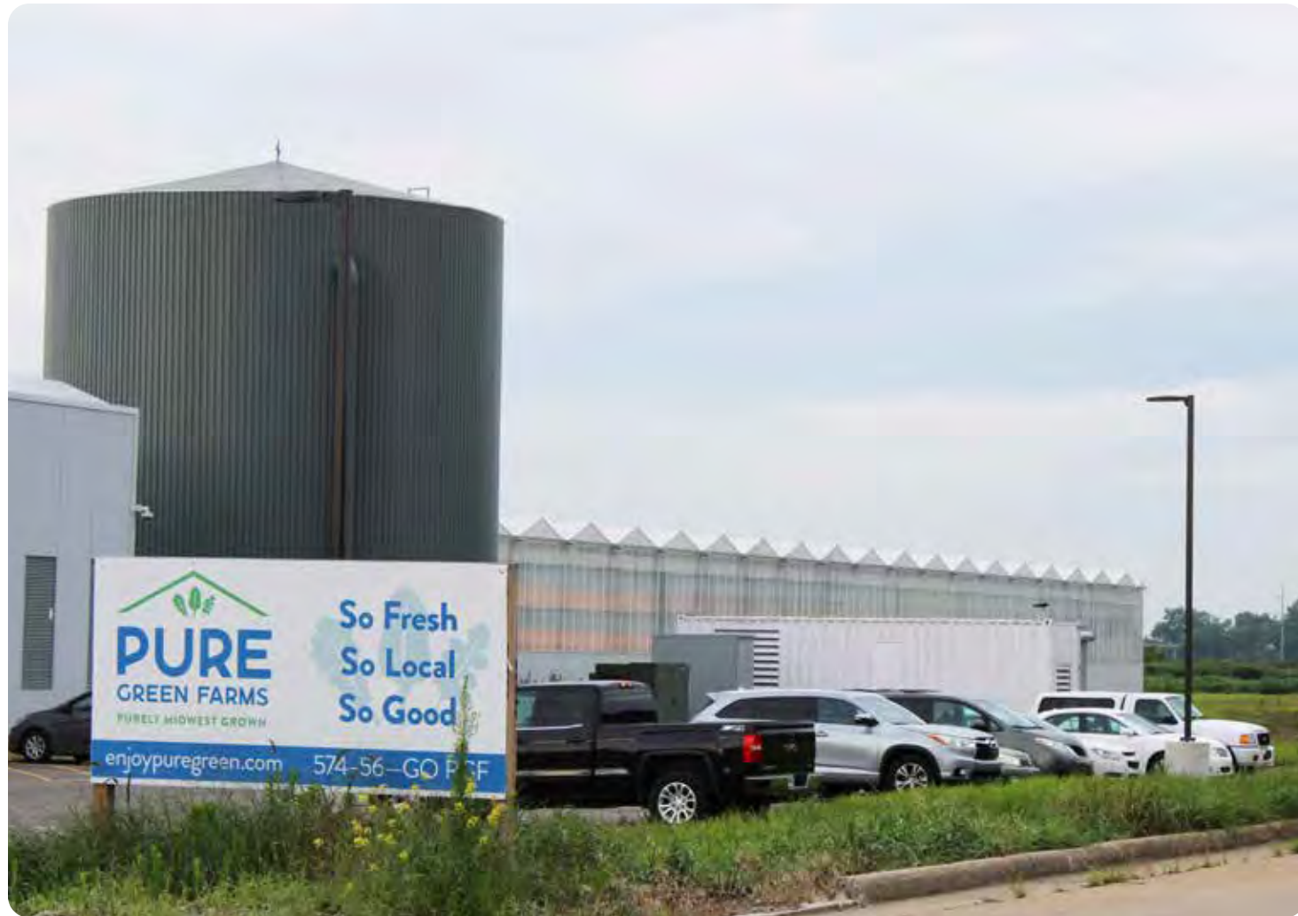
Pure Green greenhouse building.
