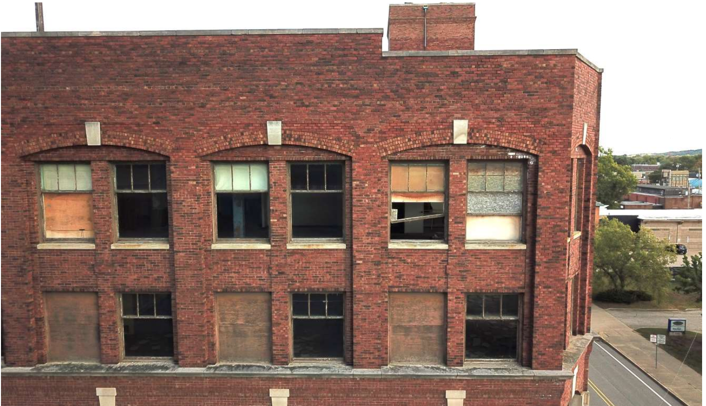
Photo 11 - Typical Condition 3-4 Floors - W Facade
