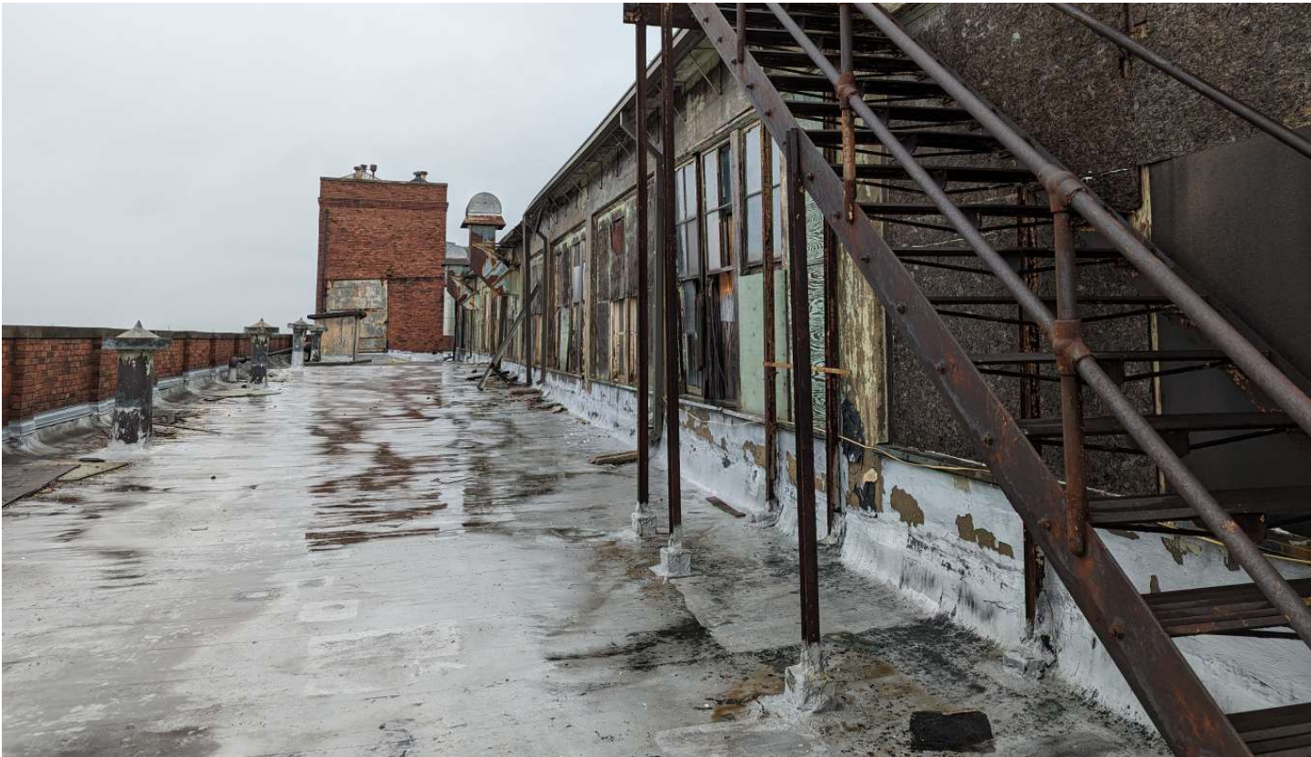
Photo 21 - View to W of Clerestory Windows and Roof
