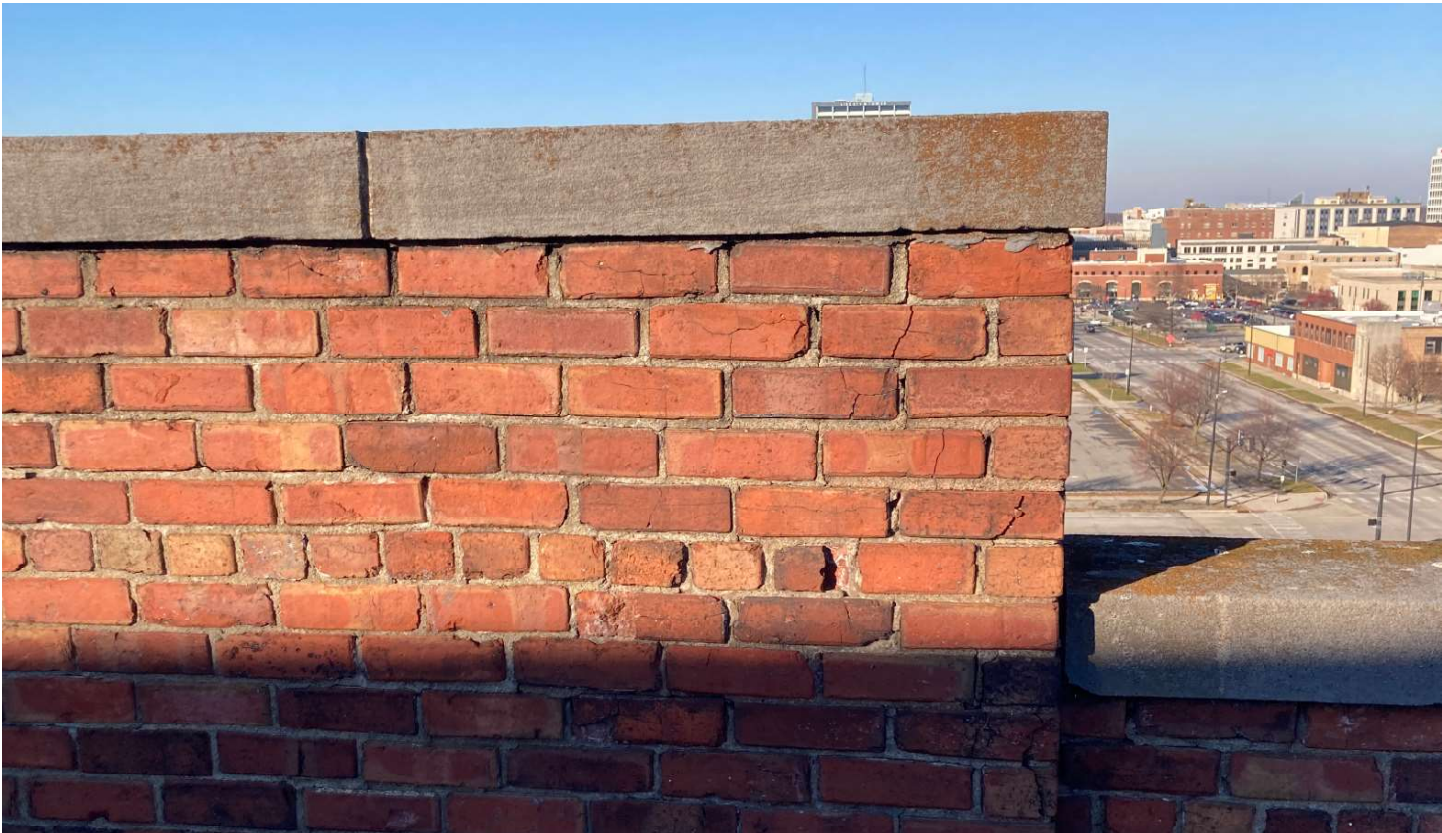
Photo 27 - Typical Step in Height of Parapet Wall
