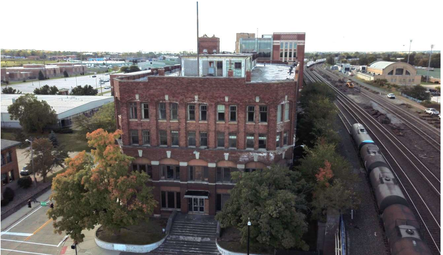
Photo 5 - Aerial from East
