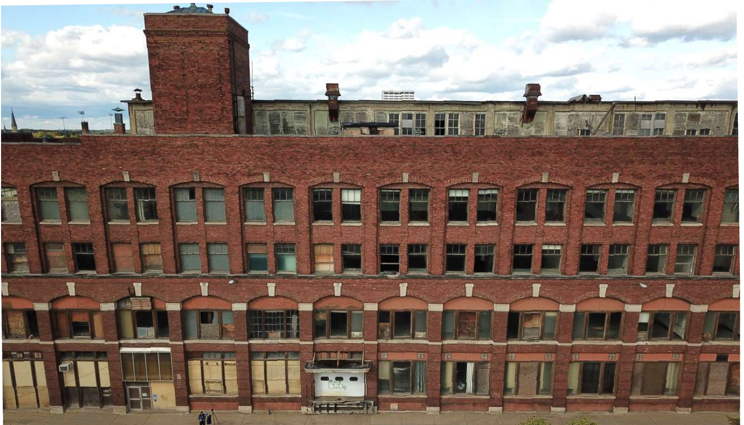
Photo 9 - South Central Facade
