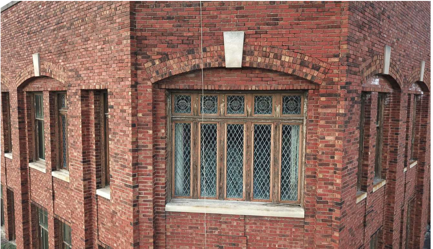
Photo 7 - Executive Office Windows at SE Corner
