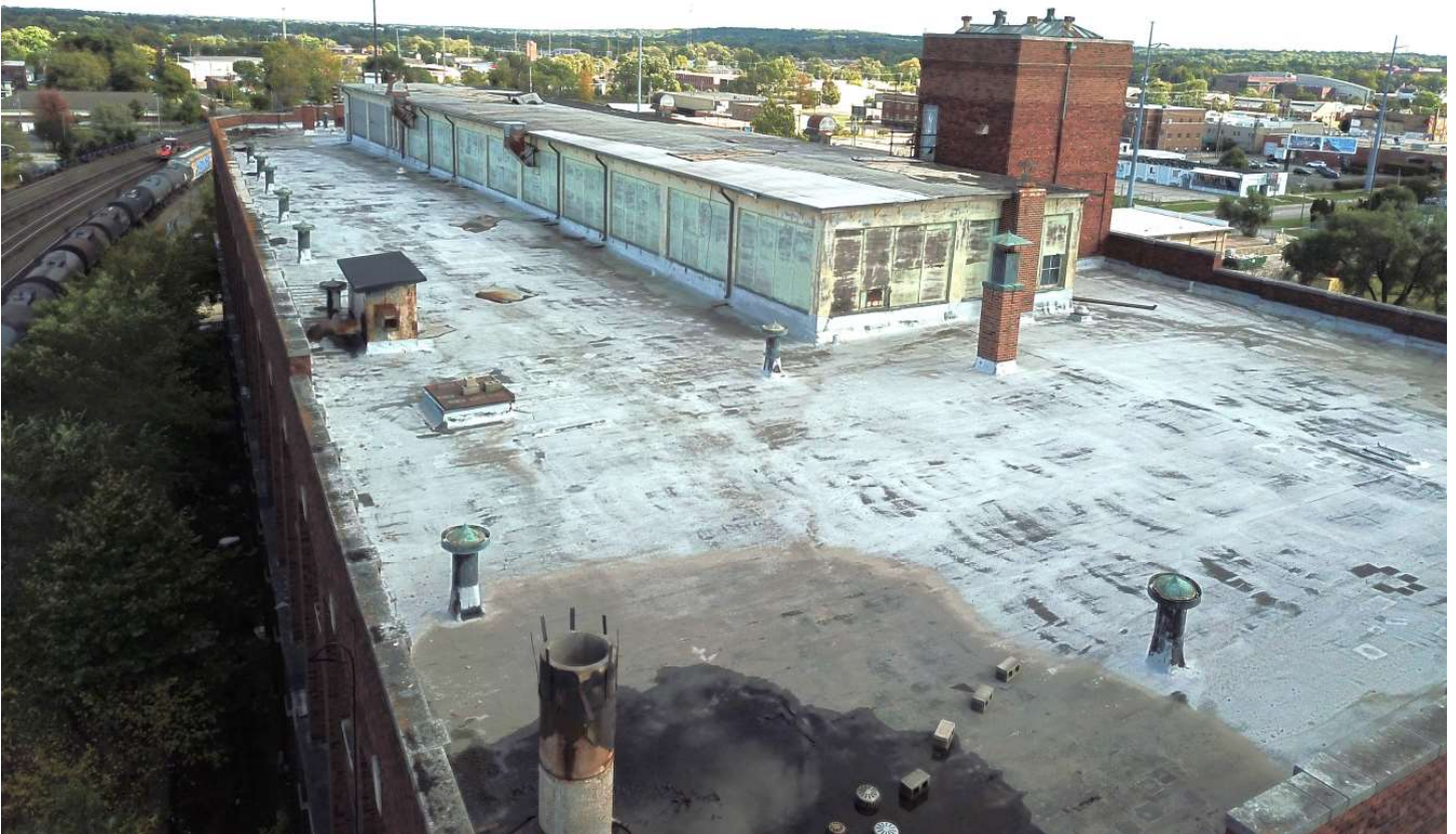
Photo 13 - Monitor Roof w/ Clerestory from NW
