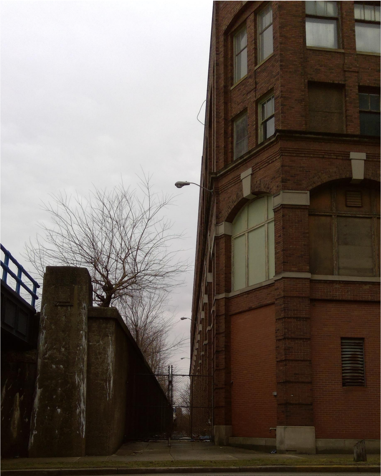
Picture of the East side of building March 2000
