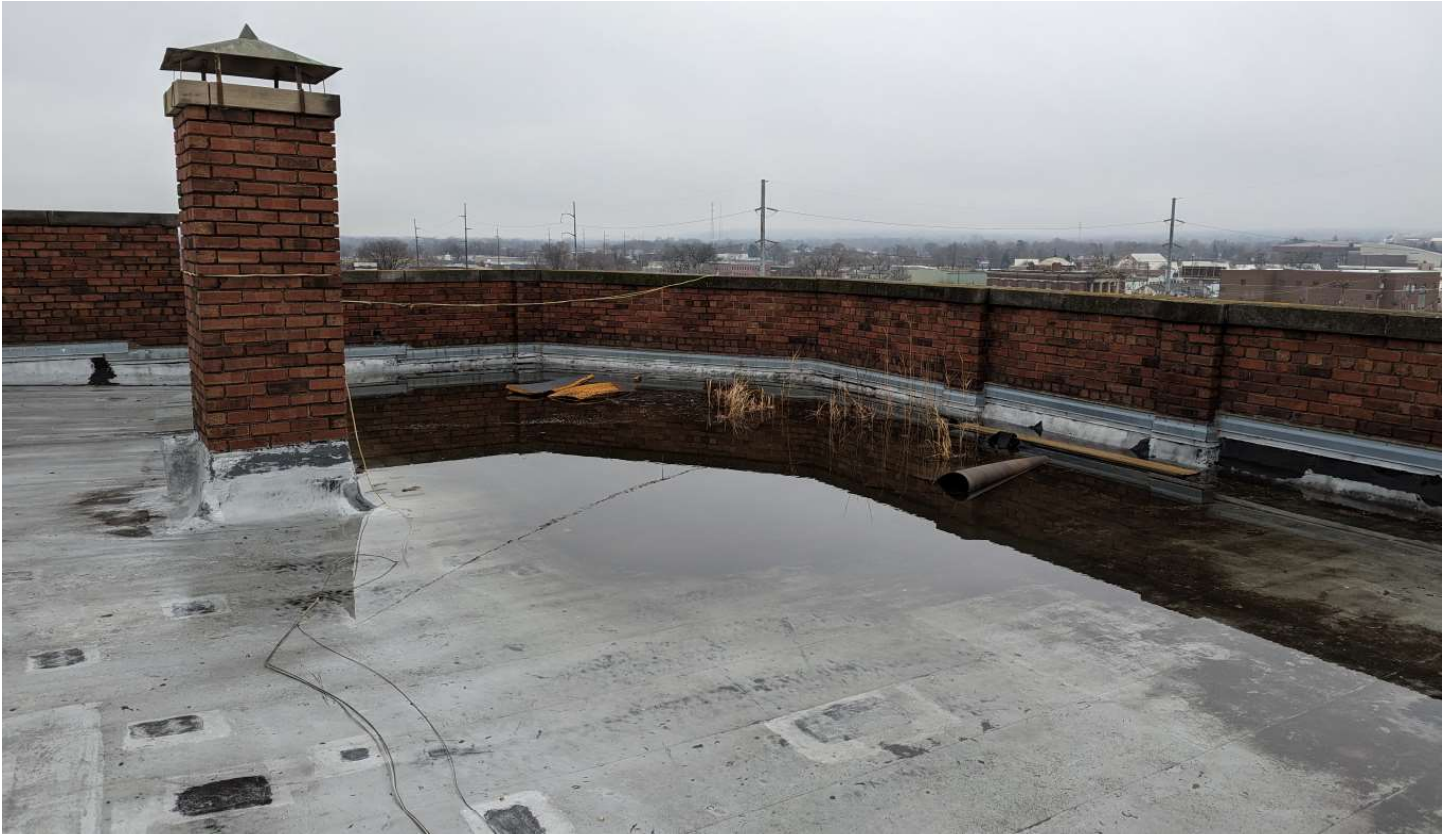
Photo 22 - Significant Ponding above Executive Offices
