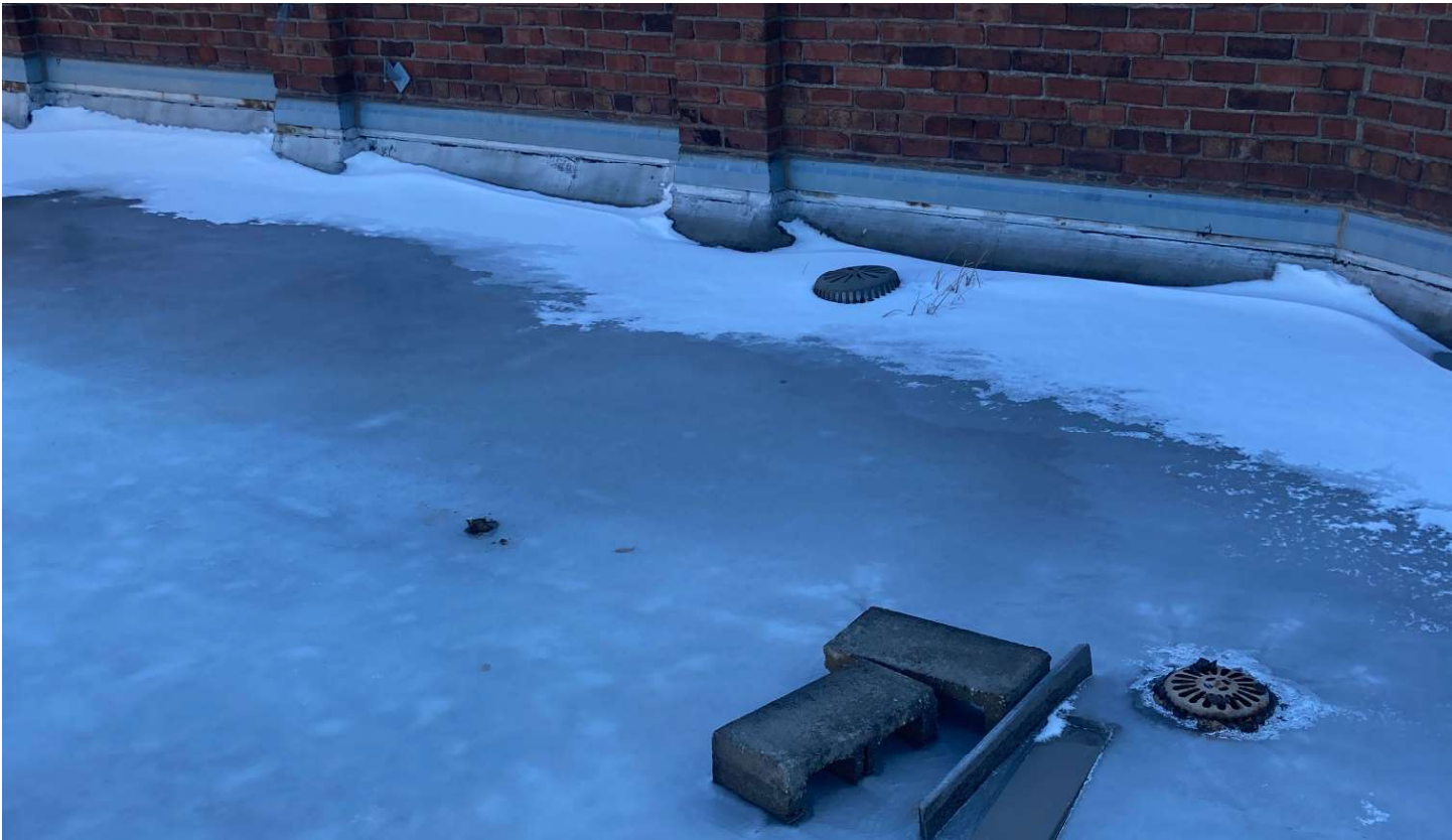
Photo 28 - Ponding at Corner Drain
