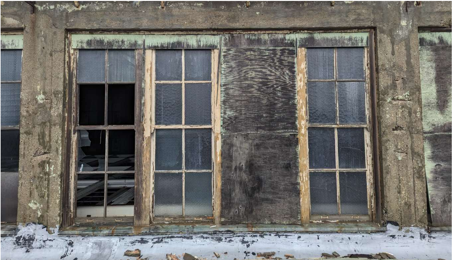
Photo 19 - Typical Bank of Clerestory Double Hung Windows
