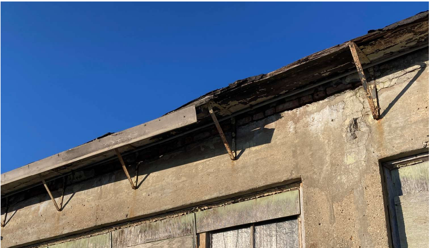
Photo 20 - Brackets, Flashing, etc. at Monitor Roof
