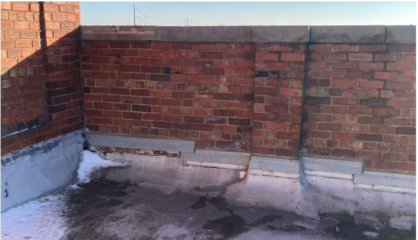
Photo 24 - Typical Stepped Flashing and Parapet Pier adjacent to Elevator Tower
