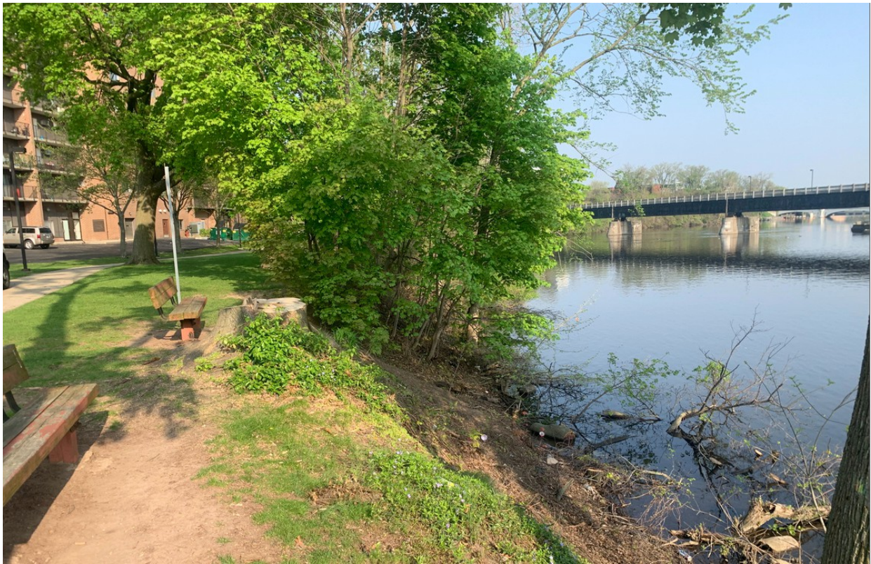
Eroding shoreline at Plaza Park as seen on May 14, 2022
