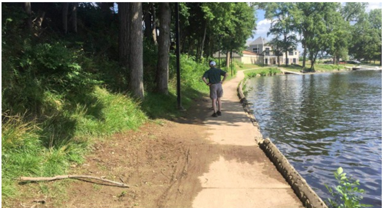
Garry Harrington and Andrew Tucker survey erosion and hillside destabilization at Gov. Joe Kernan Park
