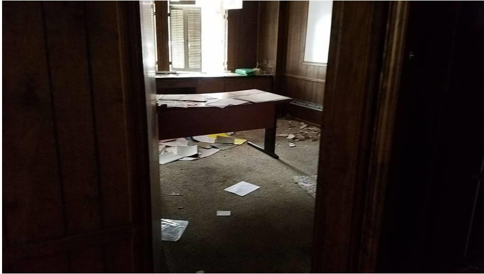
CLIENT NAME: City of South Bend & South Bend Brownfields Coalition DATE: December 14, 2017 LOCATION: Lafayette Building, 115 South Lafayette Boulevard in South Bend, Indiana SUBJECT: General view of vacant former office space in site building PHOTOGRAPHER: Nivas R. Vijay (Heartland) PHOTO: 5
