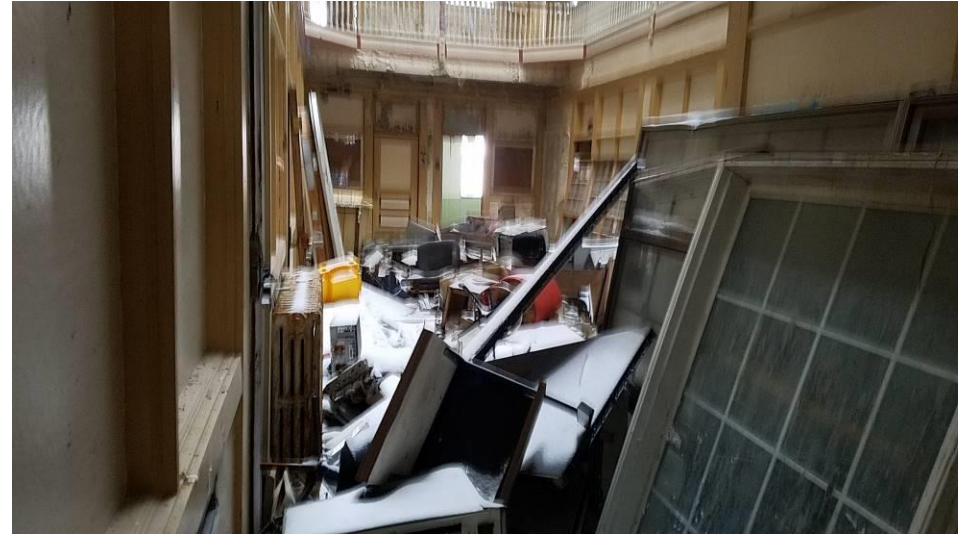
CLIENT NAME: City of South Bend & South Bend Brownfields Coalition DATE: December 14, 2017 LOCATION: Lafayette Building, 115 South Lafayette Boulevard in South Bend, Indiana SUBJECT: Close up view of strewn refuse and debris and entry way area of site building PHOTOGRAPHER: Nivas R. Vijay (Heartland) PHOTO: 4
