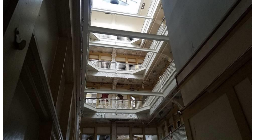
CLIENT NAME: City of South Bend & South Bend Brownfields Coalition DATE: December 14, 2017 LOCATION: Lafayette Building, 115 South Lafayette Boulevard in South Bend, Indiana SUBJECT: View looking up at floors of site building from entry way PHOTOGRAPHER: Nivas R. Vijay (Heartland) PHOTO: 6
