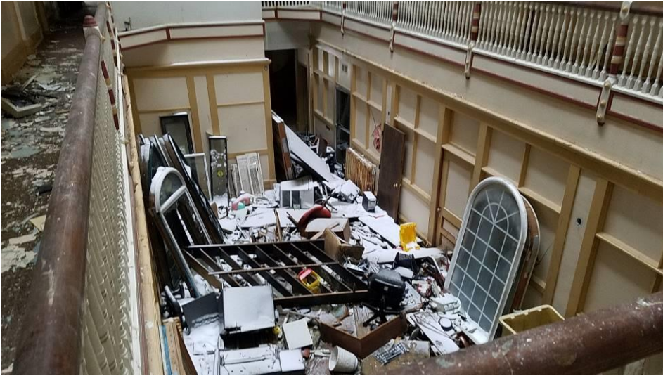
CLIENT NAME: City of South Bend & South Bend Brownfields Coalition DATE: December 14, 2017 LOCATION: Lafayette Building, 115 South Lafayette Boulevard in South Bend, Indiana SUBJECT: View entryway of site building, looking down from second floor walkway PHOTOGRAPHER: Nivas R. Vijay (Heartland) PHOTO: 3
