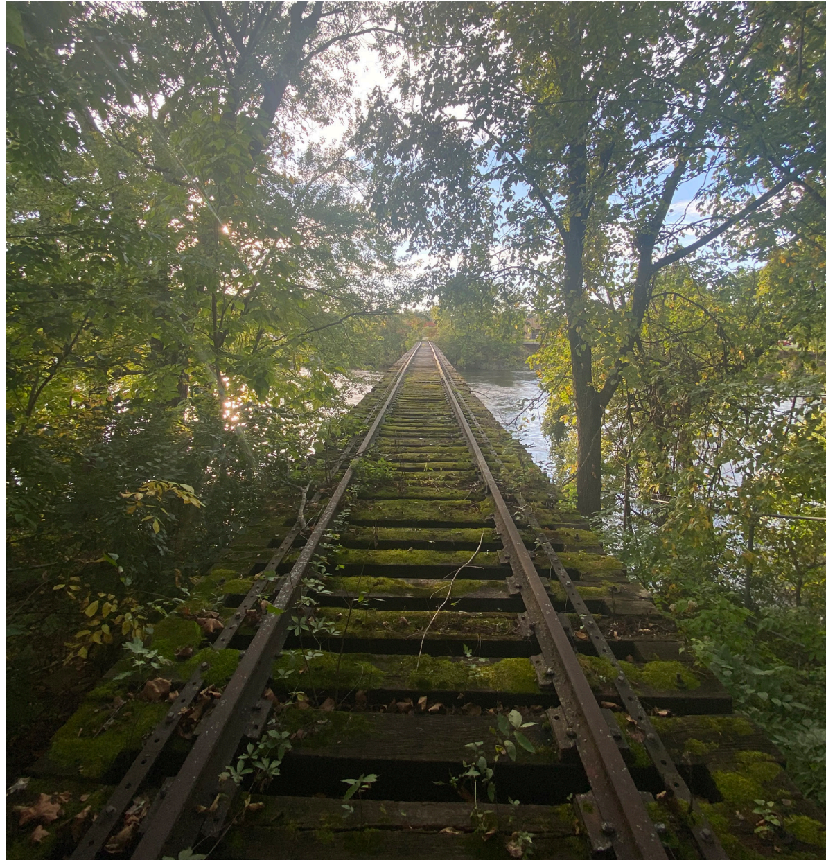
Existing Railroad Bridge Looking West
