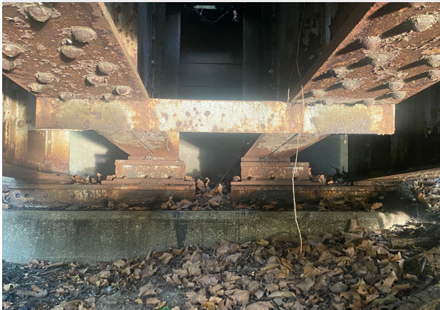
Existing Bridge Bearings
