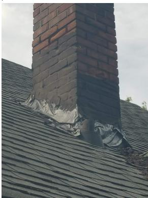
2. 8x14 section of roof -water damaged and rotting away from the wall of the house in the Northeast corner. Replacing the sub-roof, ice & water shield, asphalt shingles and wall flashing with like materials.
