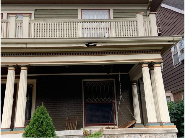
I enclose photos of the water damage for your review. We bought the house in spring 2018, and the gutters appeared not to have been cleaned for the four years the property was tenant occupied. We believe this led to water backup behind the fascia and resulted in the rot you see below:
