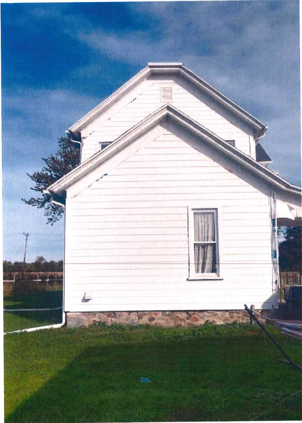
West face of house
