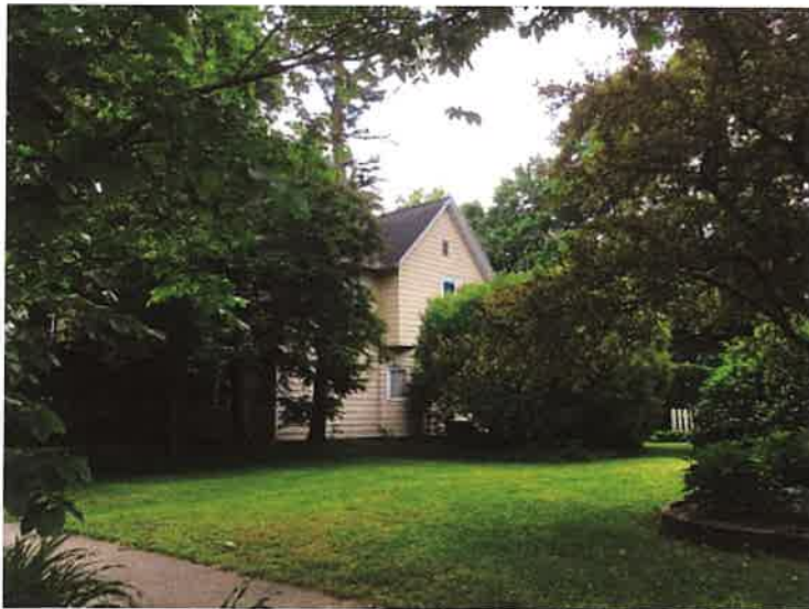
Figure 4. General view of the house from the street, looking east.
